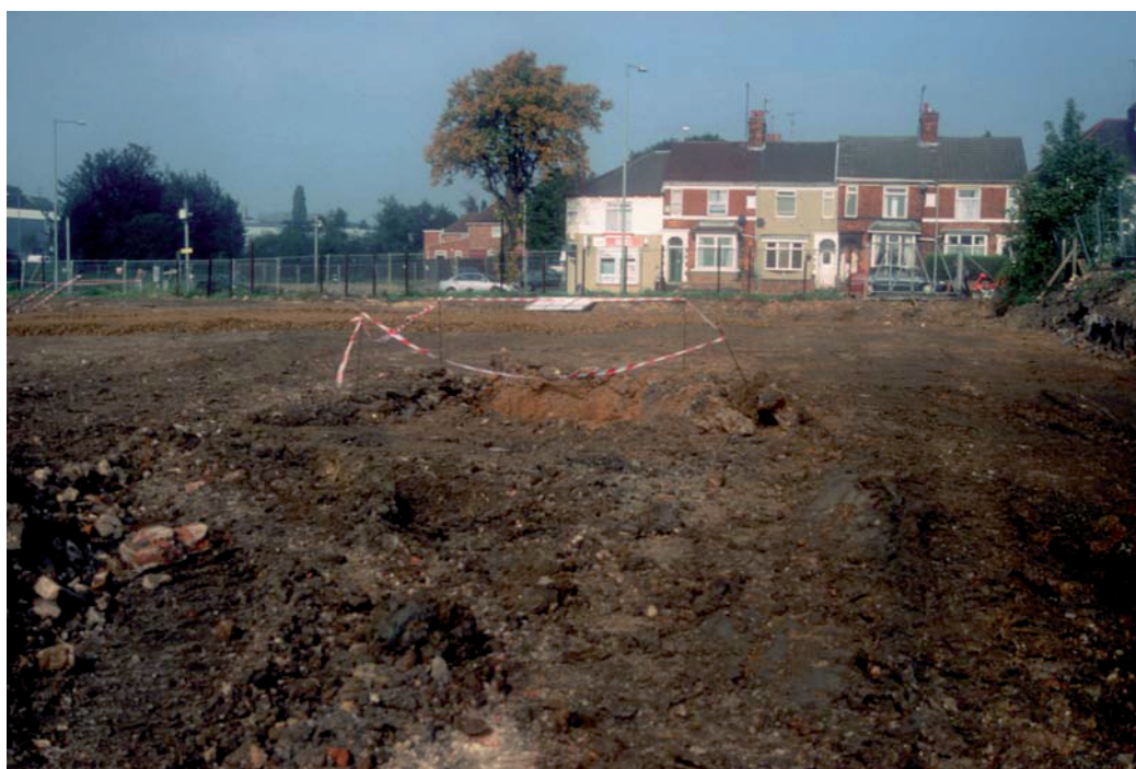
Plate 2: The development area during ground-works
