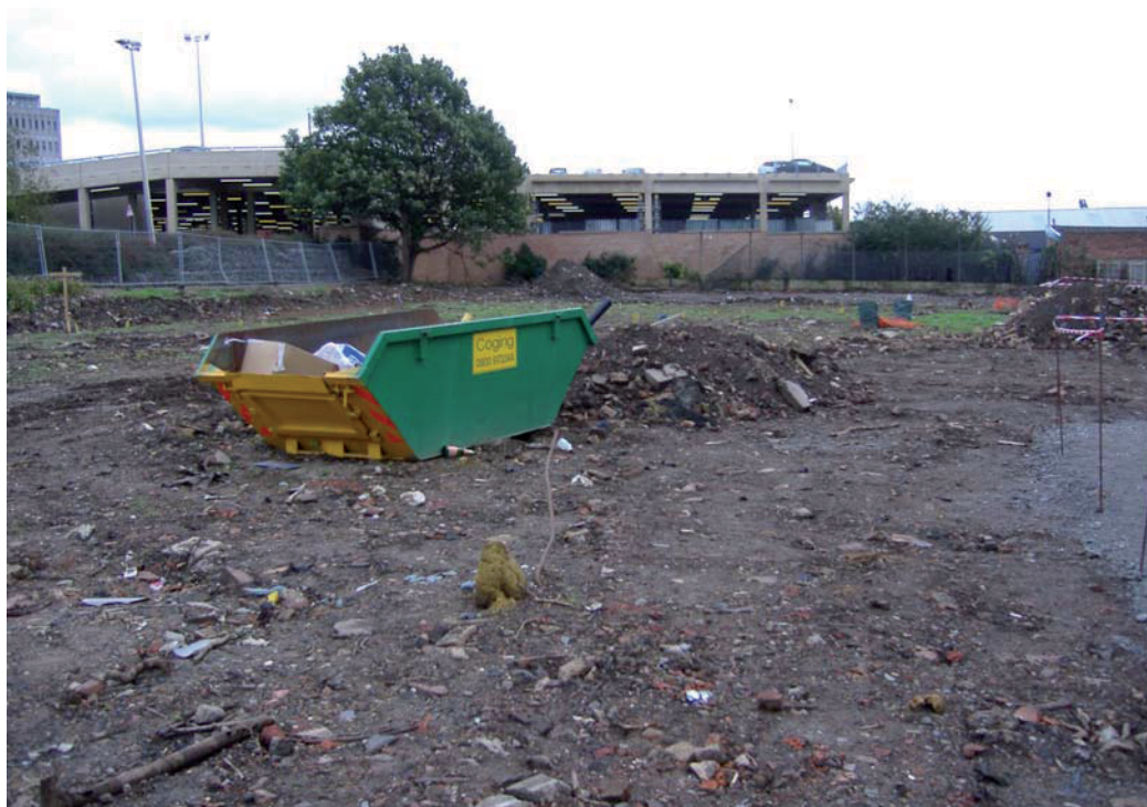
Plate 1: The area of development prior to the start of ground-works, viewed from the north
