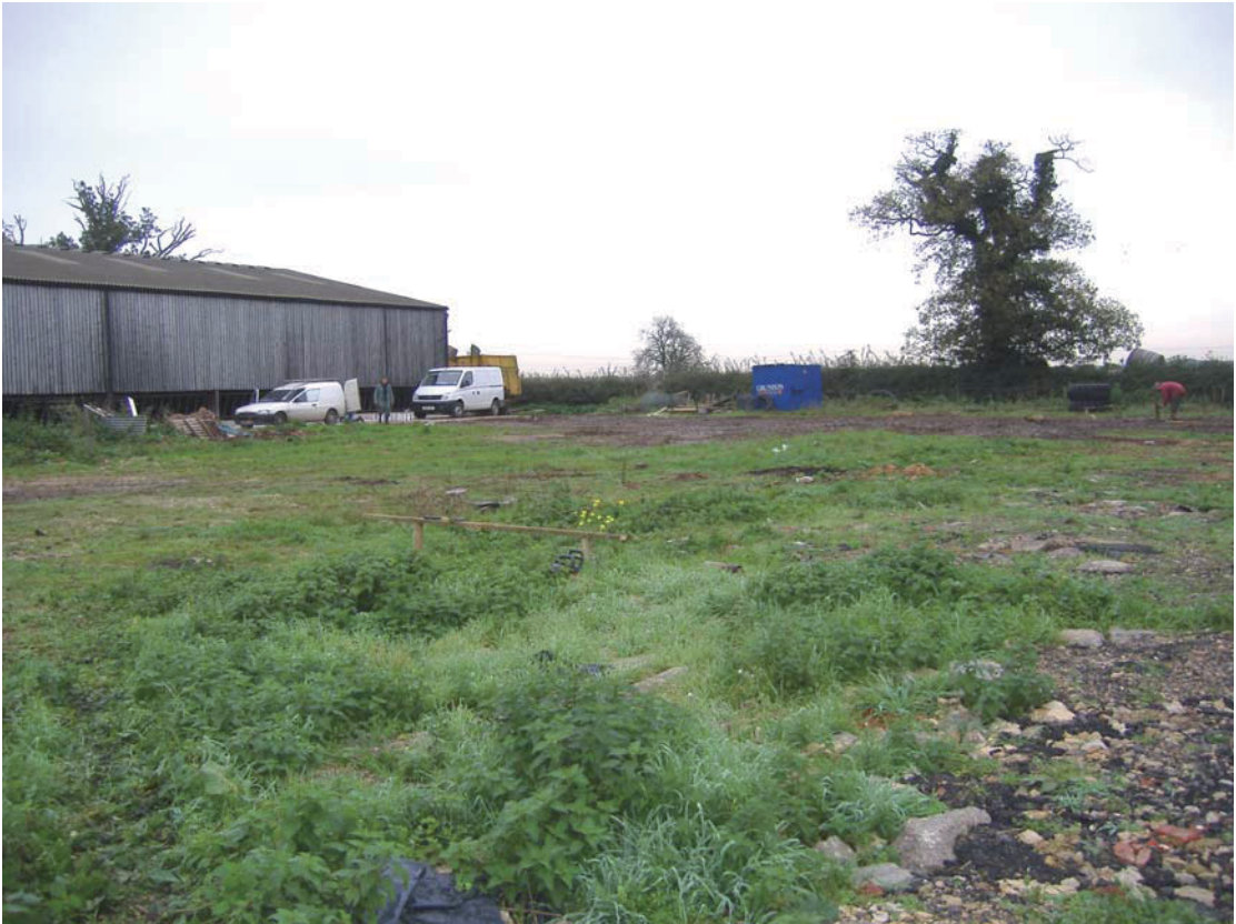
Plate 1: The development area at the start of groundworks
