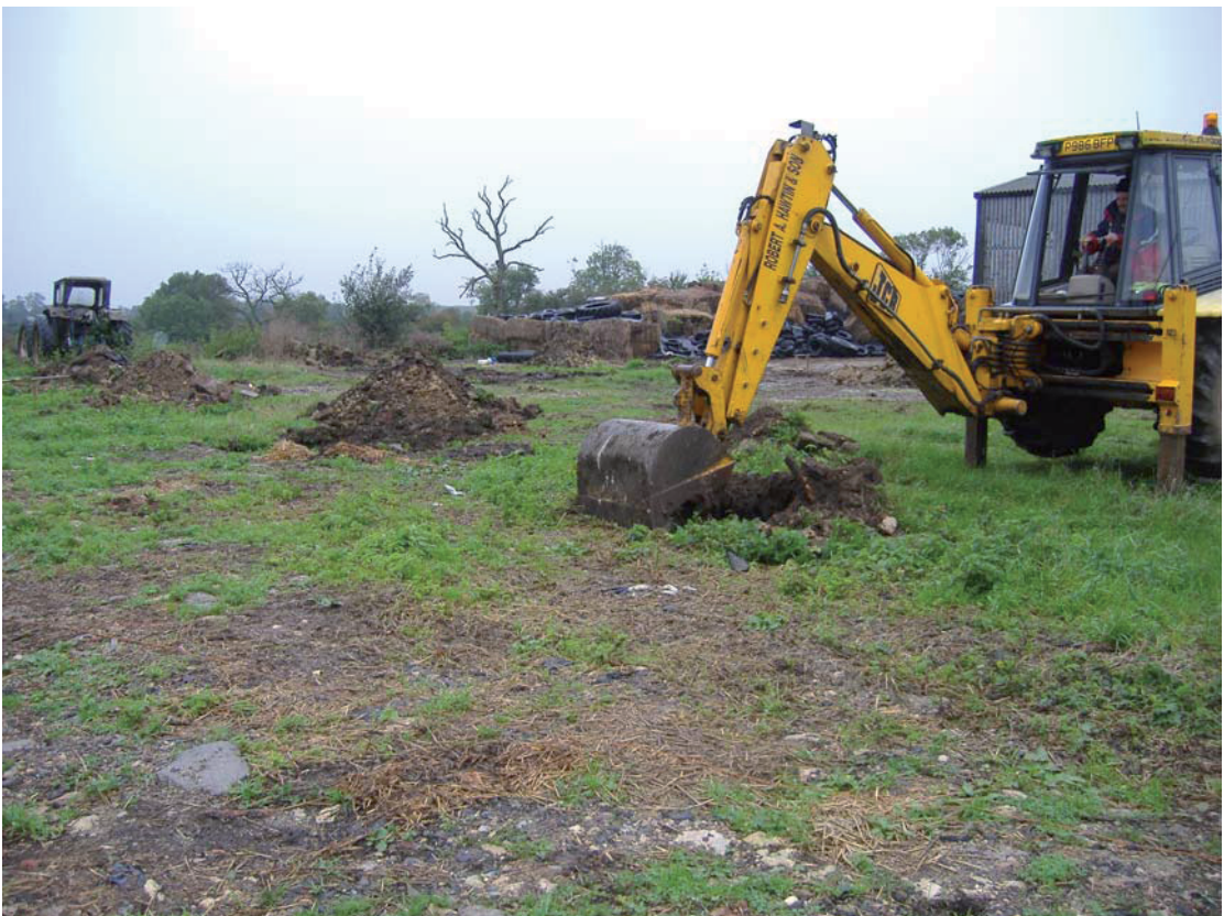
Plate 2: The excavation of the stanchion pits
