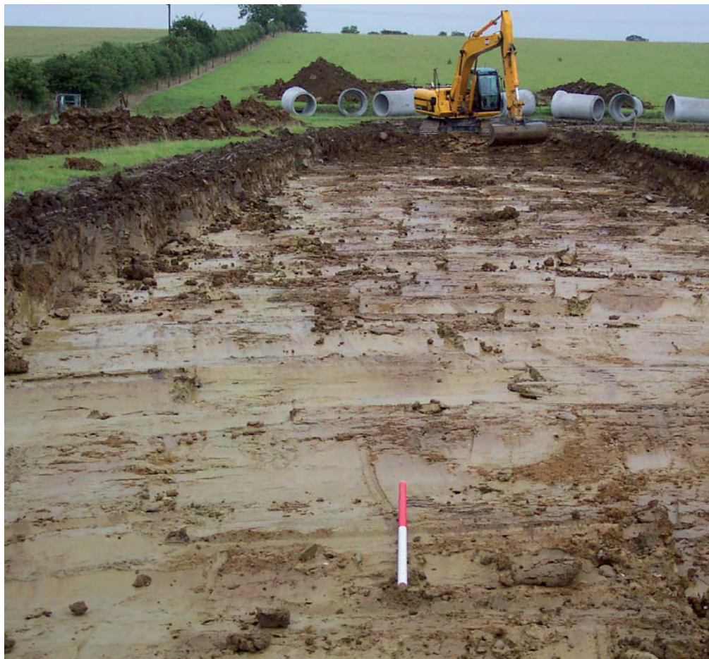
Plate 4: West Lake Wall Trench looking east
