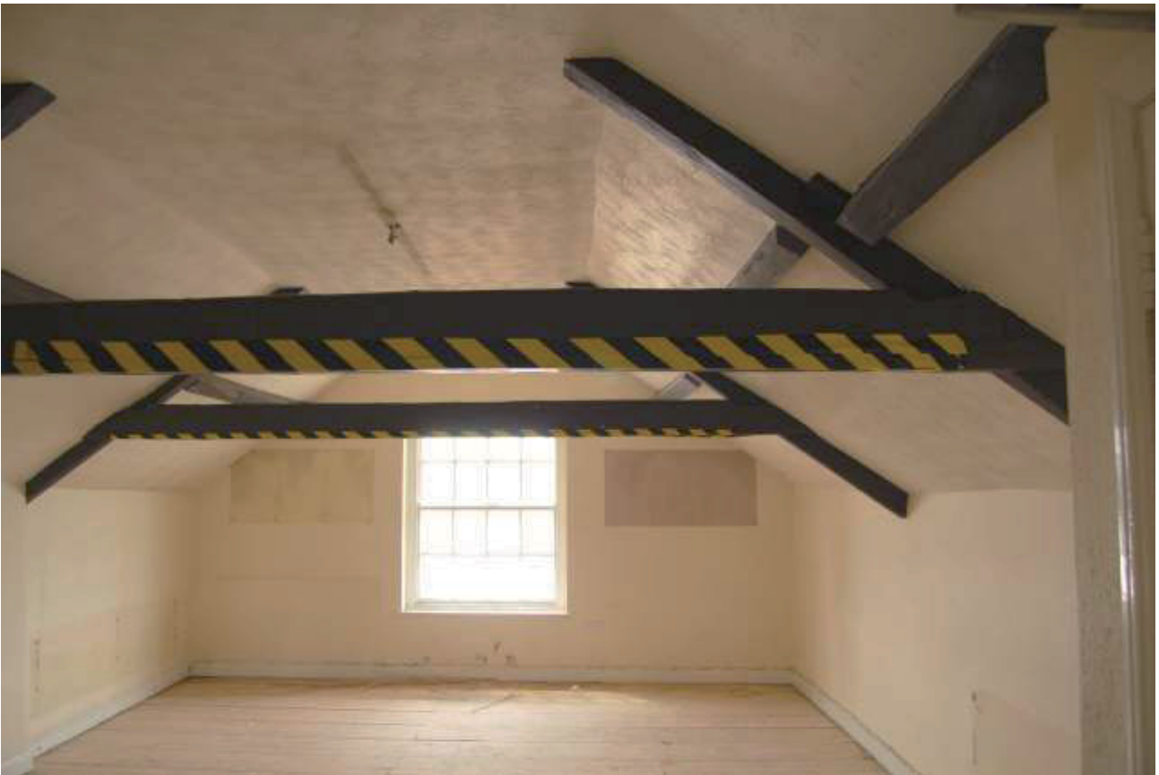
Plate 12: The exposed rafters and purlins in Room S1
