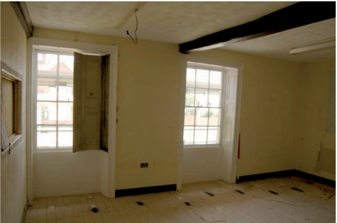
Plate 10: The sash windows and shutter boxes in Room F11
