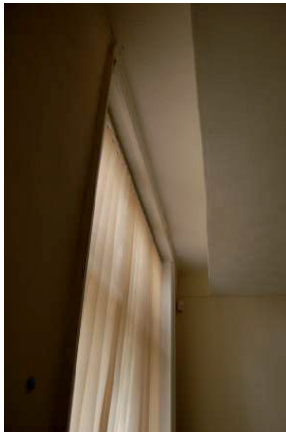
Plate 2: Lowered Ceiling Room G5
