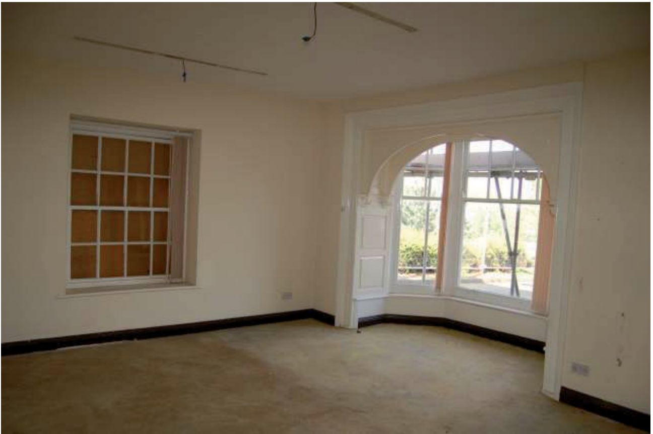
Plate 5: The arched timber pelmet in Room G21
