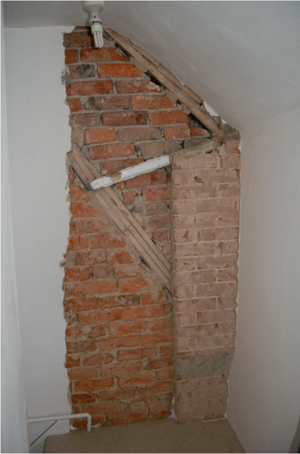
Plate 6 Dividing wall between cottages; first floor, east side (No 18) looking west
