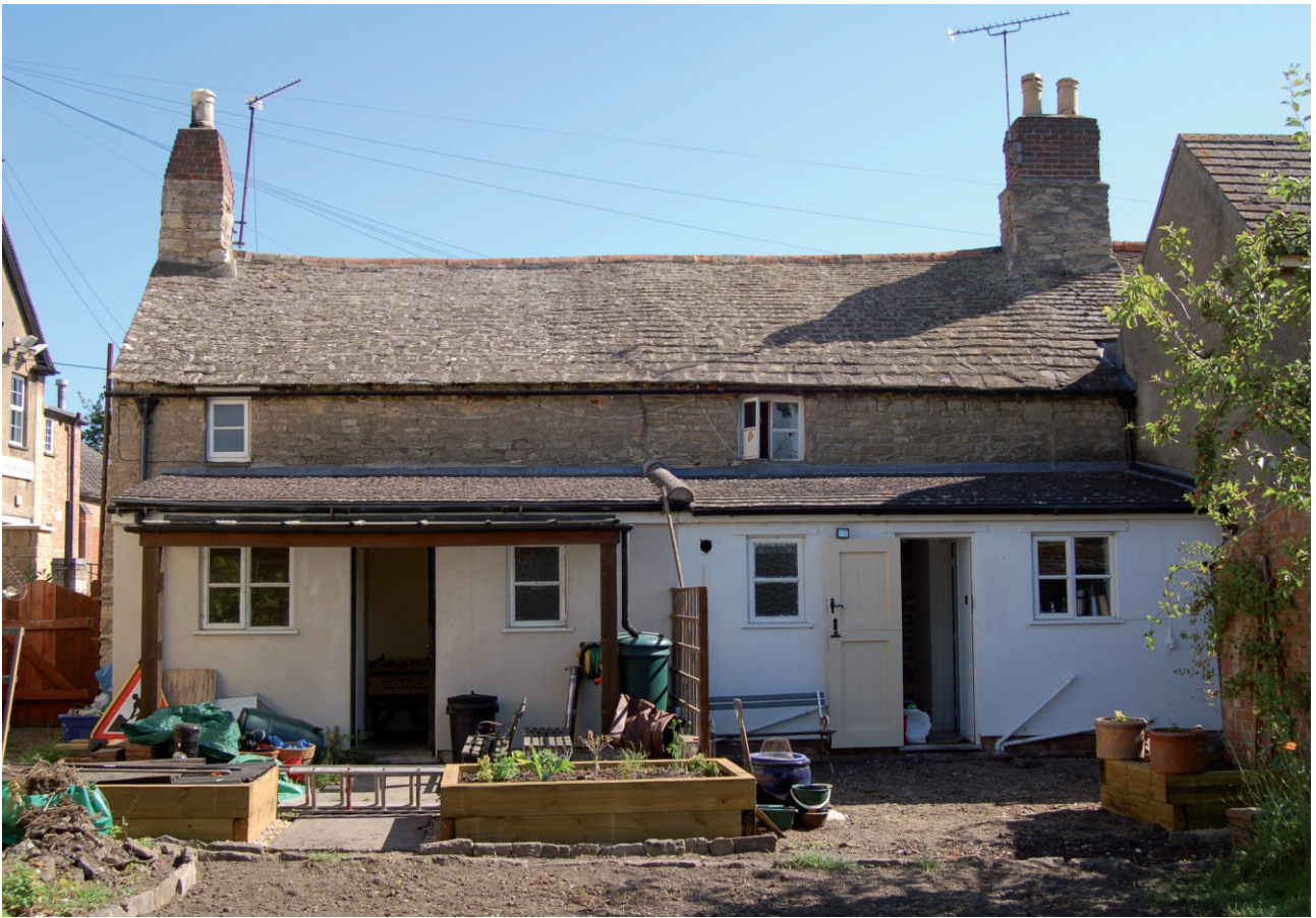
Plate 3 Garden frontage (south side) with later single storey additions
