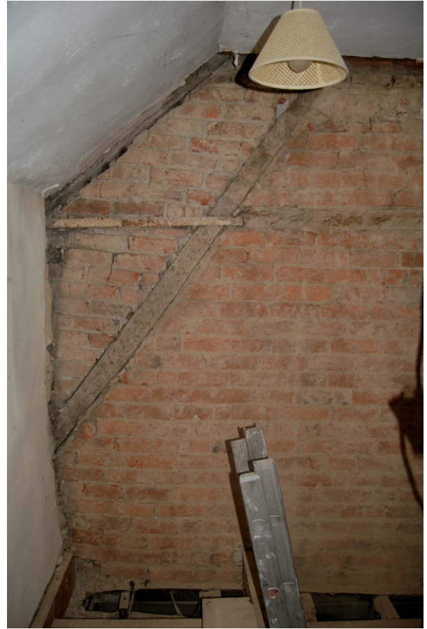
Plate 7 Dividing wall between cottages; first floor, west side (No 20) looking east
