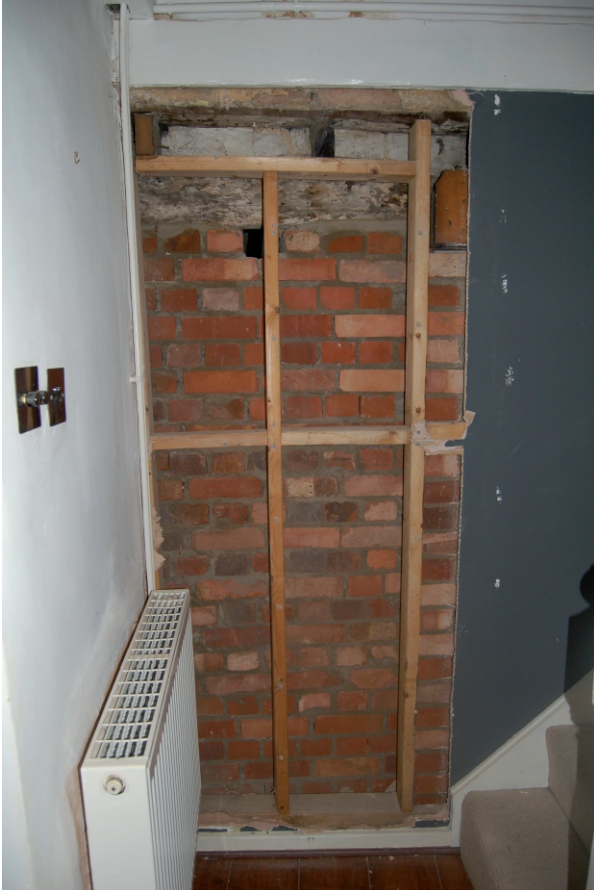
Plate 4 Dividing wall between cottages; ground floor, east side (No 18) looking west
