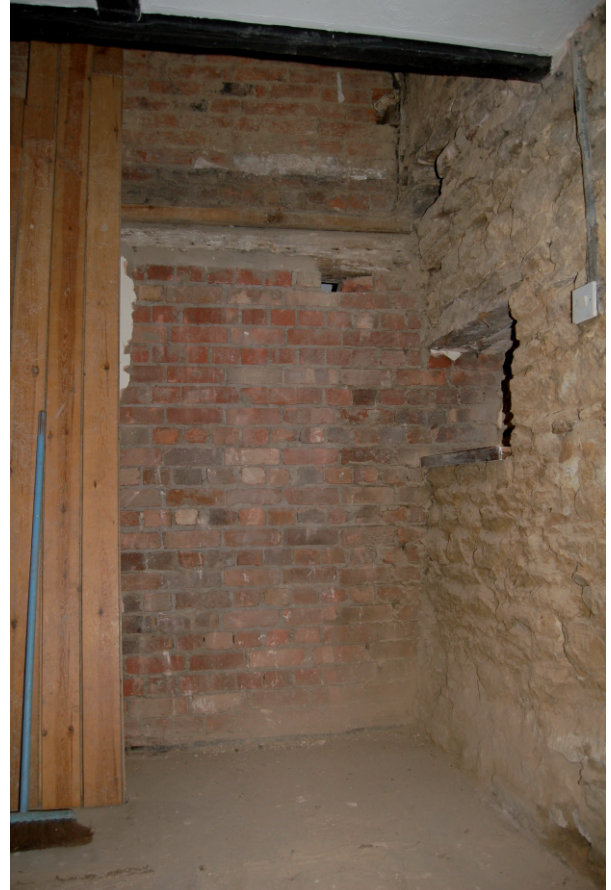
Plate 5 Dividing wall between cottages; ground floor, west side (No 20) looking east
