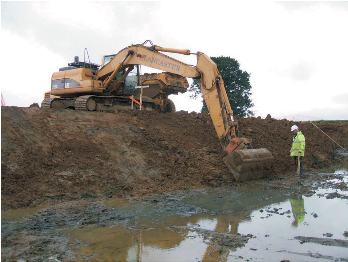
Plate 5: Machining of new river channel.
