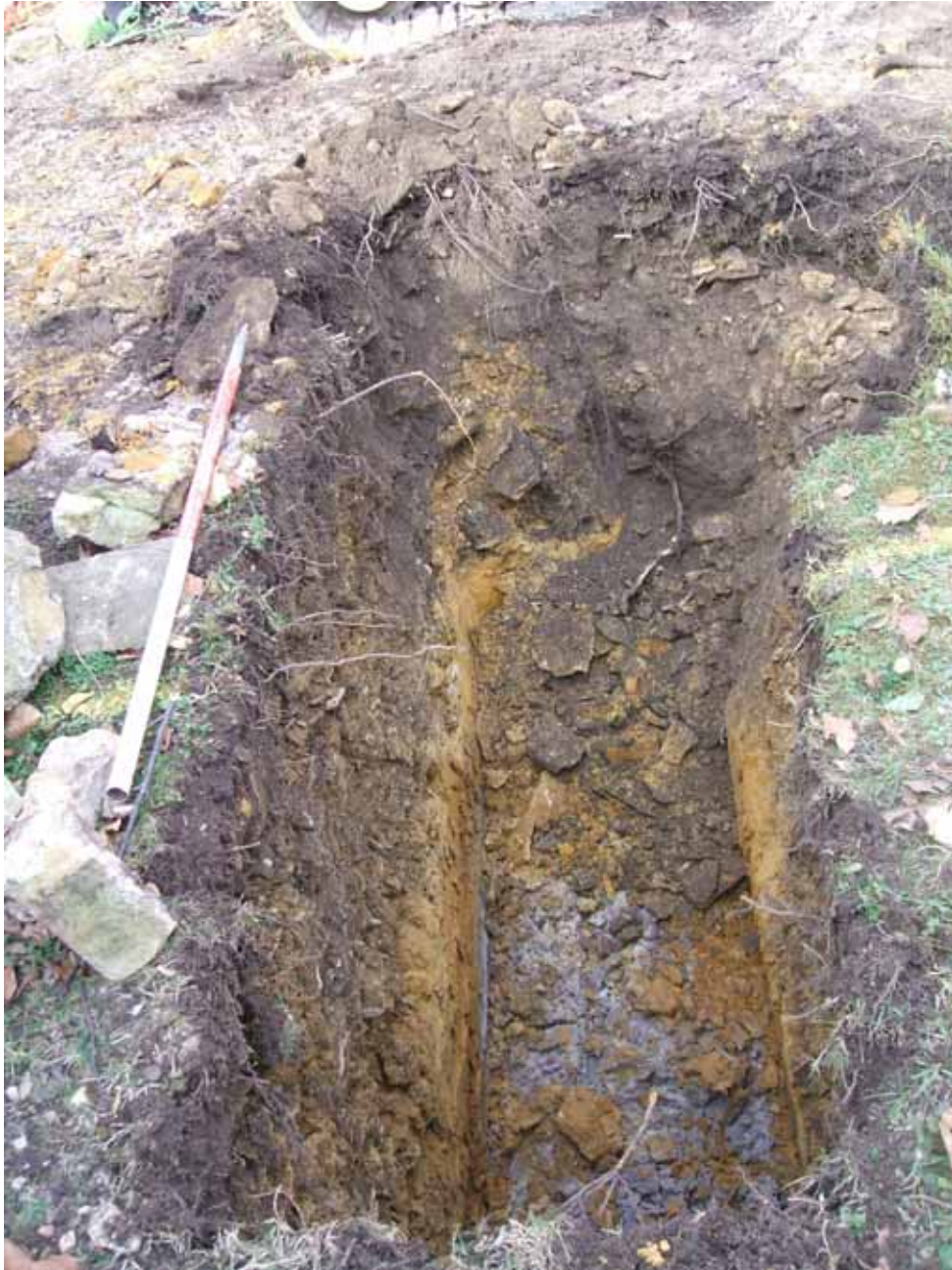
View of foundation trench looking west
