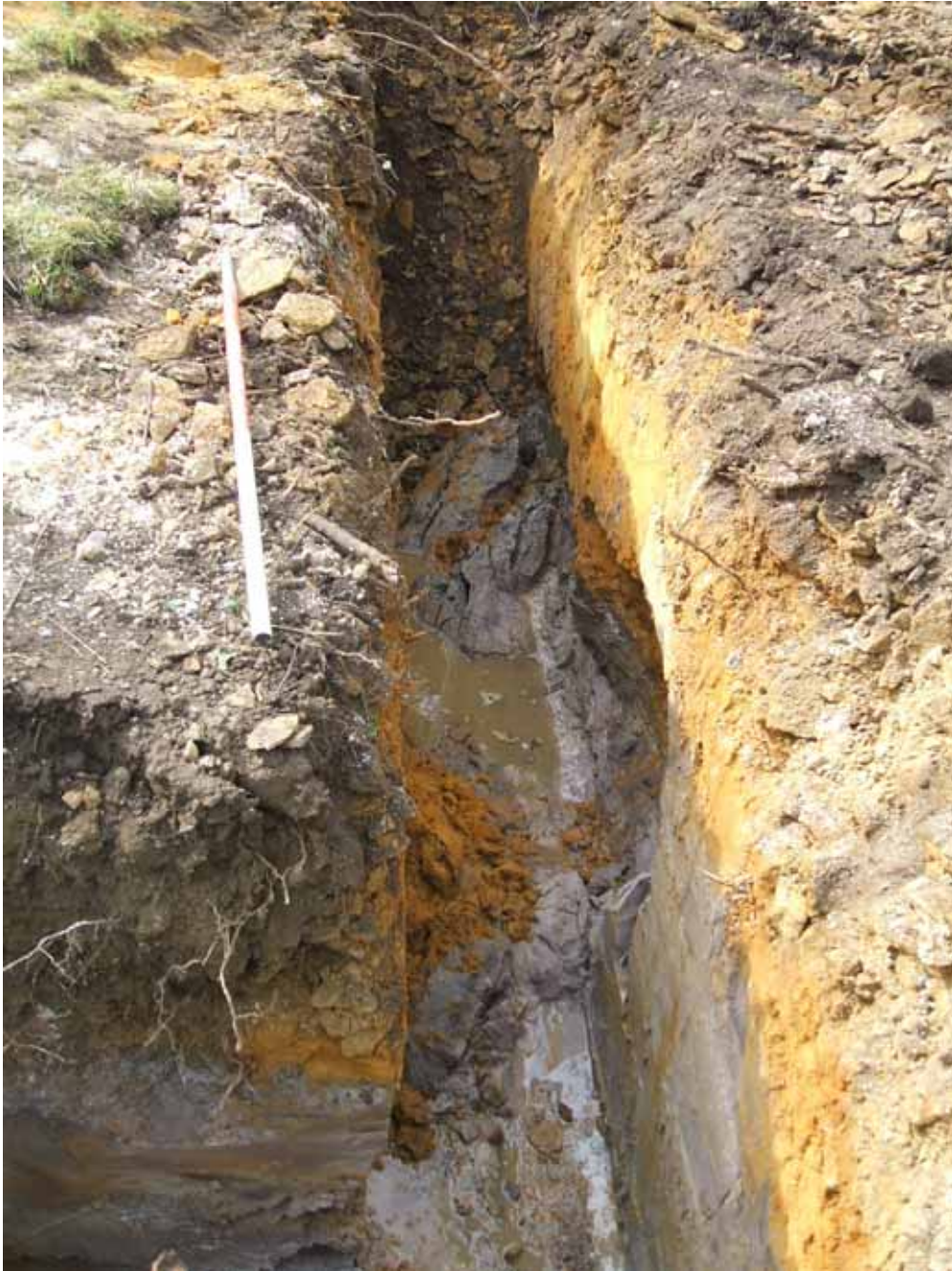
View of foundation trench looking south-west
