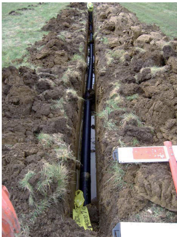
Plate 4: The new electricity cable prior to backfilling the trench
