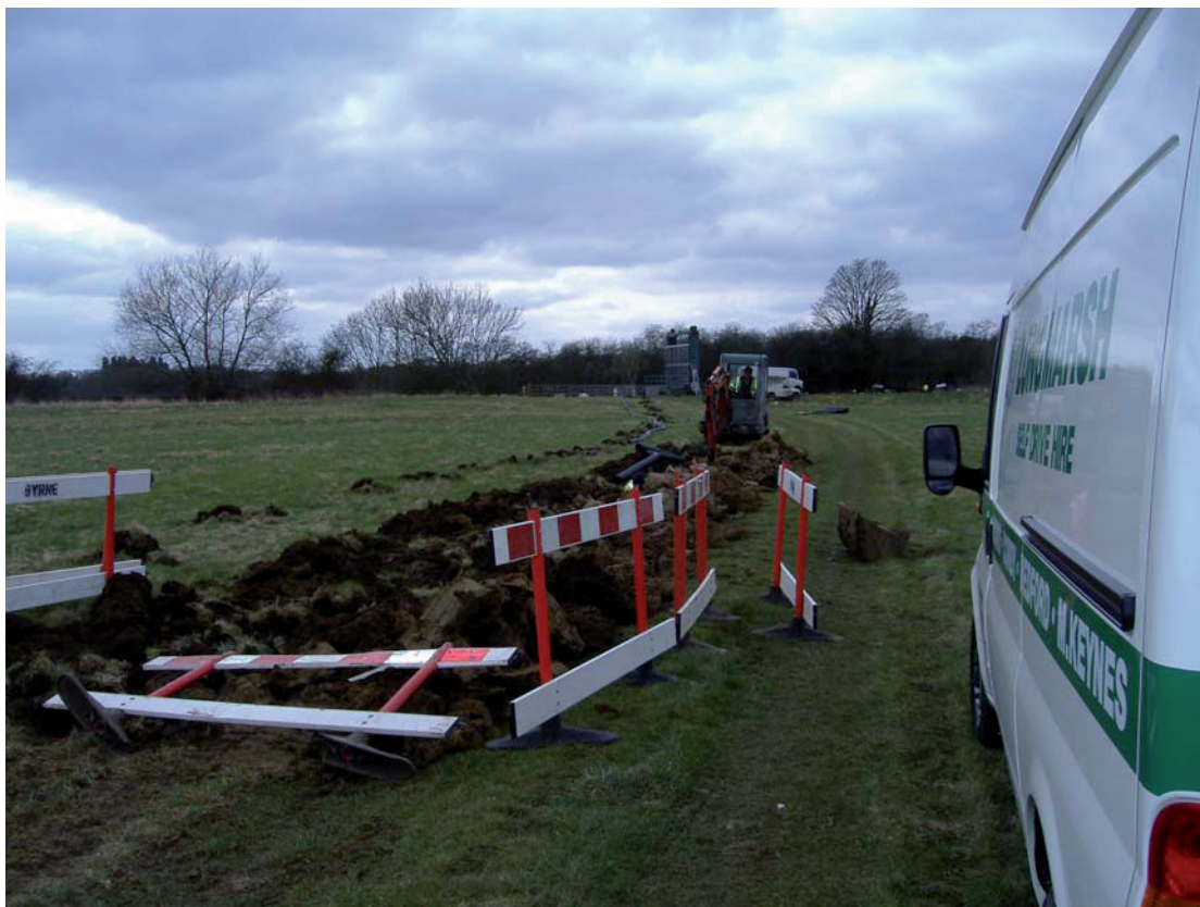
Plate 3: The excavation of the cable trench in progress
