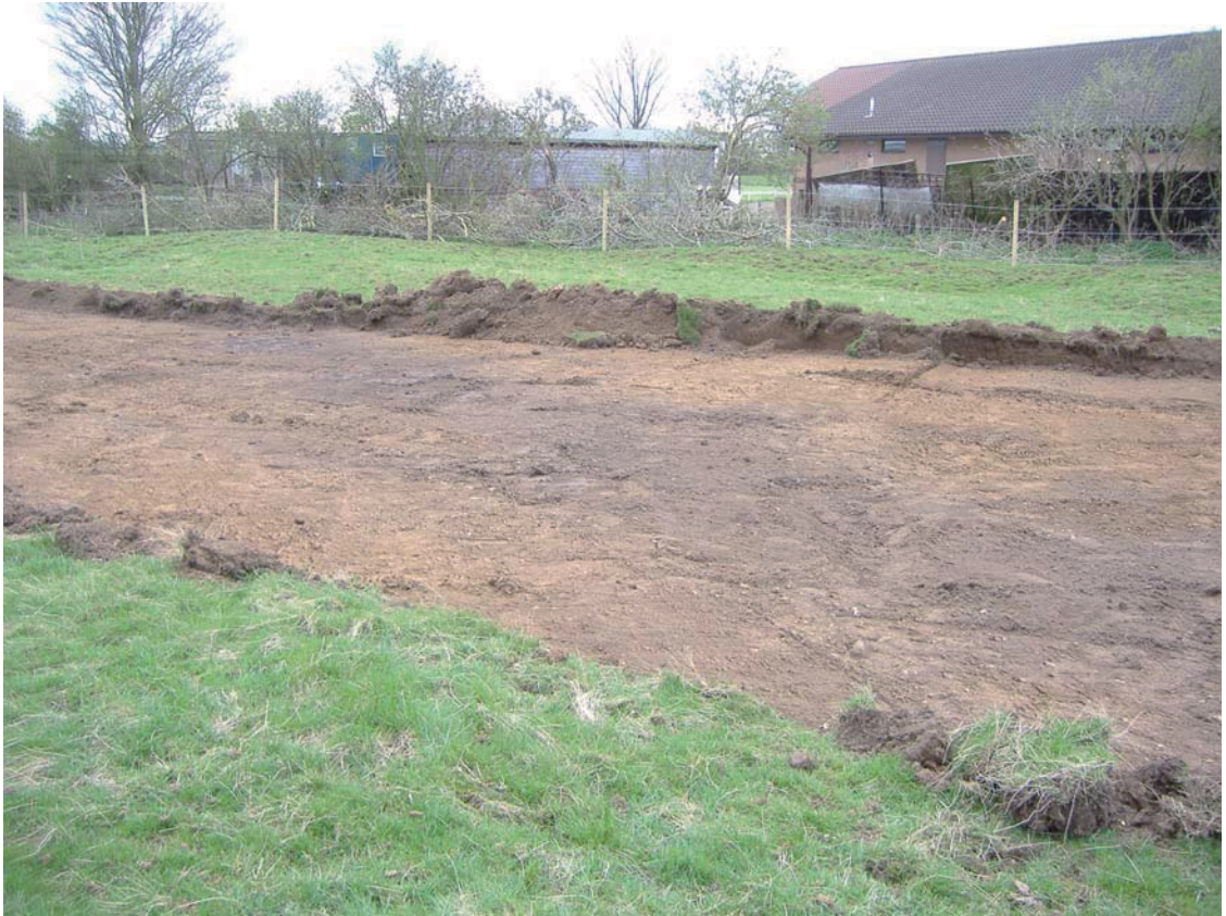
Plate 7: Area 2 during groundworks showing the dark line of a furrow
