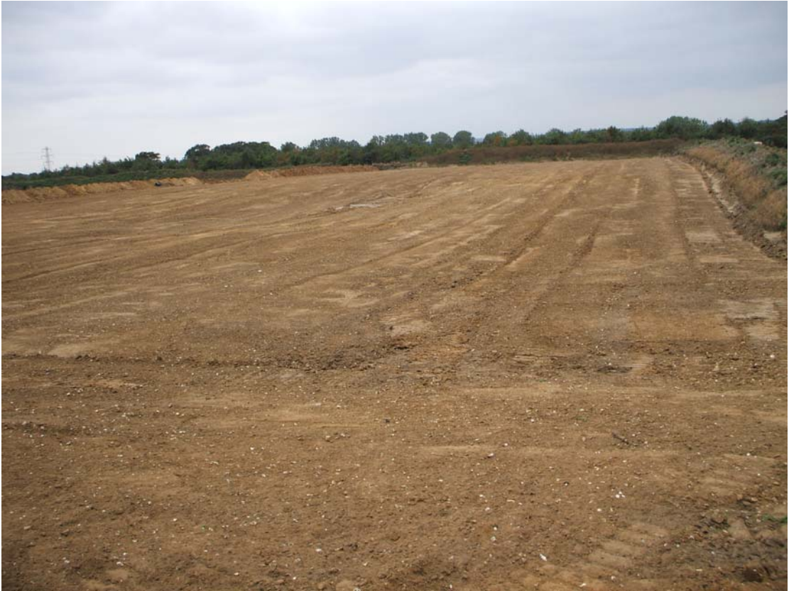
Plate 1: General view of stripped area looking south, September 2005
