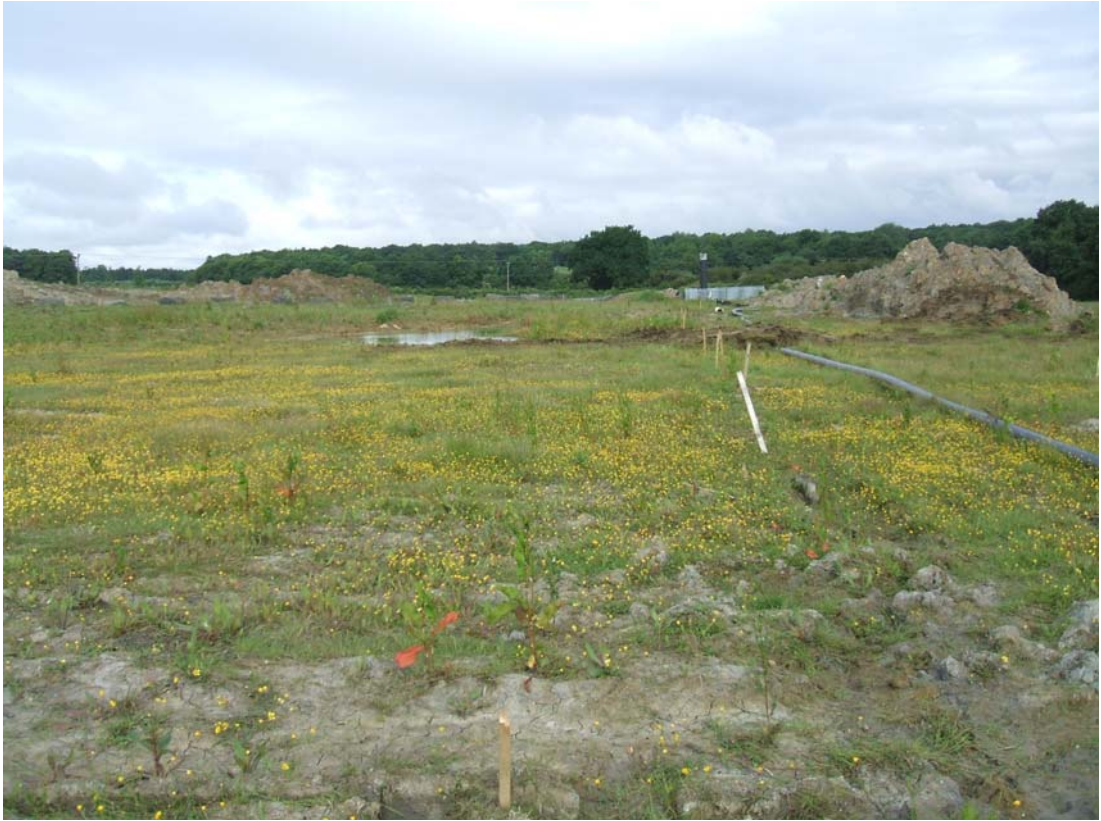
Plate 1: A view of the area of the new extension prior to the start of groundworks
