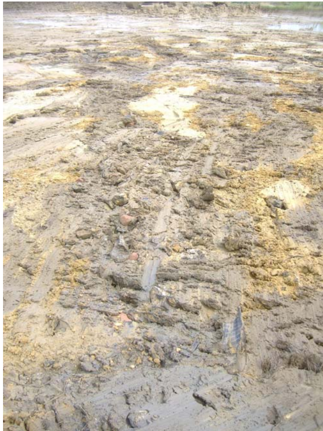
Plate 6: Vehicle rutting with tyre fragments in the track
