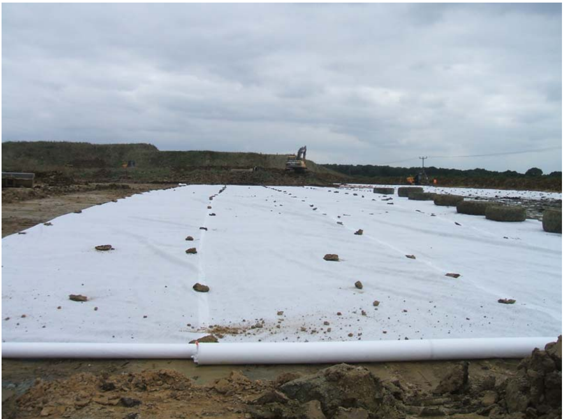
Plate 4: The membrane laid after the strip
