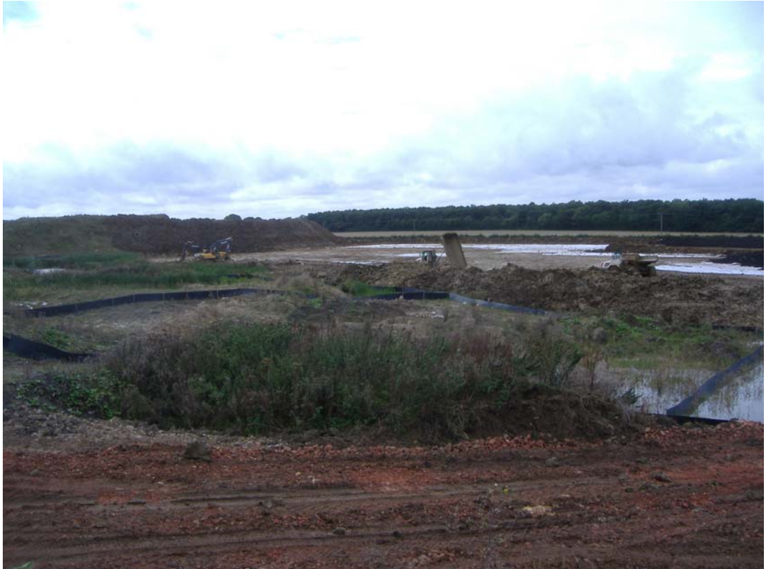
Plate 2: The area of the new extension during groundworks
