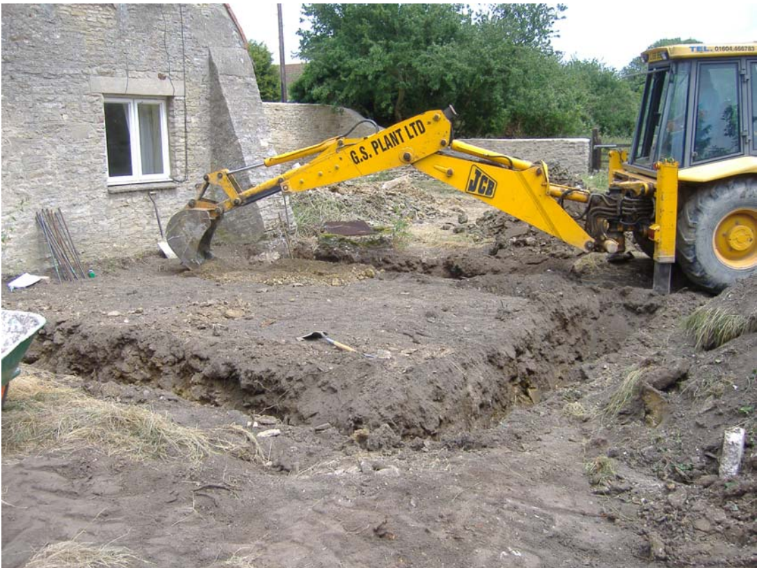
Plate 2: The excavation of the southern extension
