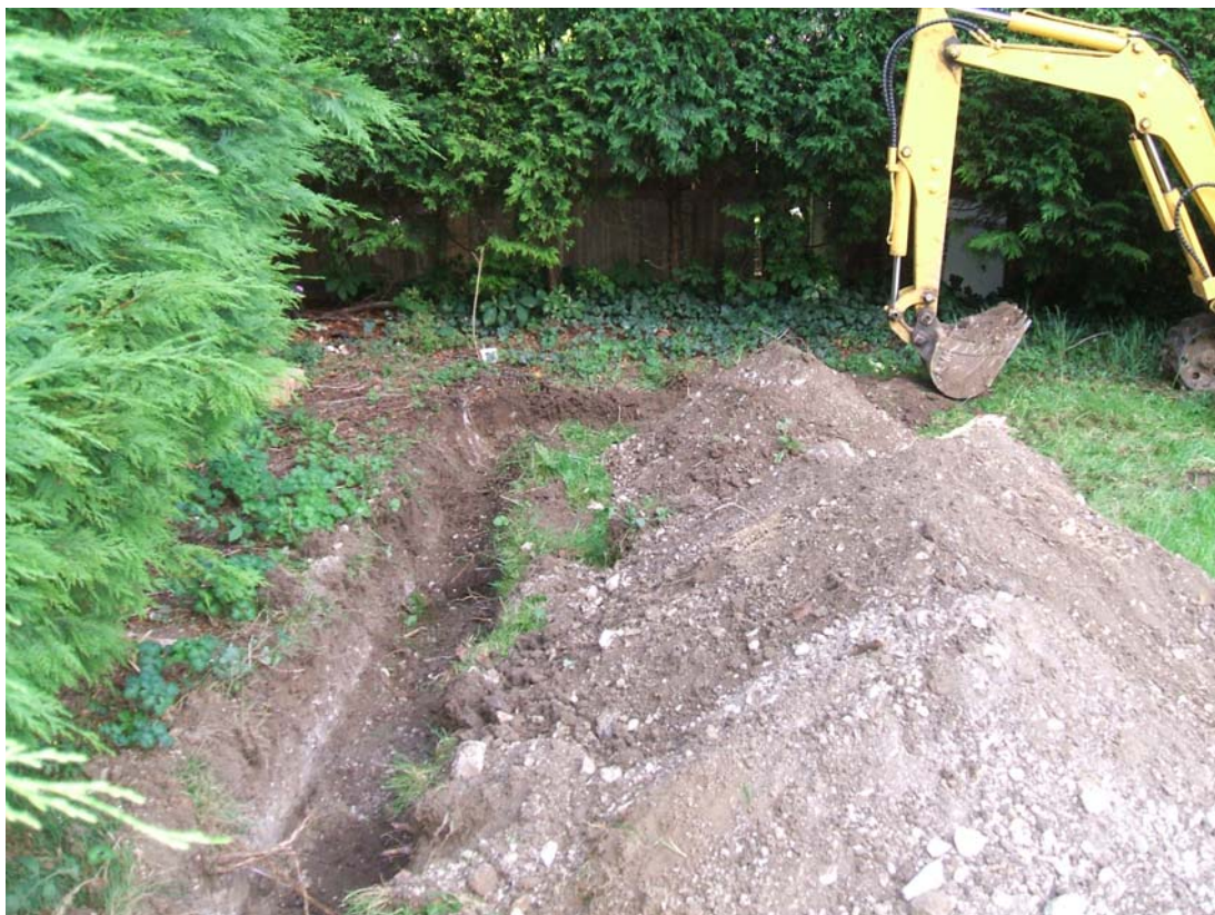
Plate 3: The garage foundations
