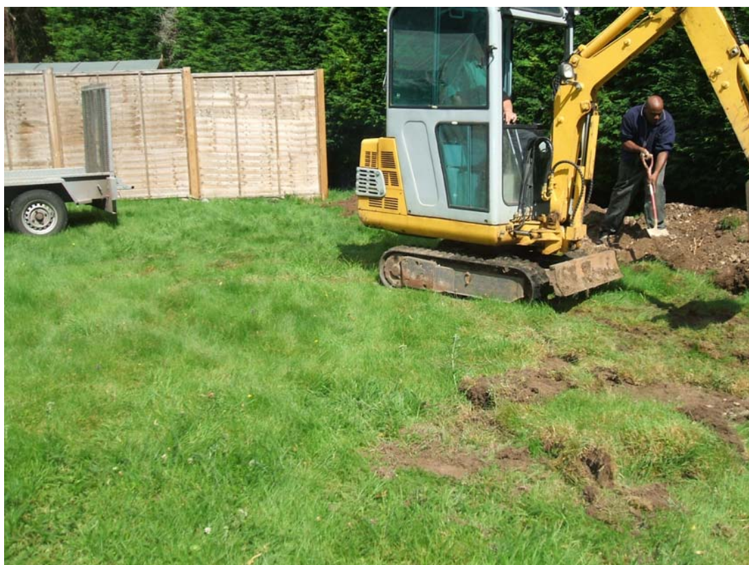
Plate 2: The development area during groundworks
