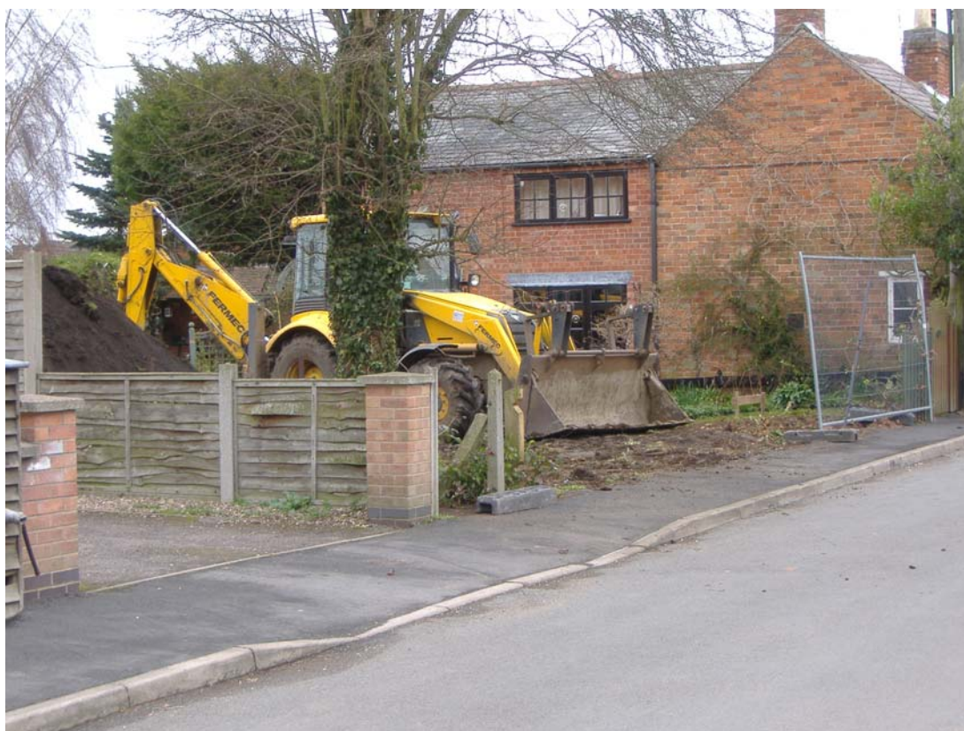
Plate 1: General view of 37 Peveril Road
