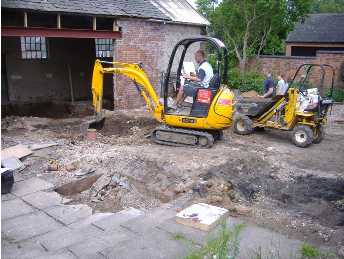
Plate 1: General view of the groundworks in progress
