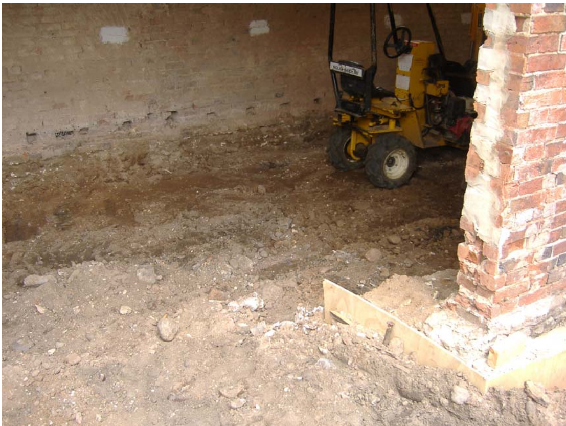
Plate 2: The groundworks within the barn
