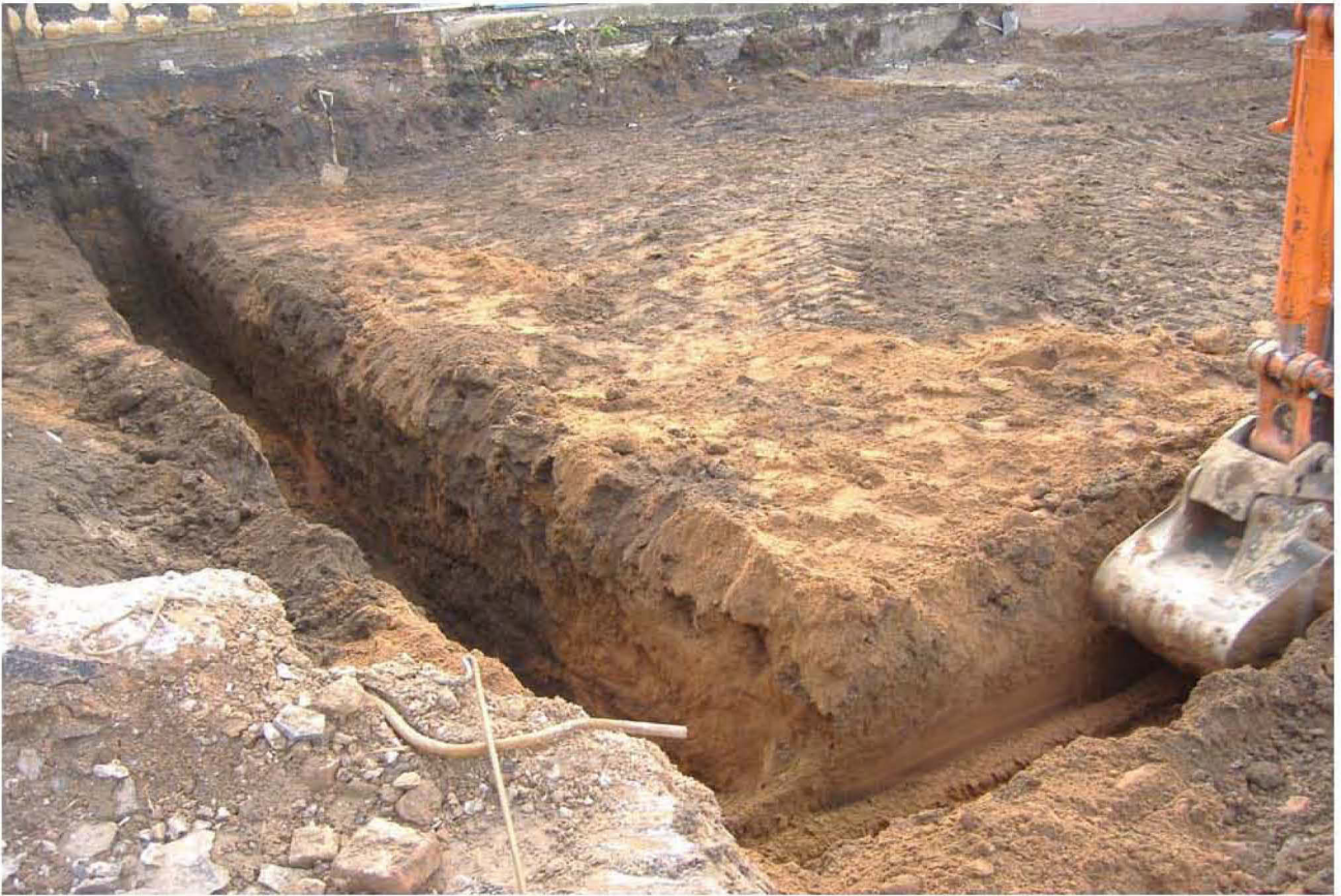
Plate 3: Foundation trench, view of natural and modern deposits, looking west
