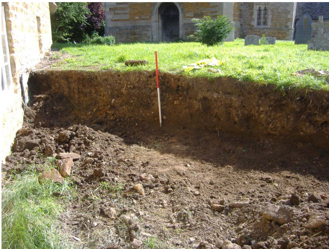
Plate 3: General view after removal of the retaining wall
