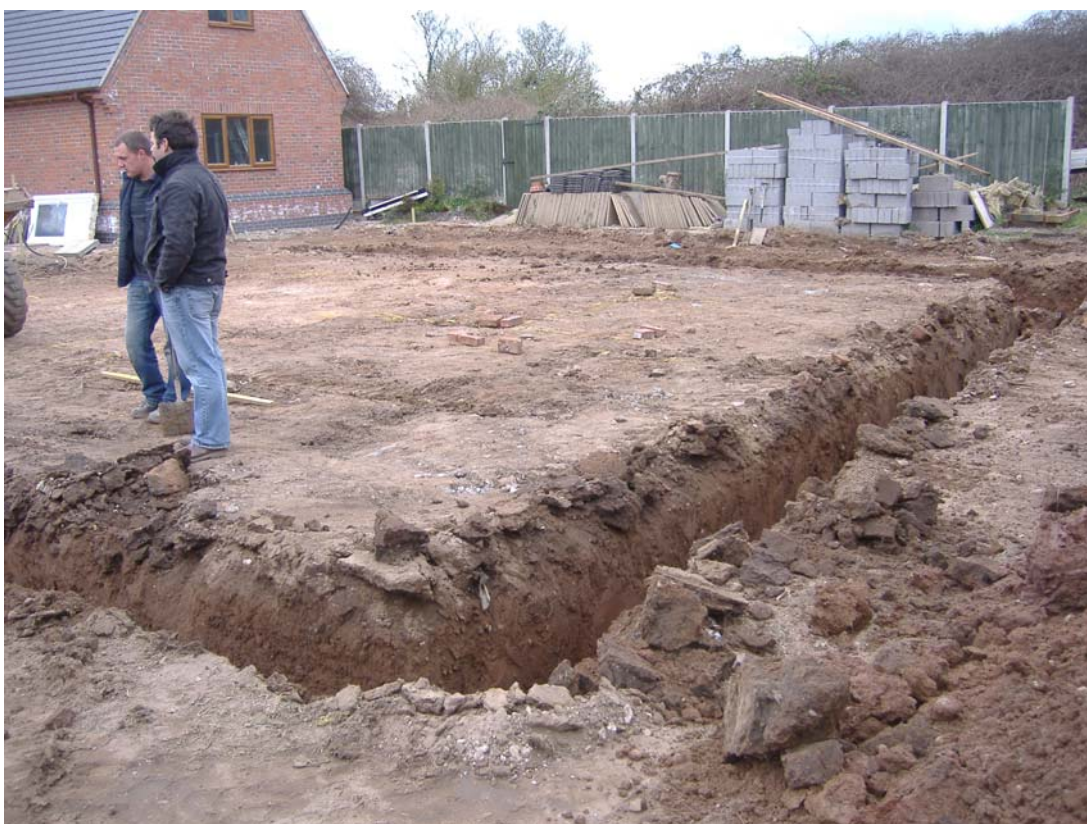
Plate 4: The ground-works nearing completion
