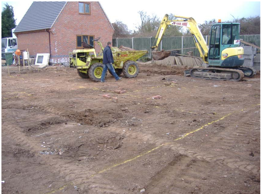
Plate 2: The ground-works in progress
