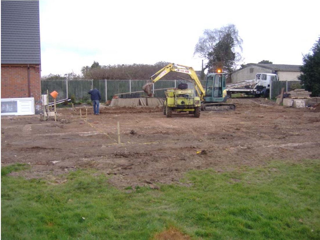
Plate 1: General view of the development area at the start of ground-works
