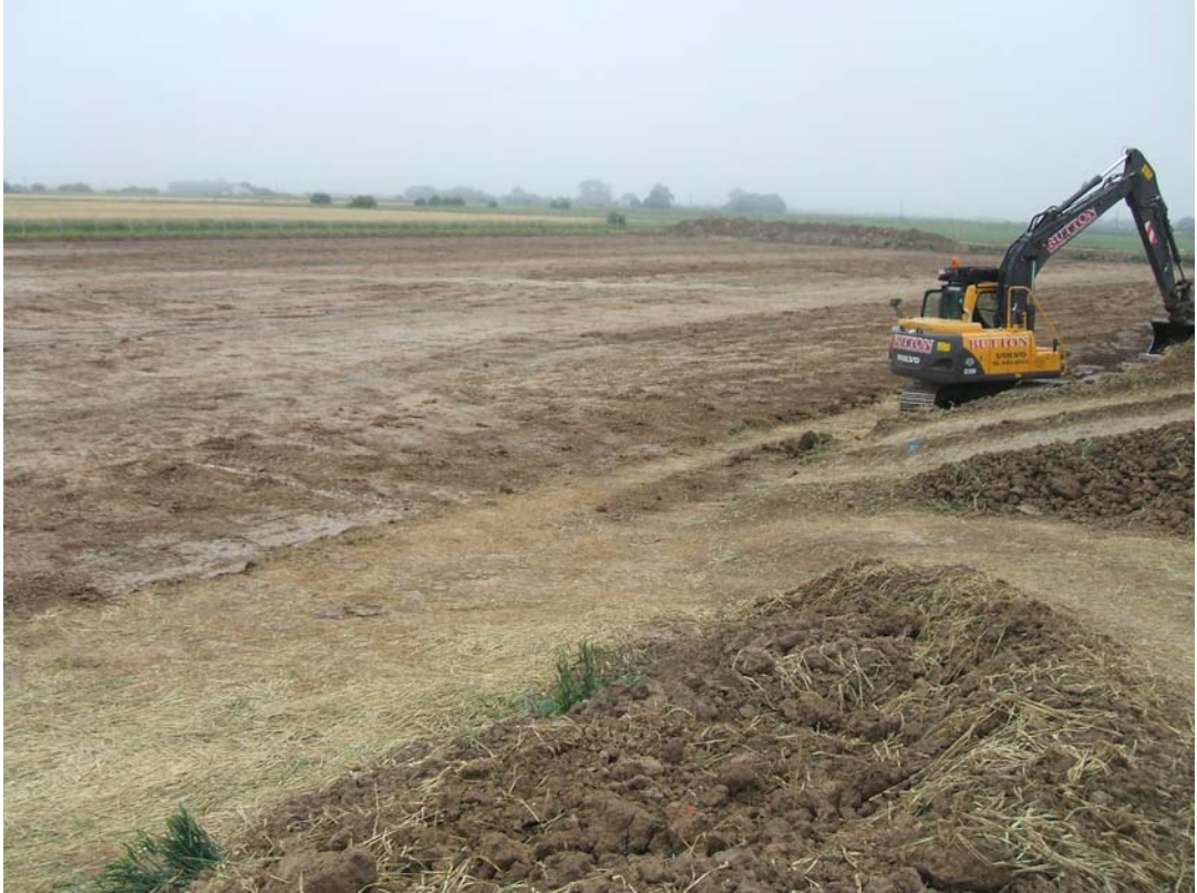
Plate 1: General view of the groundworks
