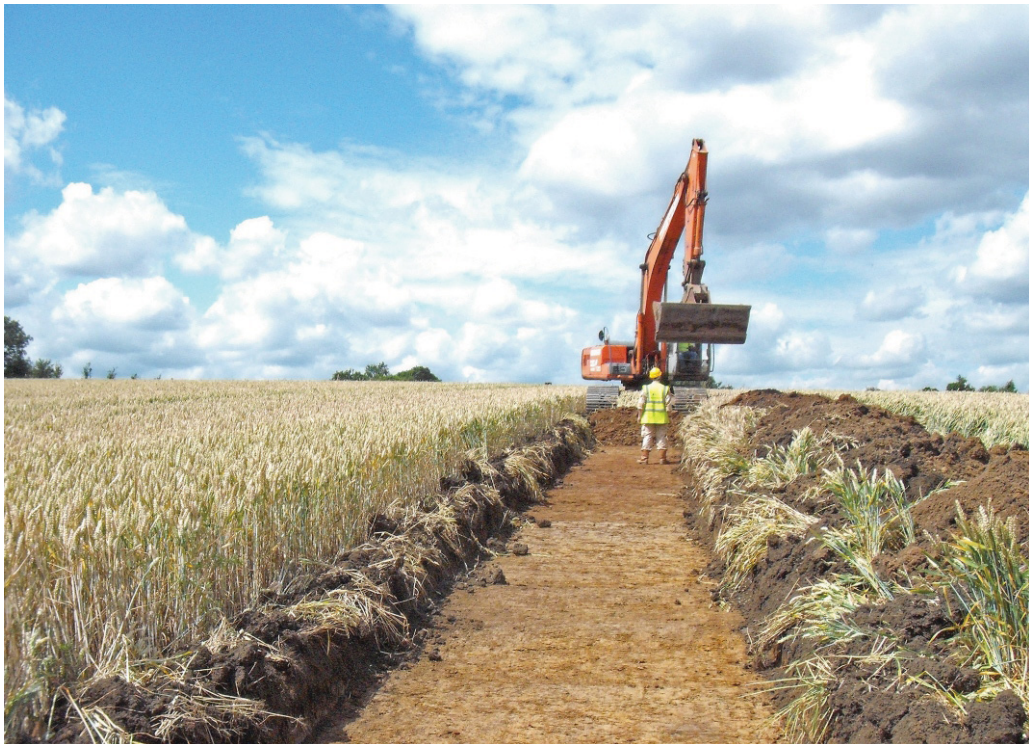
Fig 3: Machine excavation of trench 9 in progress, looking west
