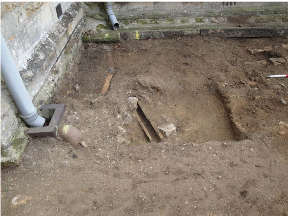
Drain (107), salt glaze pipes (117) and field drain (115), looking south Fig 14
