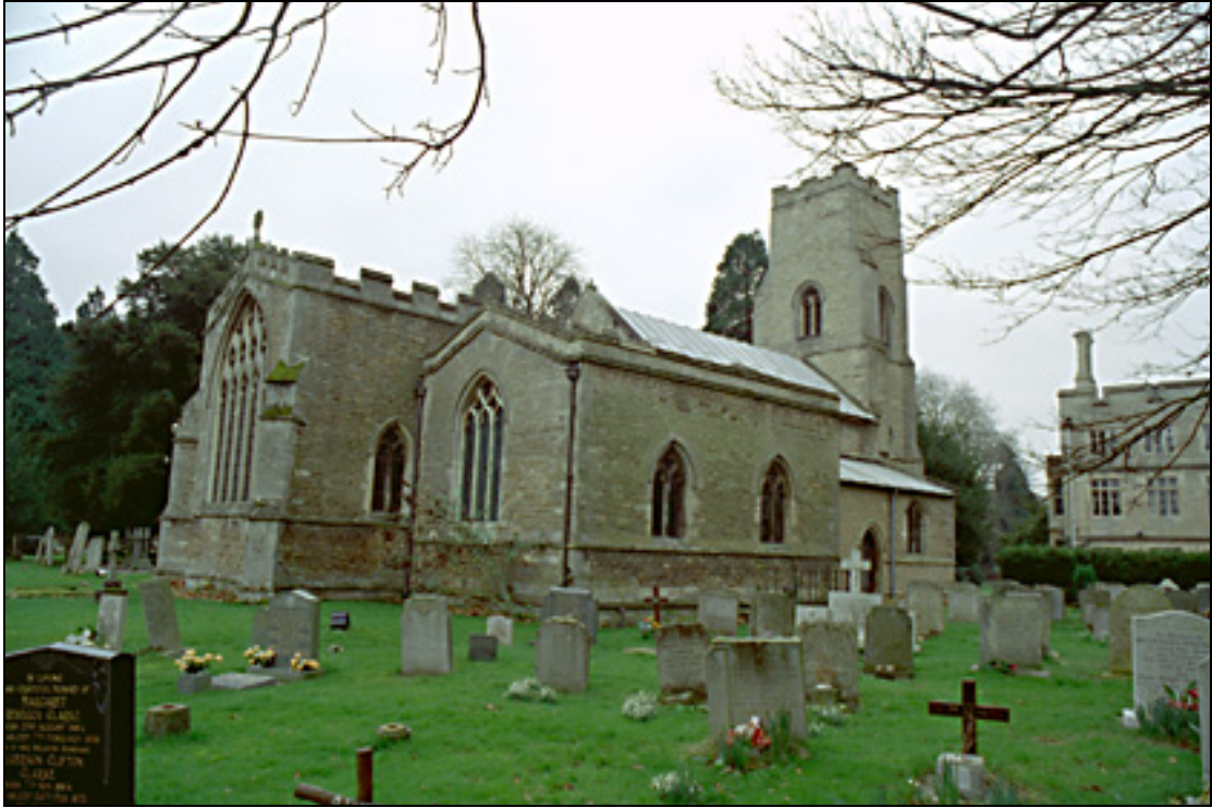
Holy Trinity Church, looking south-west
