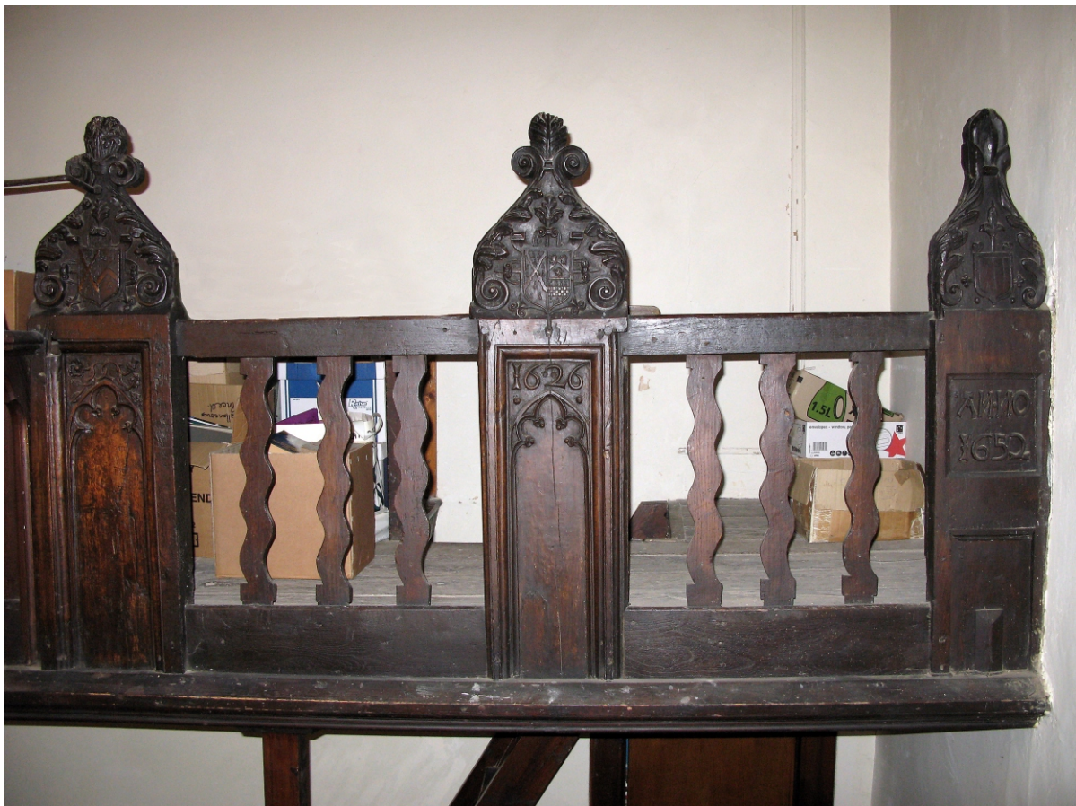
Fig 20: Re-used pew ends and wavy splat balusters
