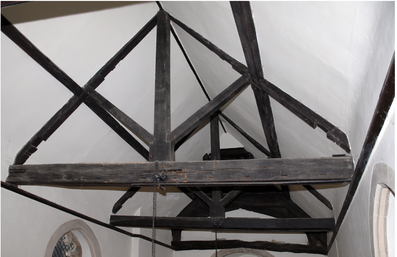
Fig 17: Roof interior, looking south
