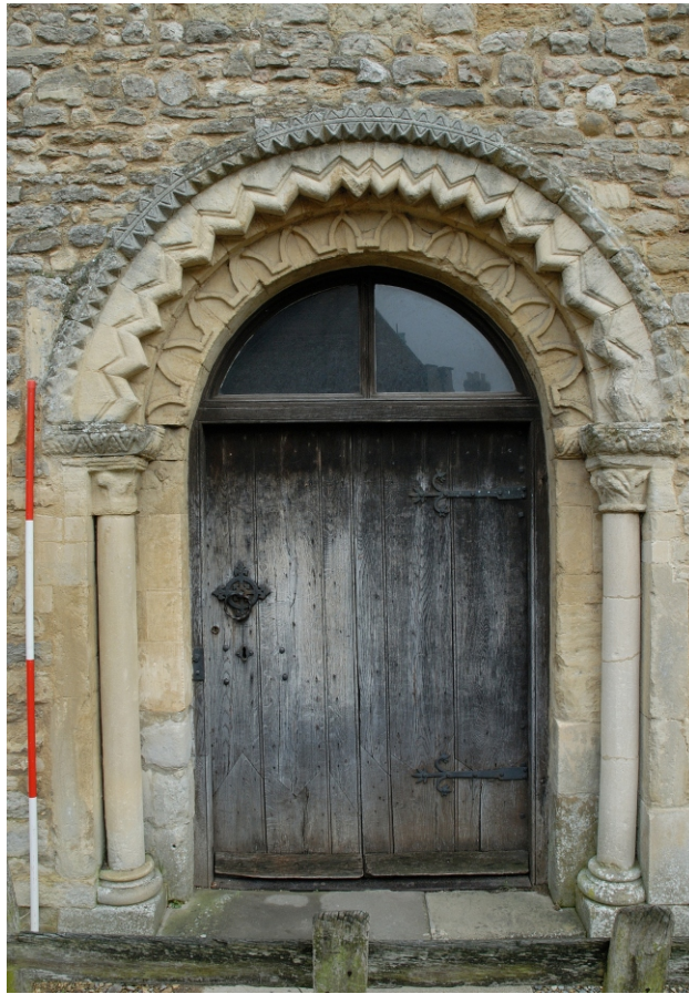
Fig 7: Detail of west entrance
