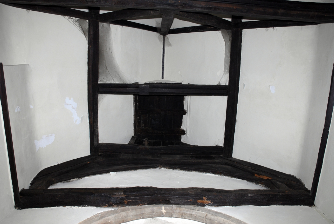
Fig 18: Southernmost truss and former cupola access
