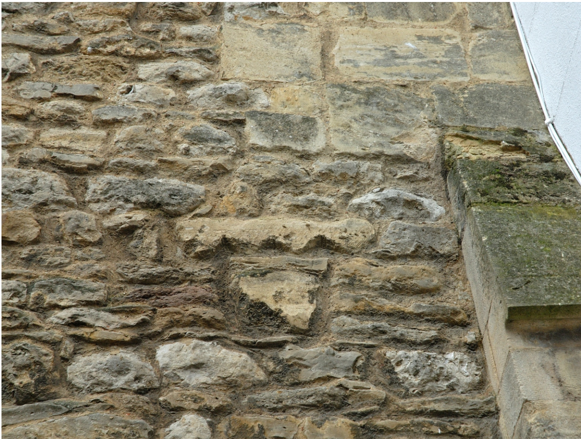
Fig 4: Re-used architectural fragment and possible put-log hole
