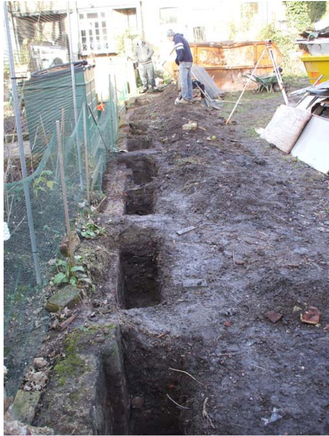
Plate 1: Site looking north
