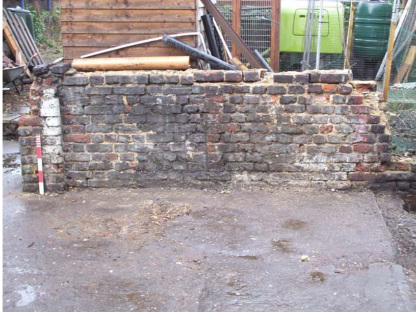
Plate 12: Upstanding fabric of 19th (?) century wall [2]
