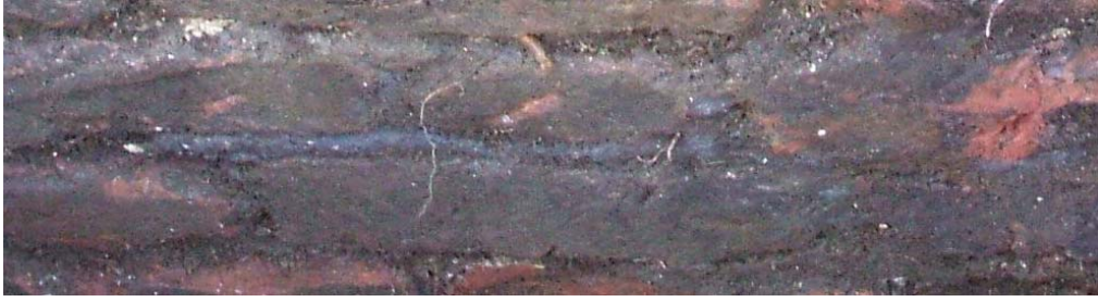
Plate 11: Re-pointing in 18th (?) century wall [3]
