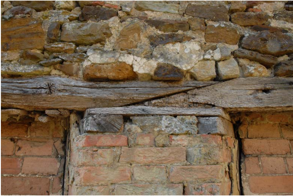
Plate 5: Detail of scarf joint and wooden blocks
