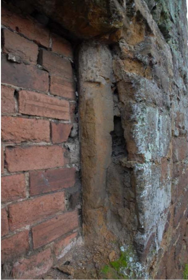
Plate 3: Detail of window bar slot
