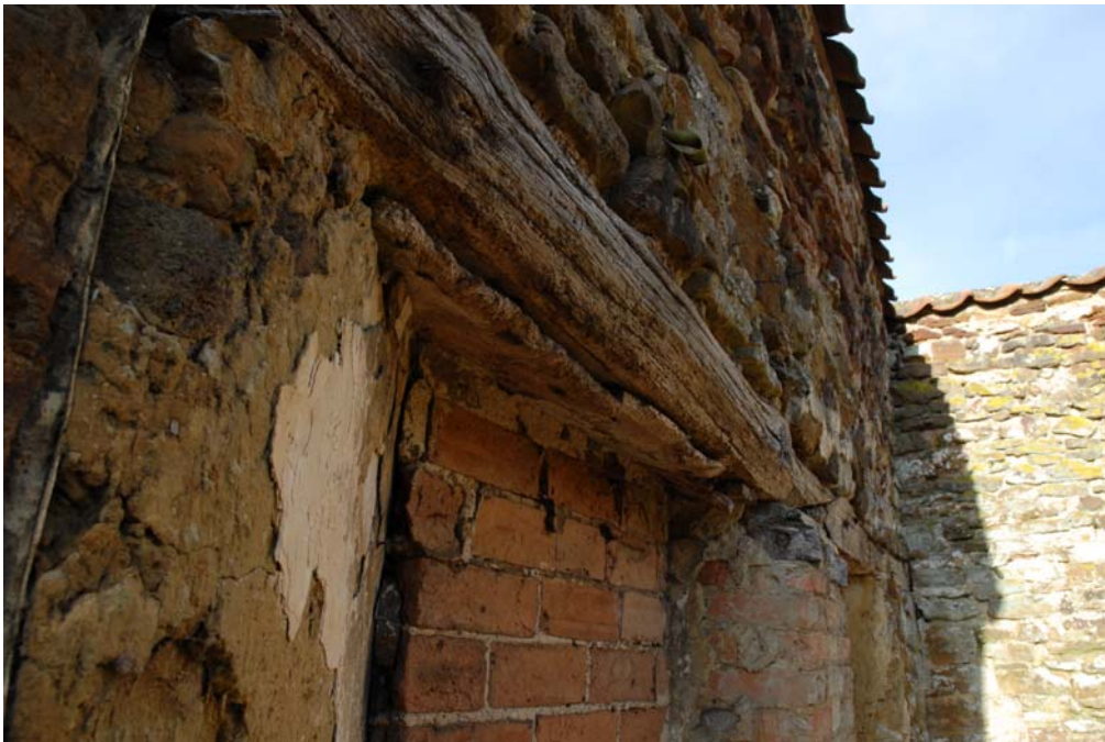
Plate 6: Detail of planking below lintel
