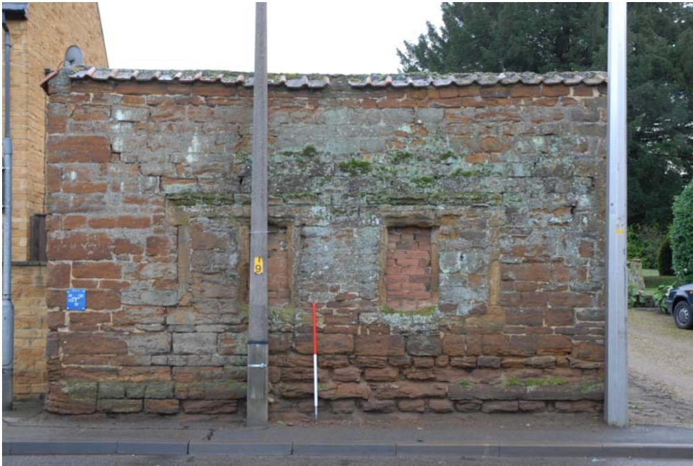
Plate 1: West facing elevation
