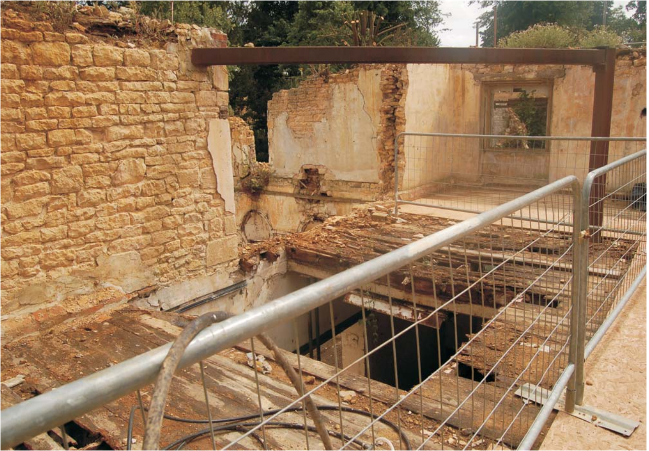
Plate 29: Room 2, first floor, looking south
