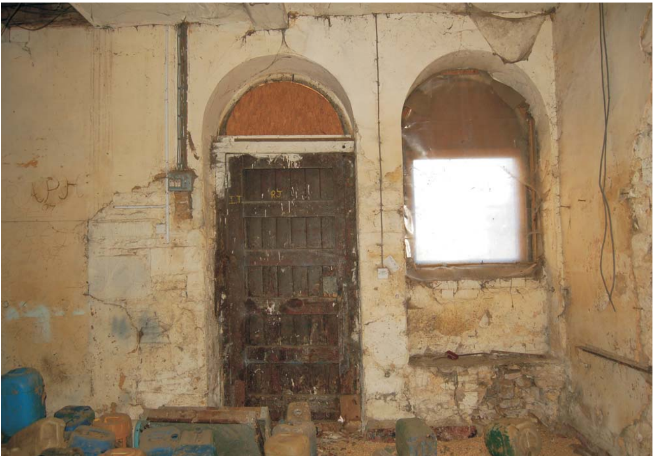
Plate 24: Interior view of original door and window to Stable 2, looking east
