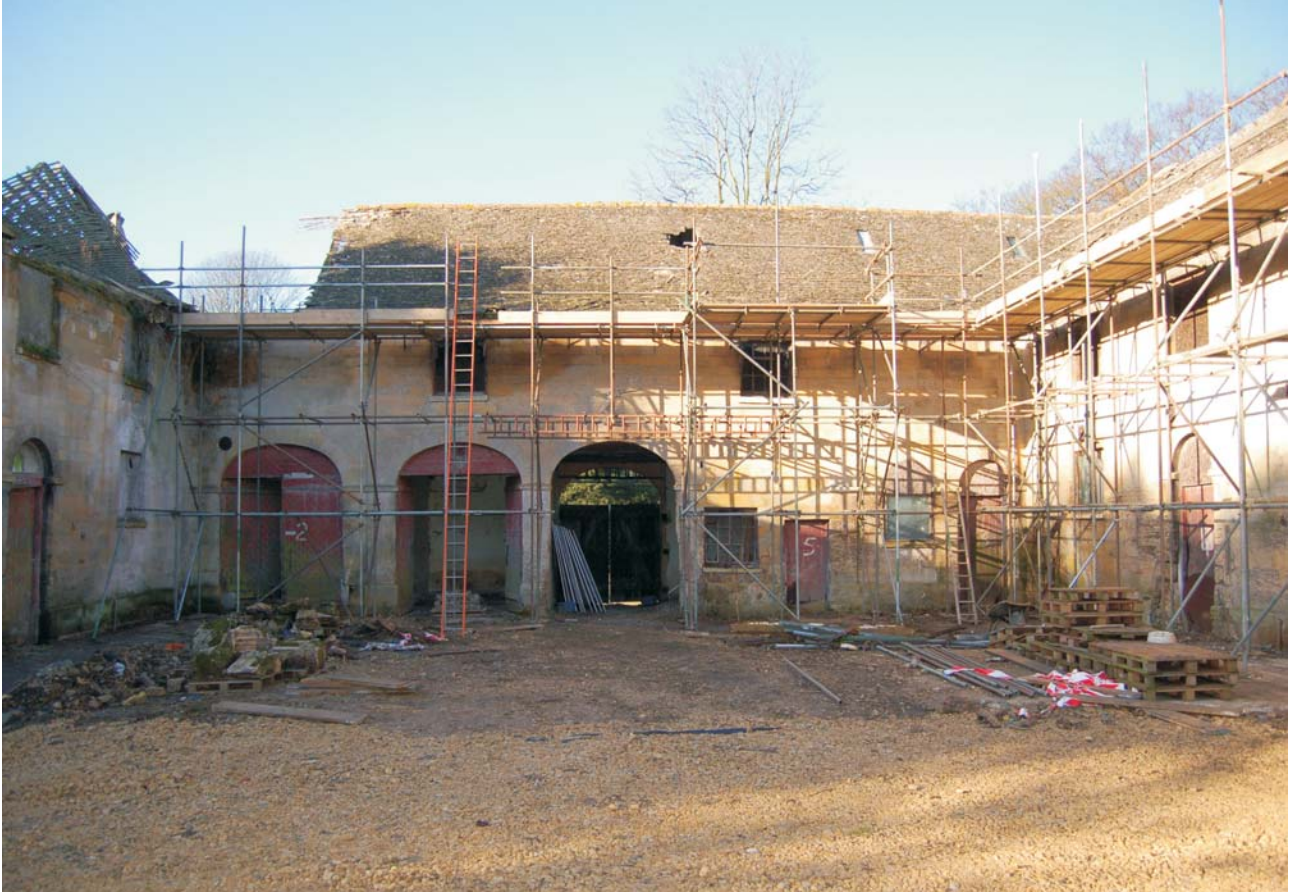
Plate 14: East facade of west range, looking west
