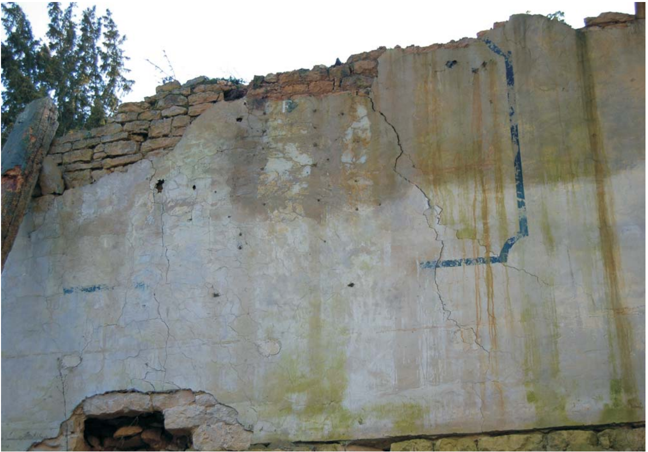
Plate 17: Decorative paint scheme, first floor- south wing, looking south
