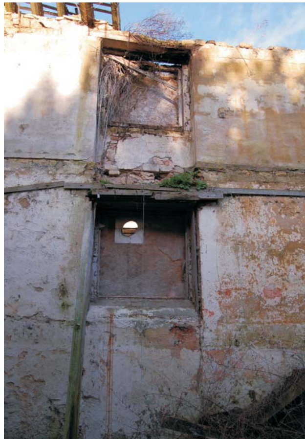
Plate 16: Window details at ground and first floor- south wing, looking north
