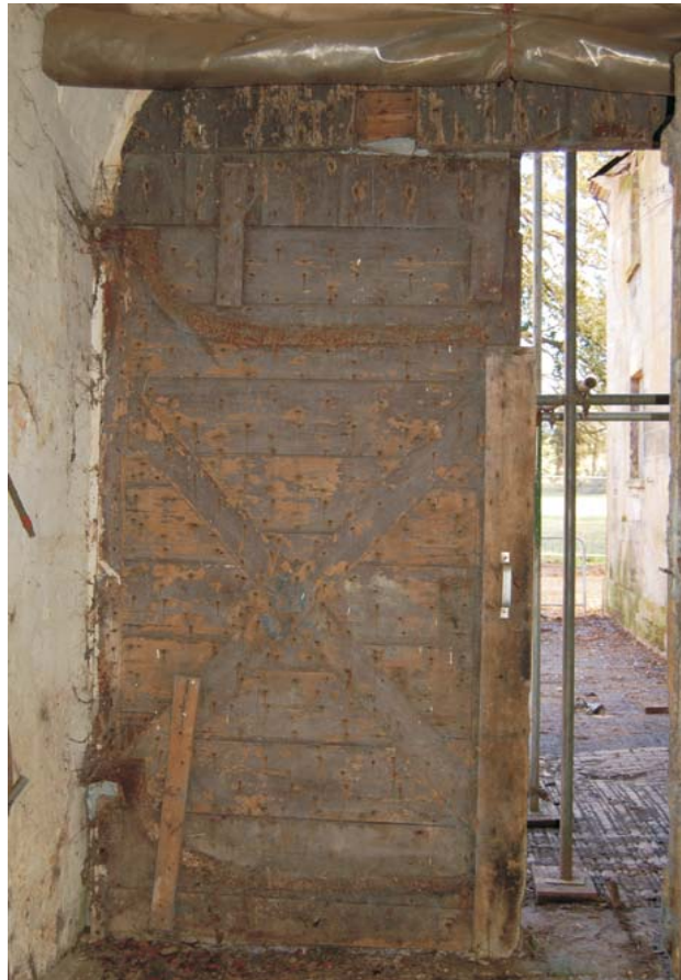
Plate 22: Internal surface of carriage house door
