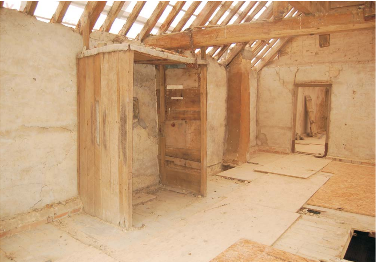
Plate 30: Oak cupboard against west wall in Room 3, looking north-west
