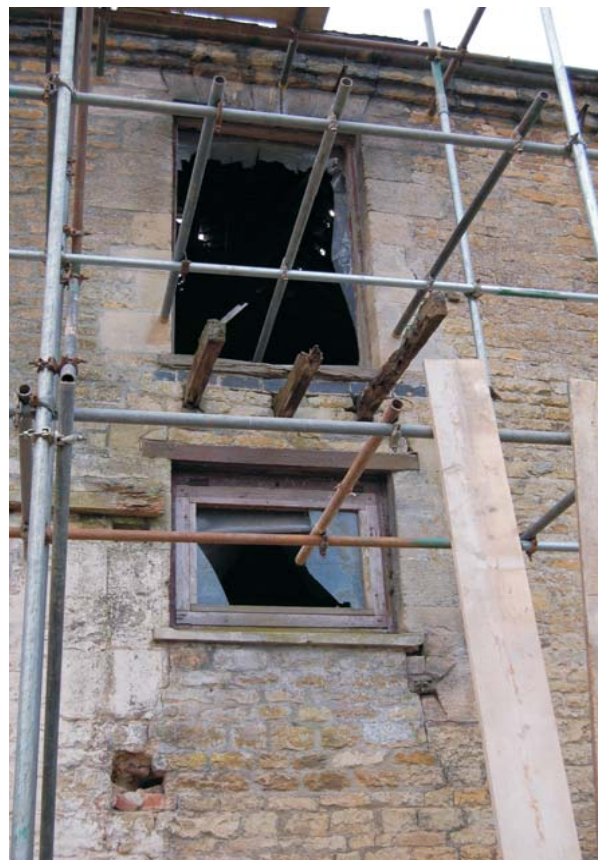
Plate 10: North facade looking south
