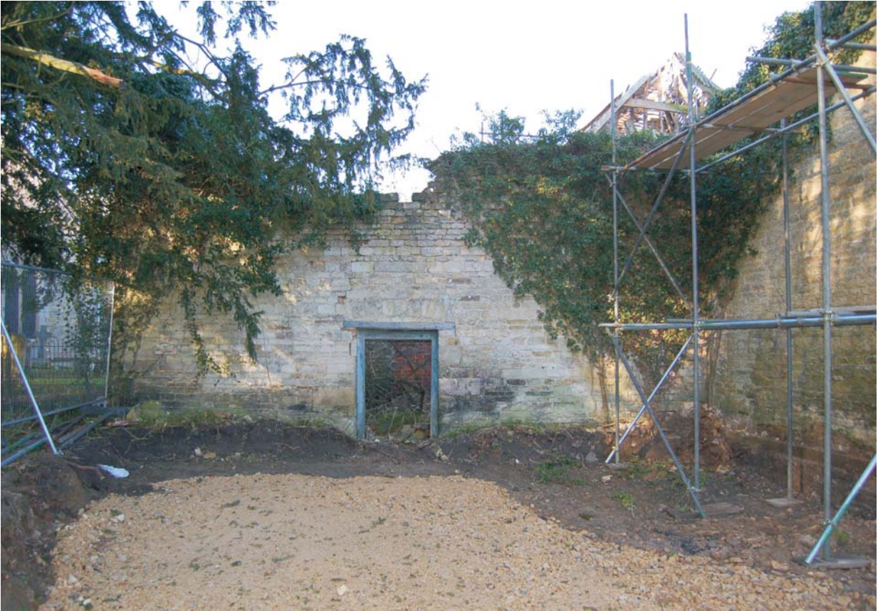
Plate 7: Door in the east facade of the "Chapel" looking west
