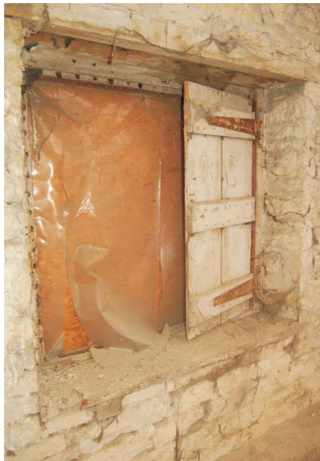
Plate 38: Shutter on central window in south wall of Room 5
