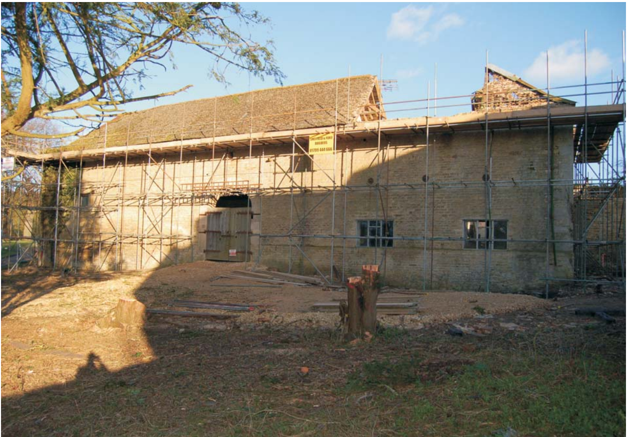
Plate 3: The west side of the stables
