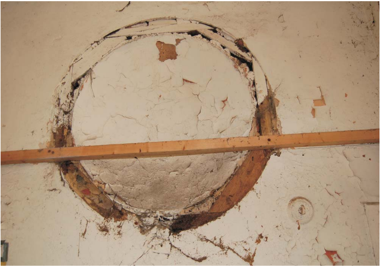
Plate 27: Hay rack roundel in east wall of Stable 4 with tethering hook, looking east
