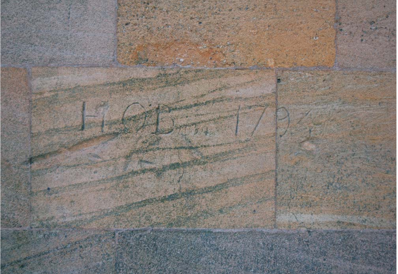
Plate 12: Graffiti; H O'B 1794 on east facade of north wing
