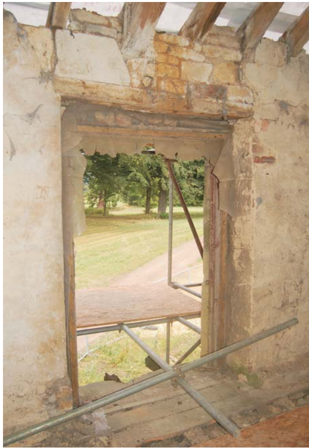
Plate 35: Former window converted to hay-loft door in north wall of Room 4
