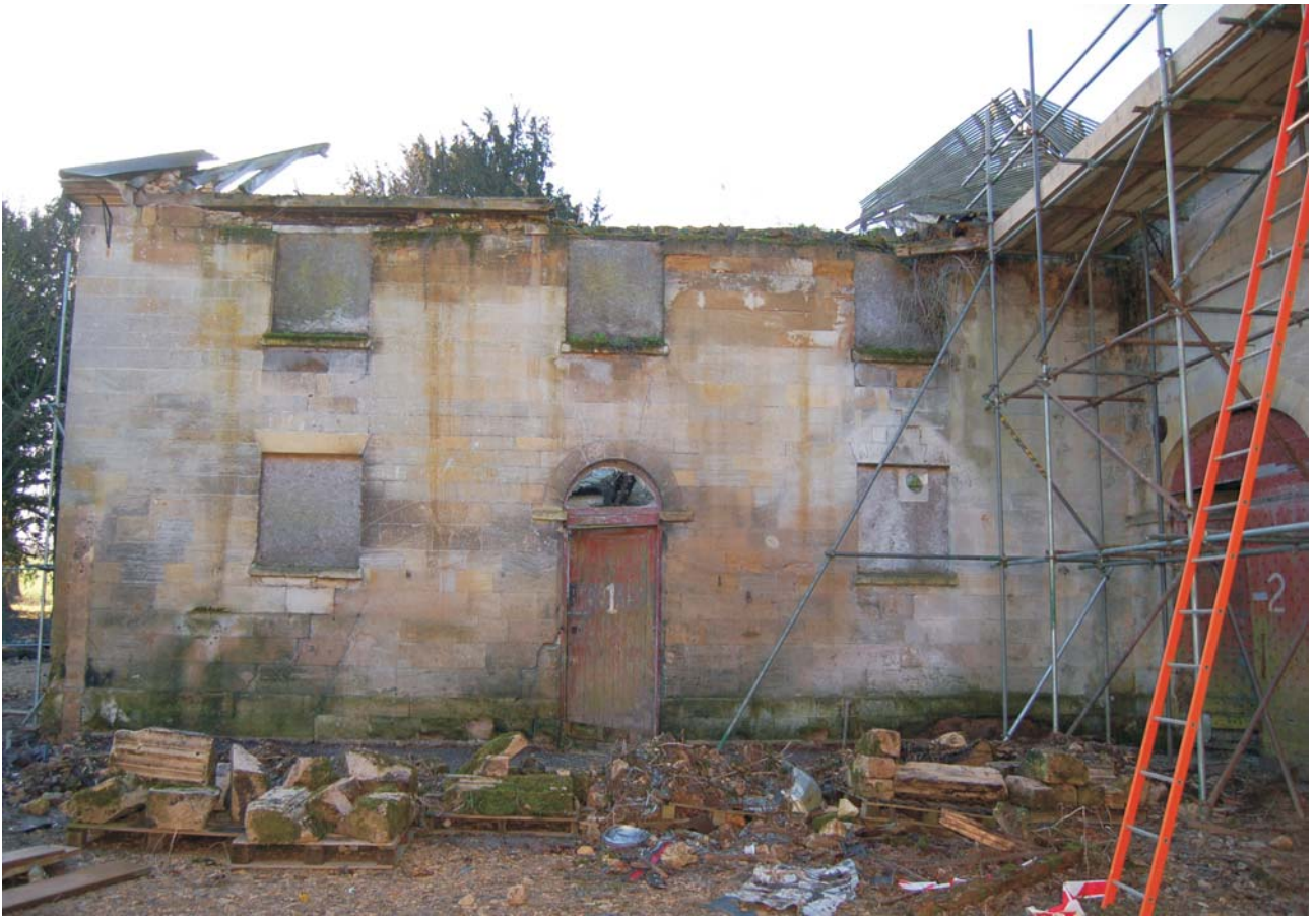
Plate 13: North facade of south wing looking south
