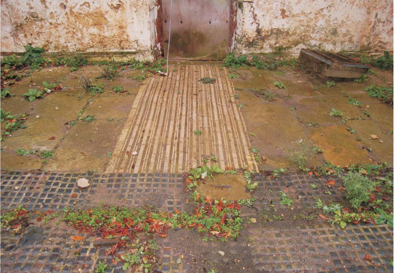
Plate 20: Paviers in stable 1, looking north
