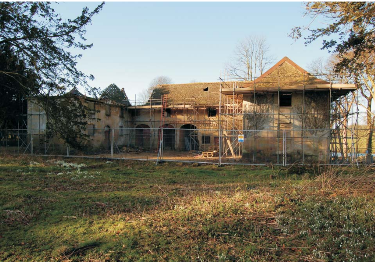
Plate 2: The stables from the north-east
