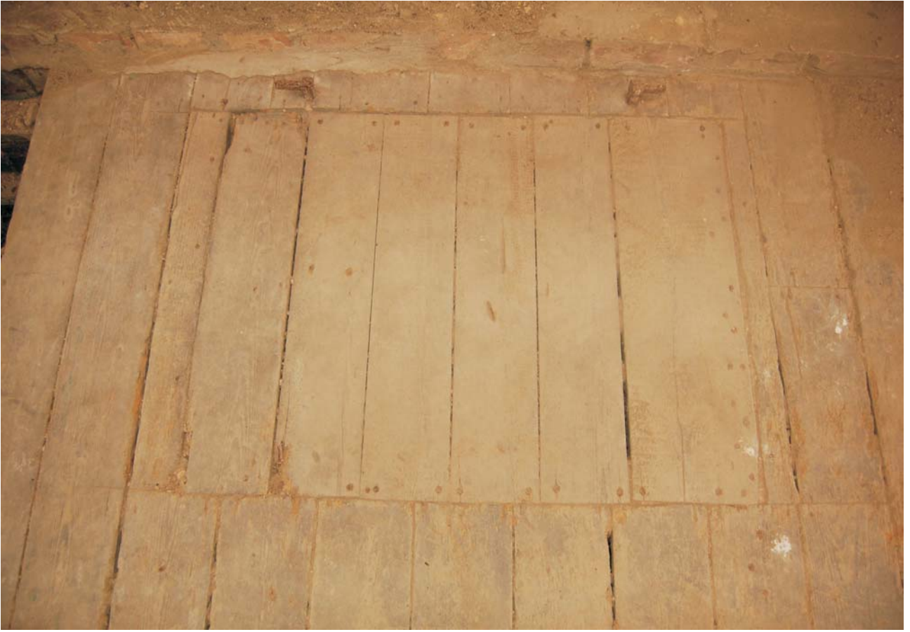
Plate 39: Trapdoor against north wall of Room 4 with hinges on north side
