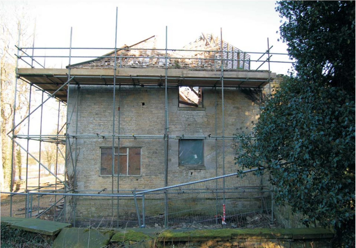
Plate 5: South facade showing original and later window openings
