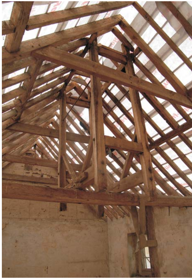
Plate 31: Oak frame for the clock, centre of Room 3, looking north-east
