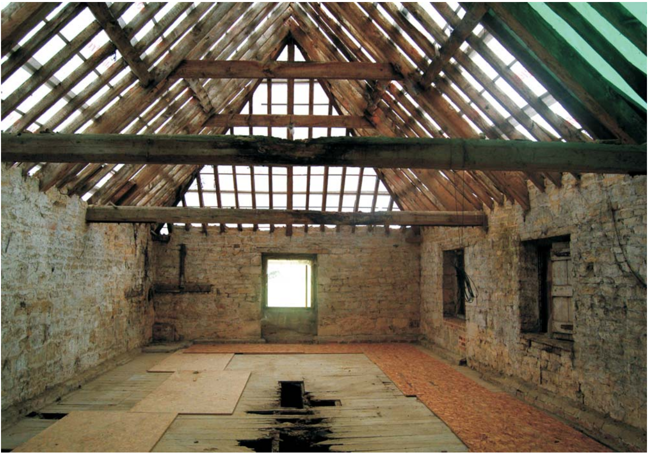
Plate 37 Room 5 looking east showing un-plastered walls and roof structure
