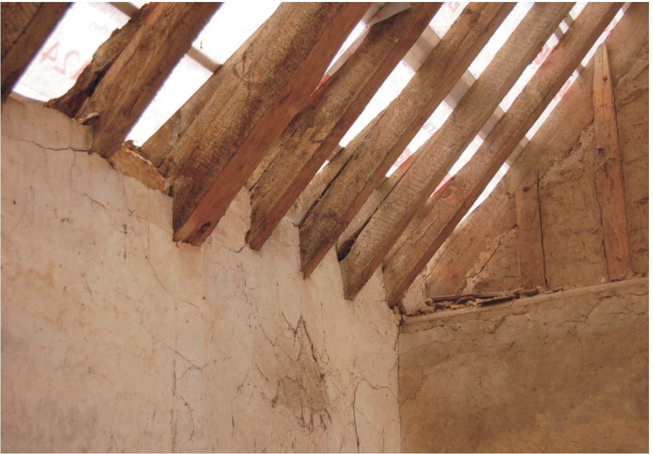
Plate 33: Configuration of rafters and splockets, north side of Room 4, looking south
