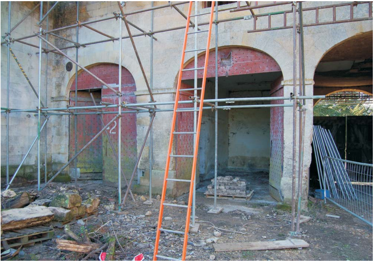
Plate 21: Carriage house doors from the stable yard
