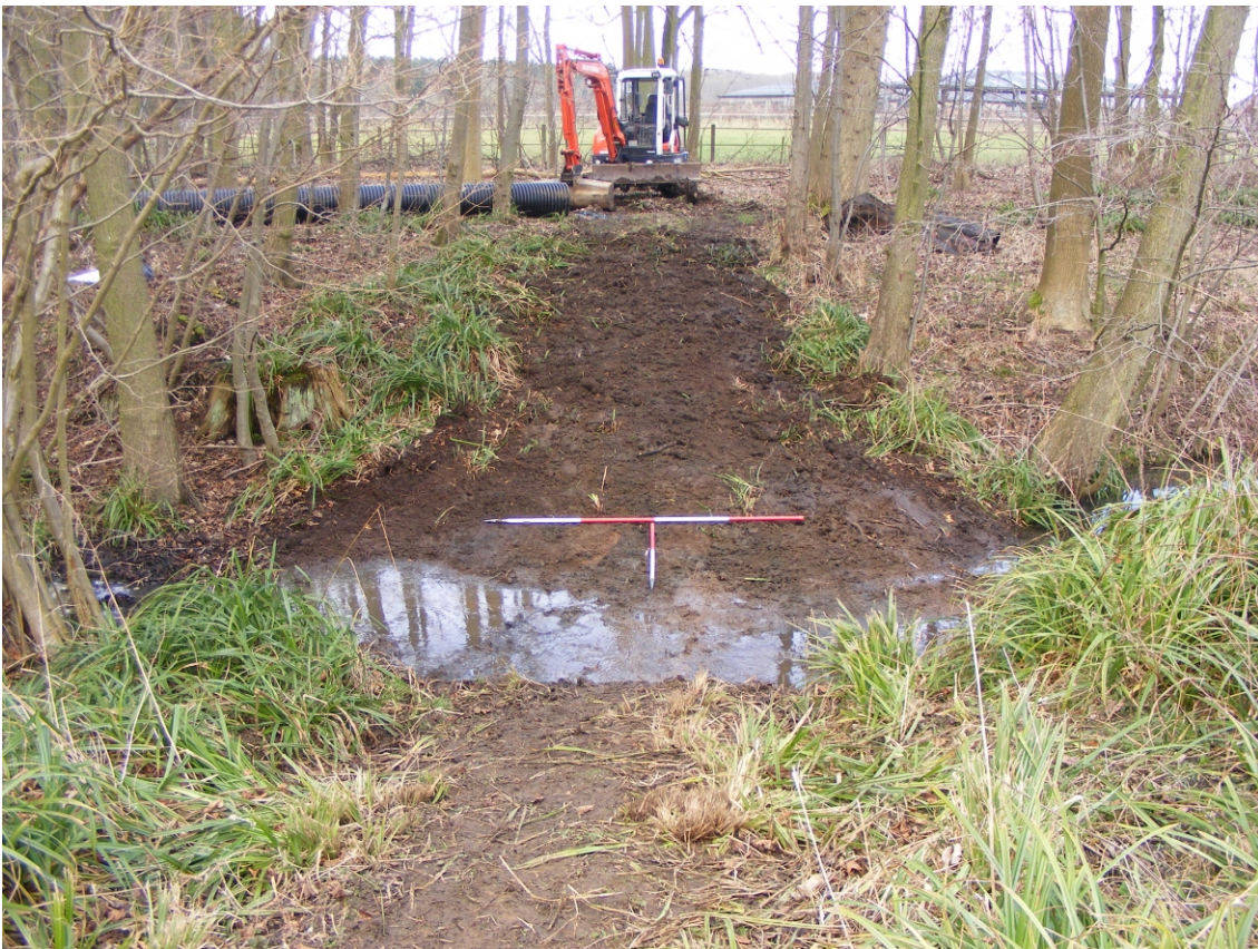
Plate 4: North moat arm/culvert [5], looking north after soil removal
