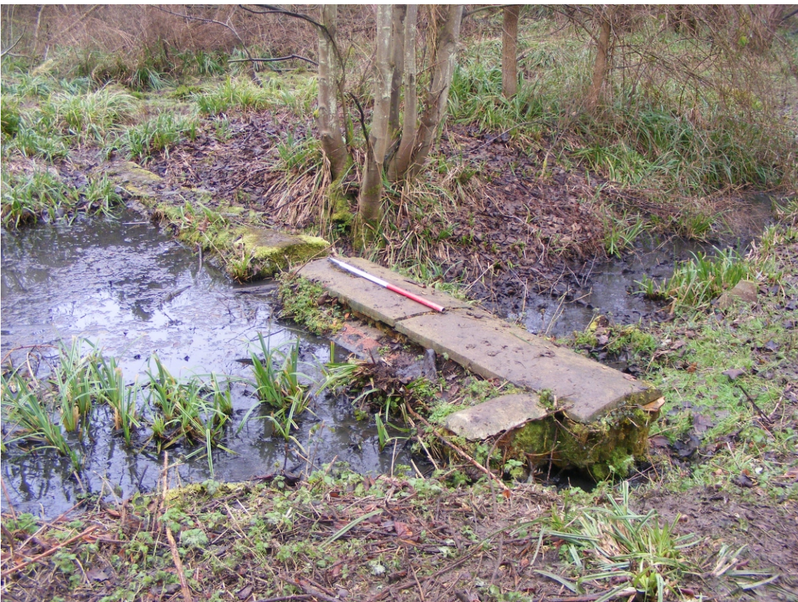
Plate 6: The dam [8] pre-works, looking south-east
