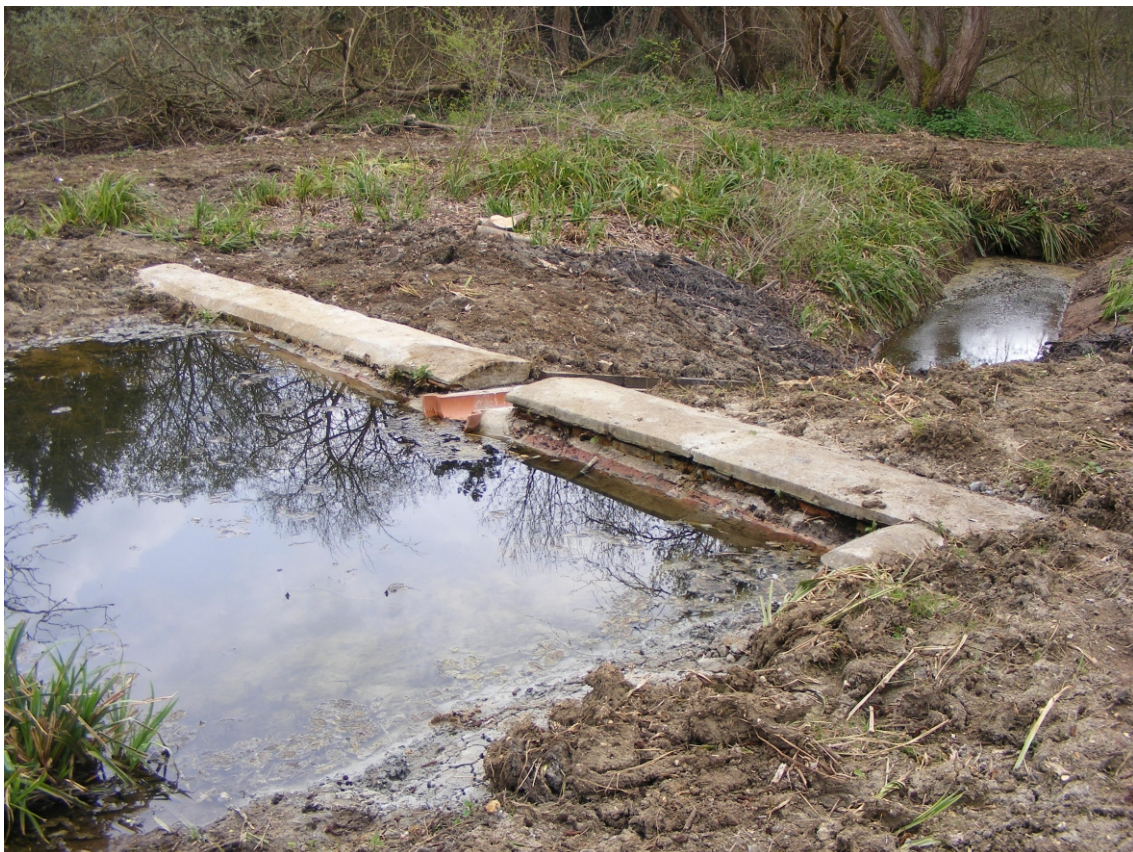
Plate 10: The dam [8] after remedial works, looking south-east
