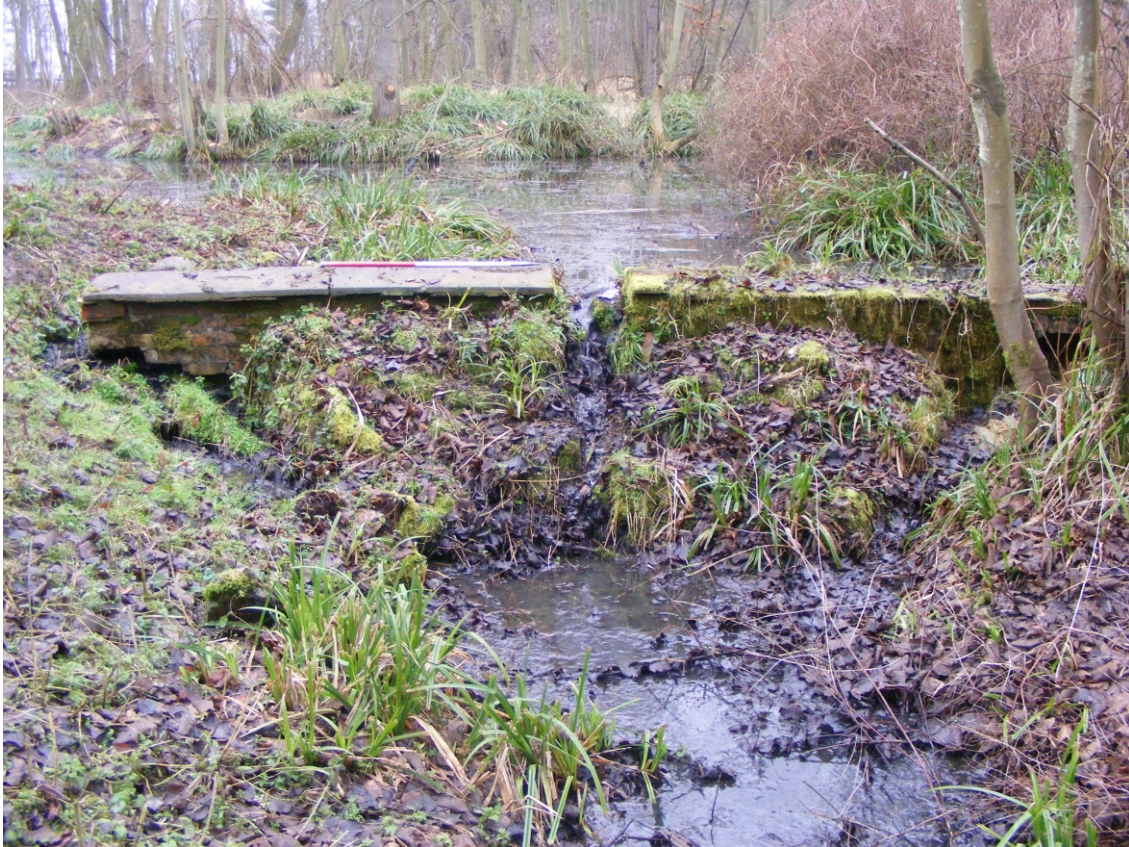
Plate 5: The dam [8] pre-works, looking north
