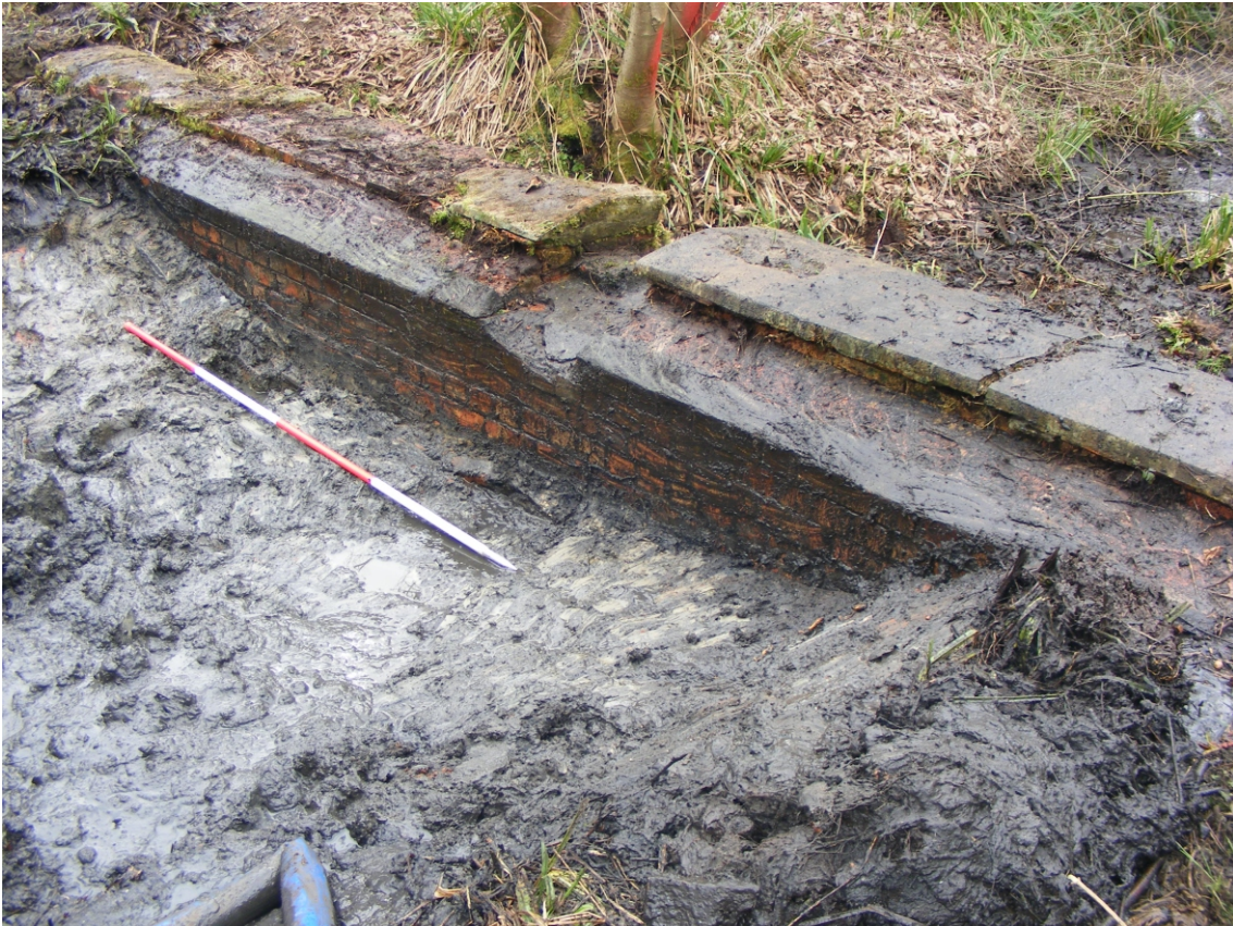
Plate 7: The dam[8] during remedial works, looking south-east
