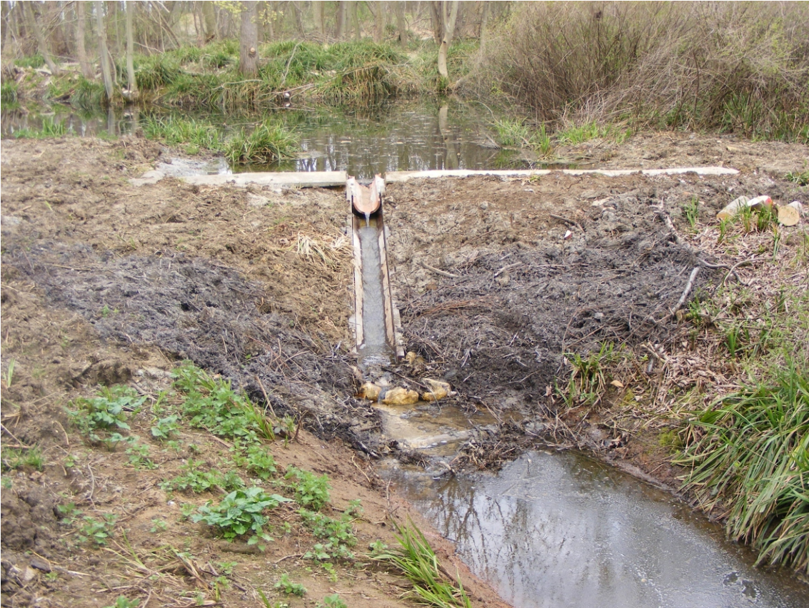
Plate 9: The dam [8] after remedial works, looking north-east
