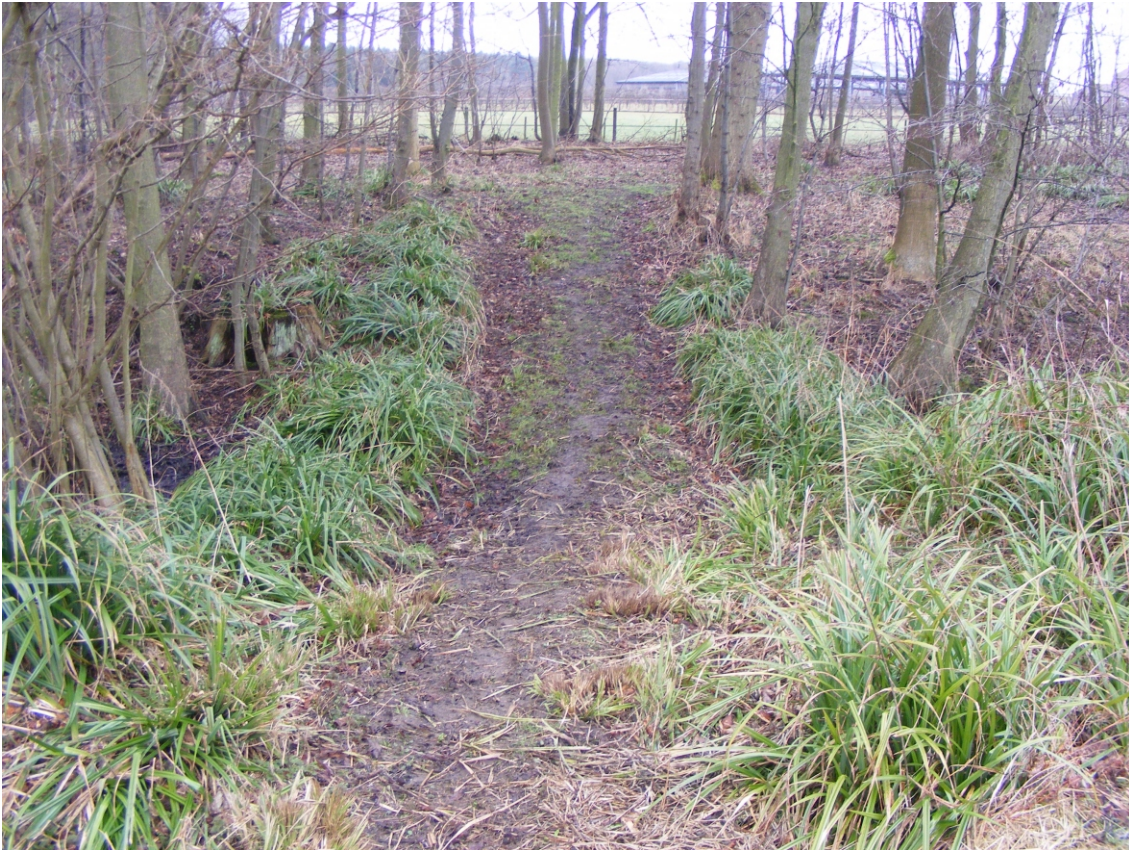
Plate 3: North moat arm/culvert [5], looking north pre-excitation
