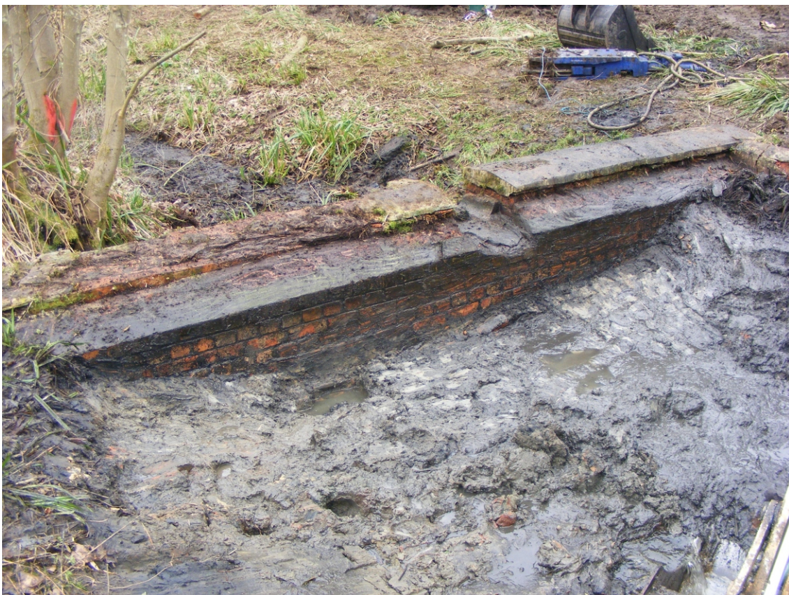
Plate 8: The dam [8] during remedial works, looking south-west
