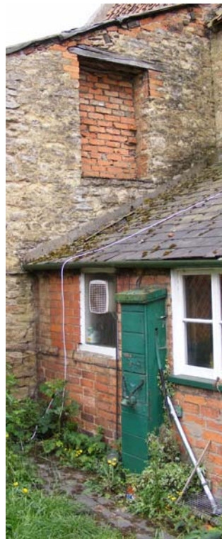
Fig 41: Blocked window in west wall of F8
