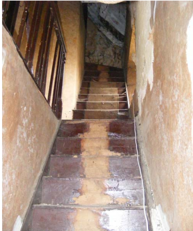
Fig 29: Stairs from G8 to first floor landing and bedrooms
