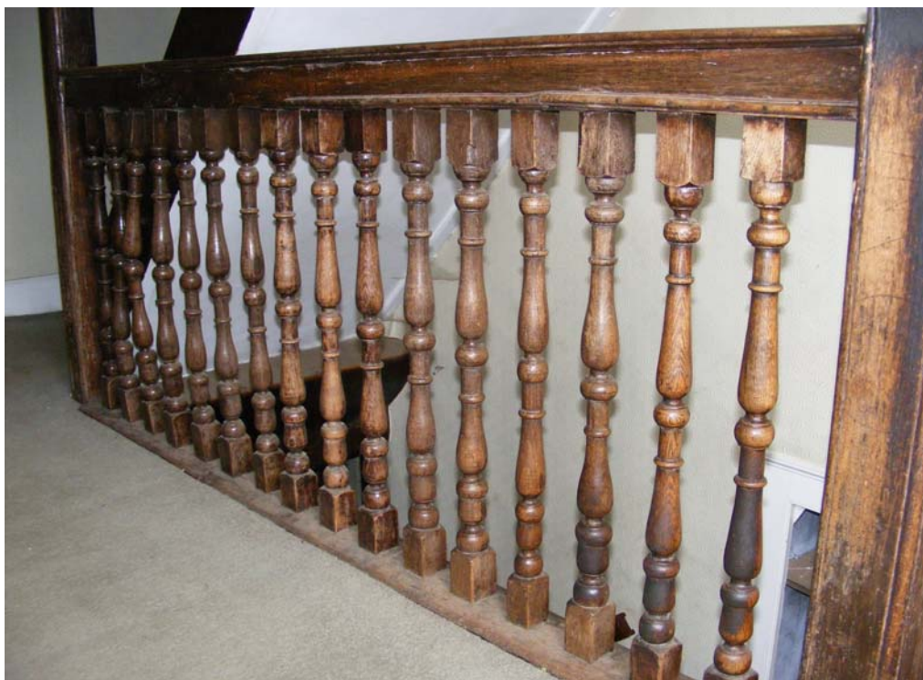
Fig 20: Hand rail and banister at first floor
