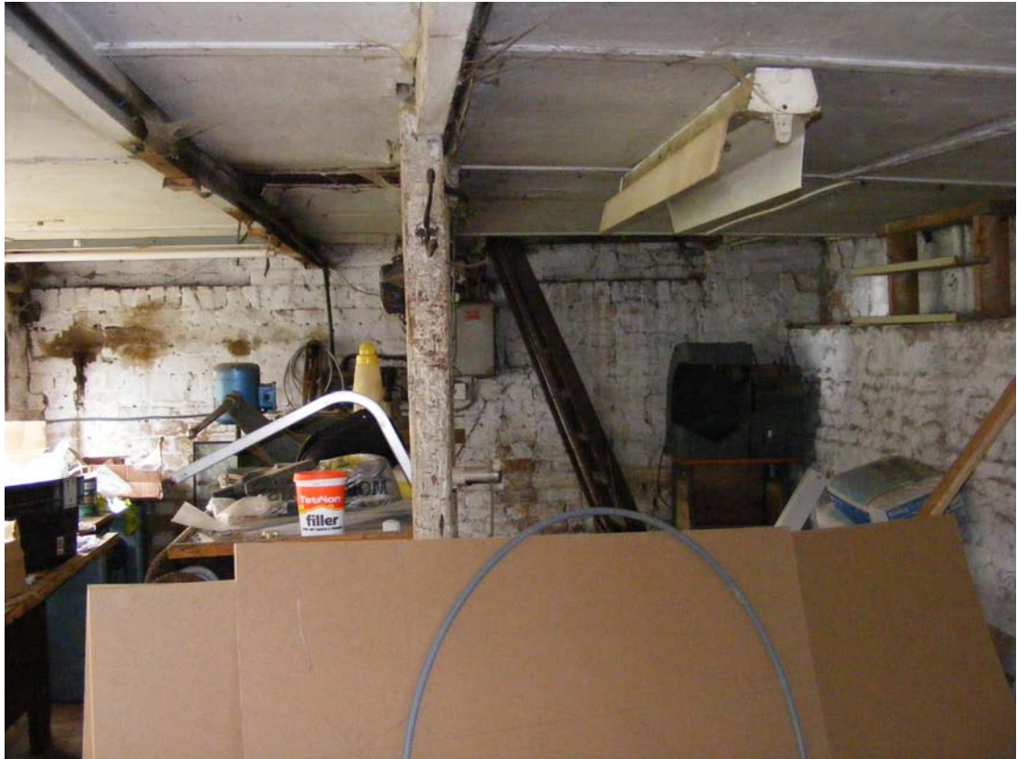
Fig 46: Cottage, ground floor interior
