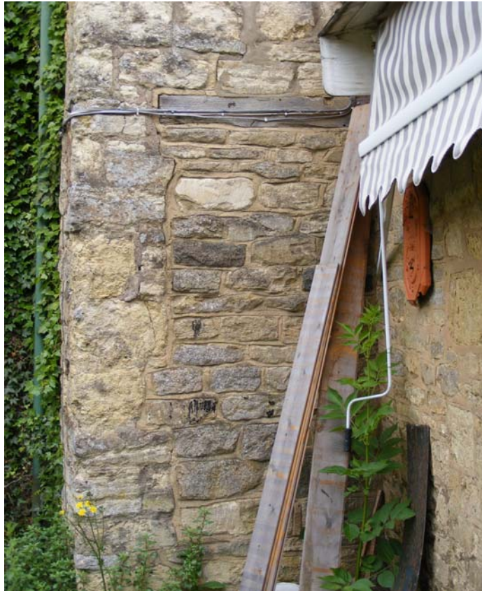
Fig 17: Blocked doorway in north wall of G4 (exterior)
