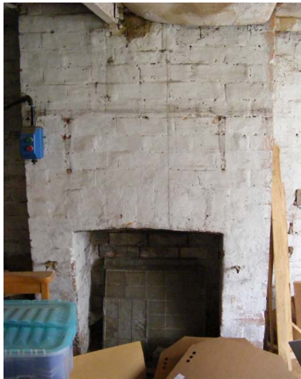
Fig 45: Cottage, ground floor interior, north end
