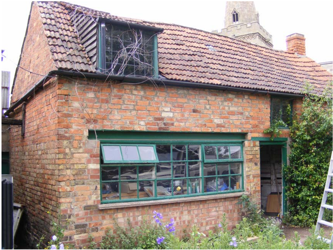
Fig 44: Cottage, east front, exterior
