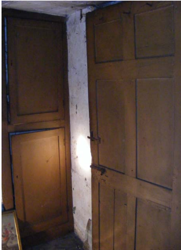
Fig 38: Room S6; note door paint scheme on woodwork
