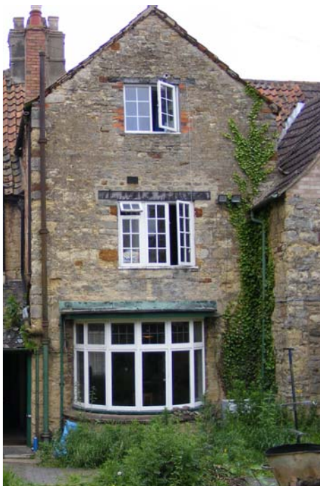
Fig 18: Extension built for the current staircase
