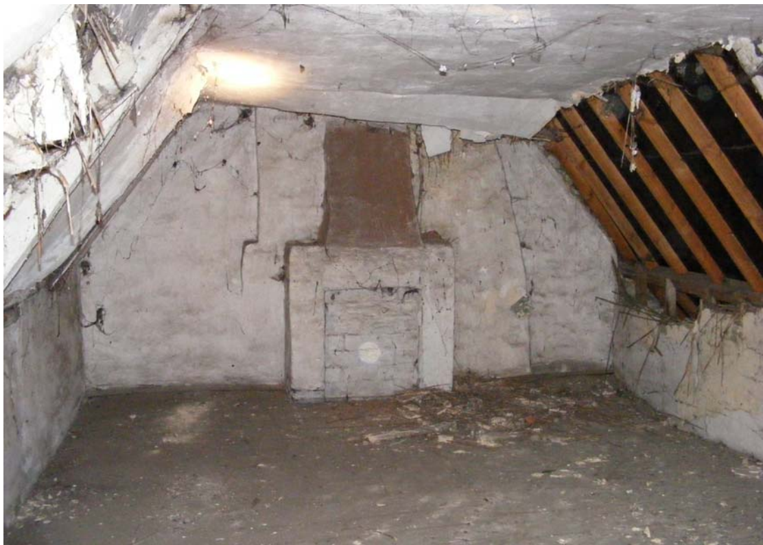
Fig 39: Room S7; note dormer removed at front (right)
