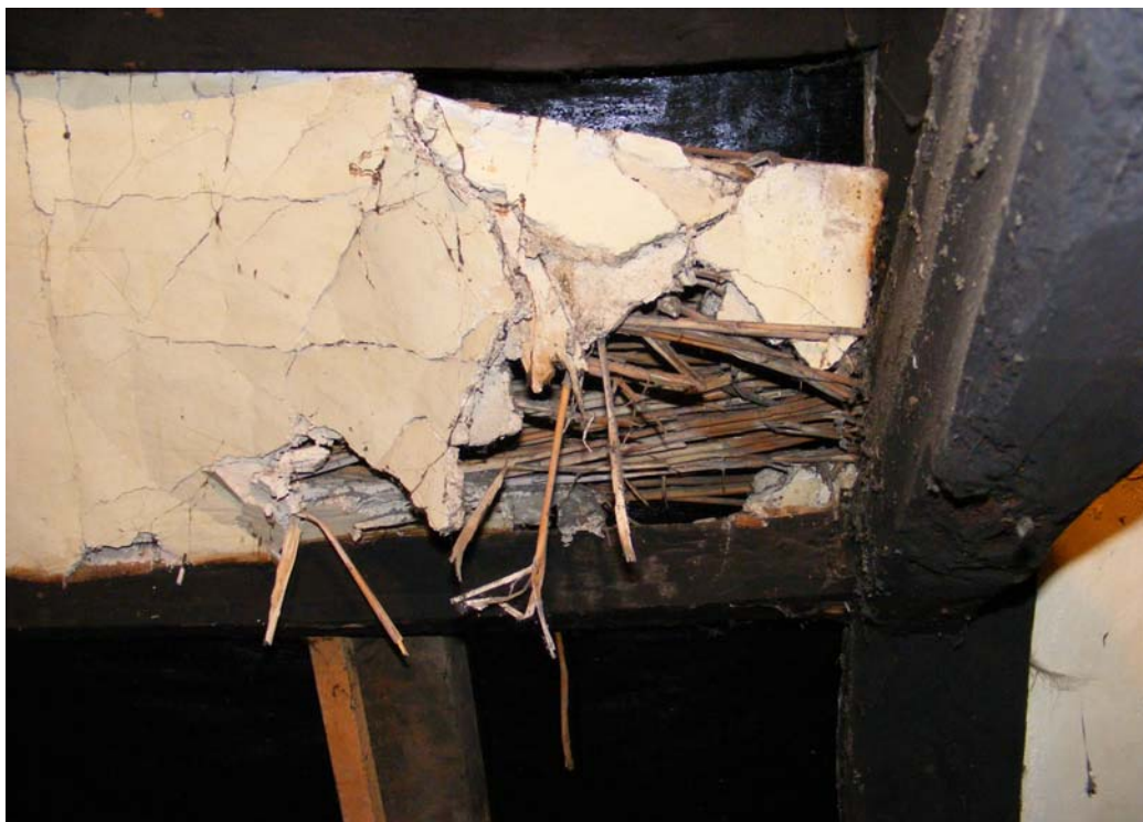
Fig 12: Reed plaster of second floor
