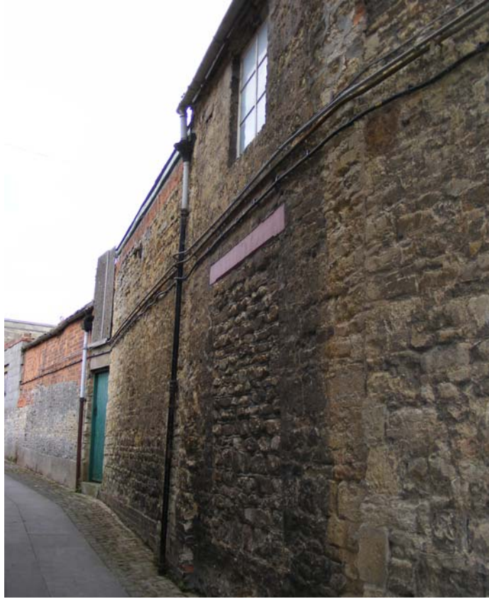
Fig 15: Blocked window in west wall of G4 (exterior)
