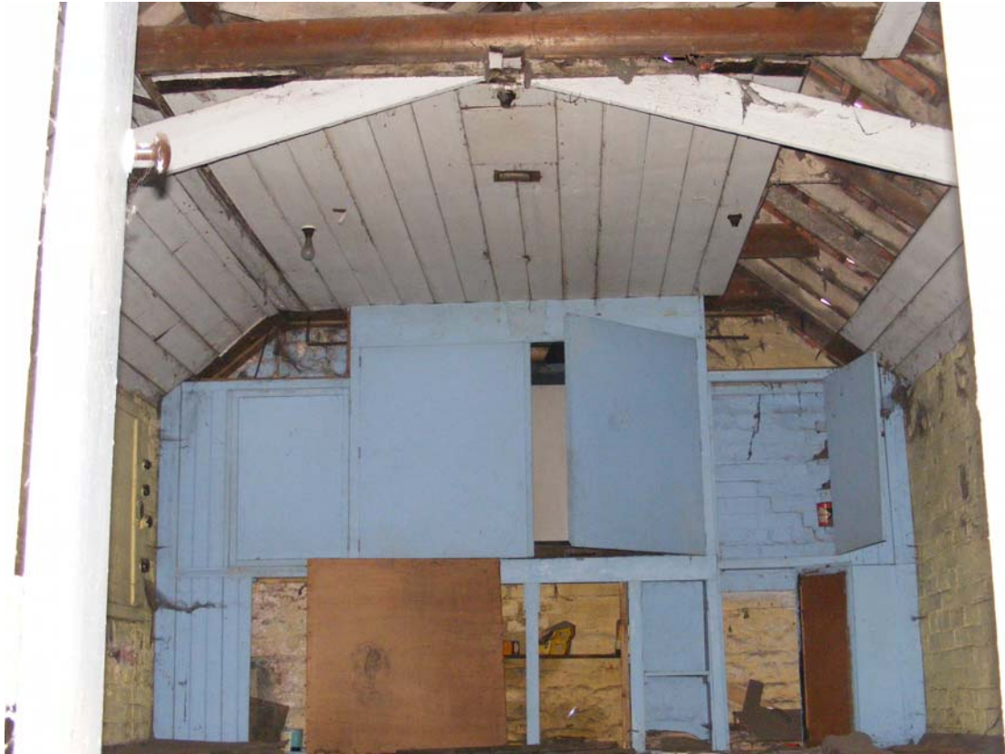
Fig 42: Room F9, remotely photographed from stair in G12
