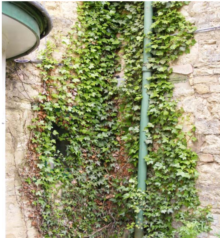
Fig 16: Blocked window in east wall of G4 (exterior)
