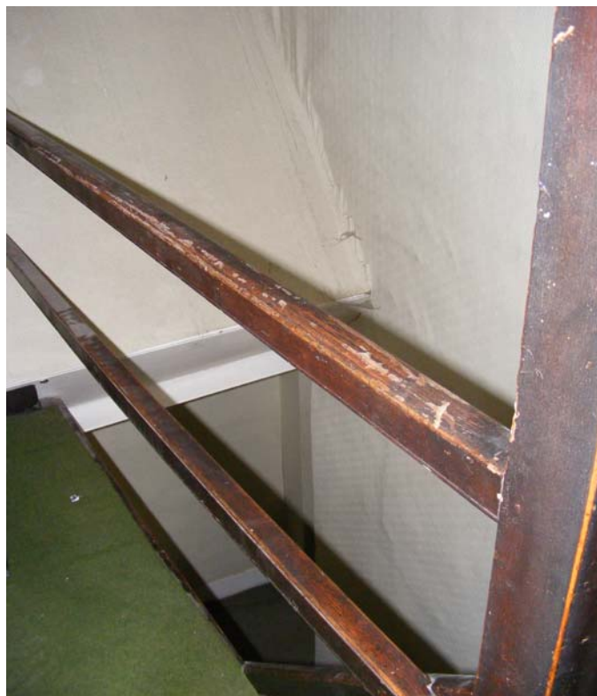
Fig 22: Landing at second floor, simple handrail
