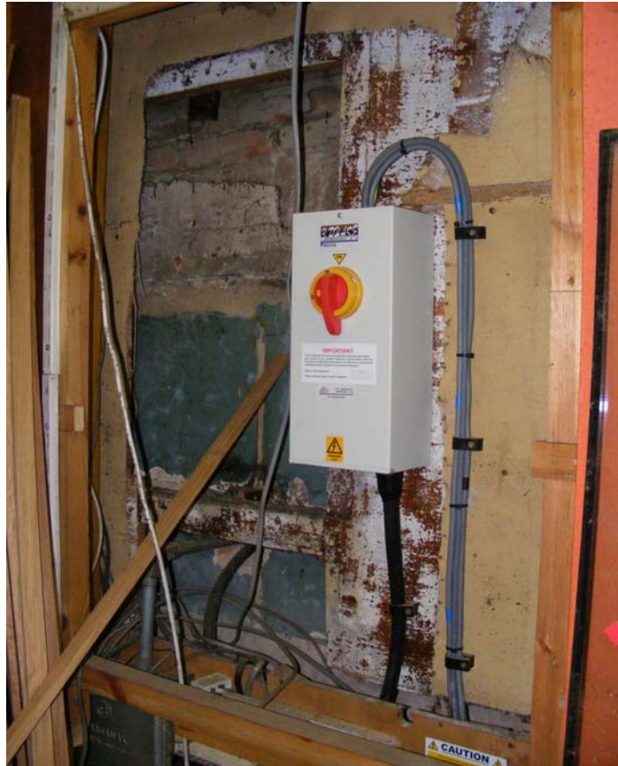
Fig 11: Former décor in west wall of G2
