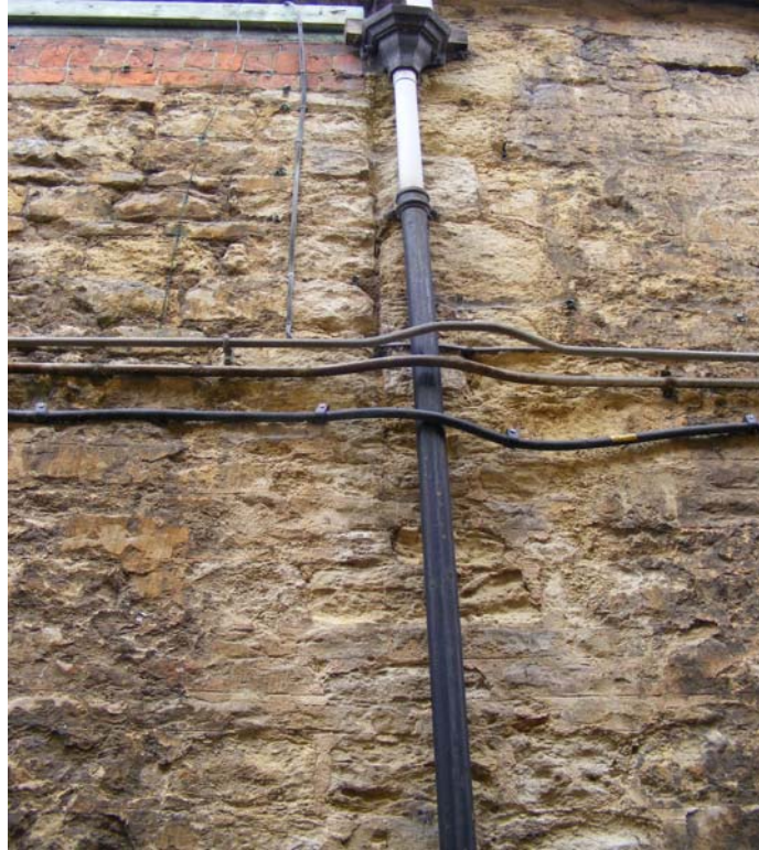
Fig 23: Butt joint between G4 and G5, viewed from The Slabs
