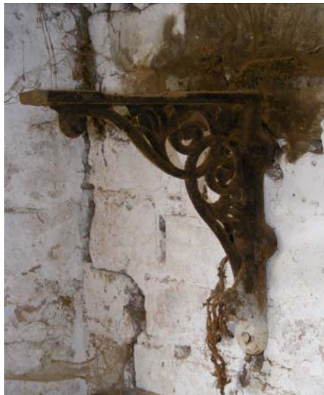
Fig 47: Cottage, cast iron shelf bracket
