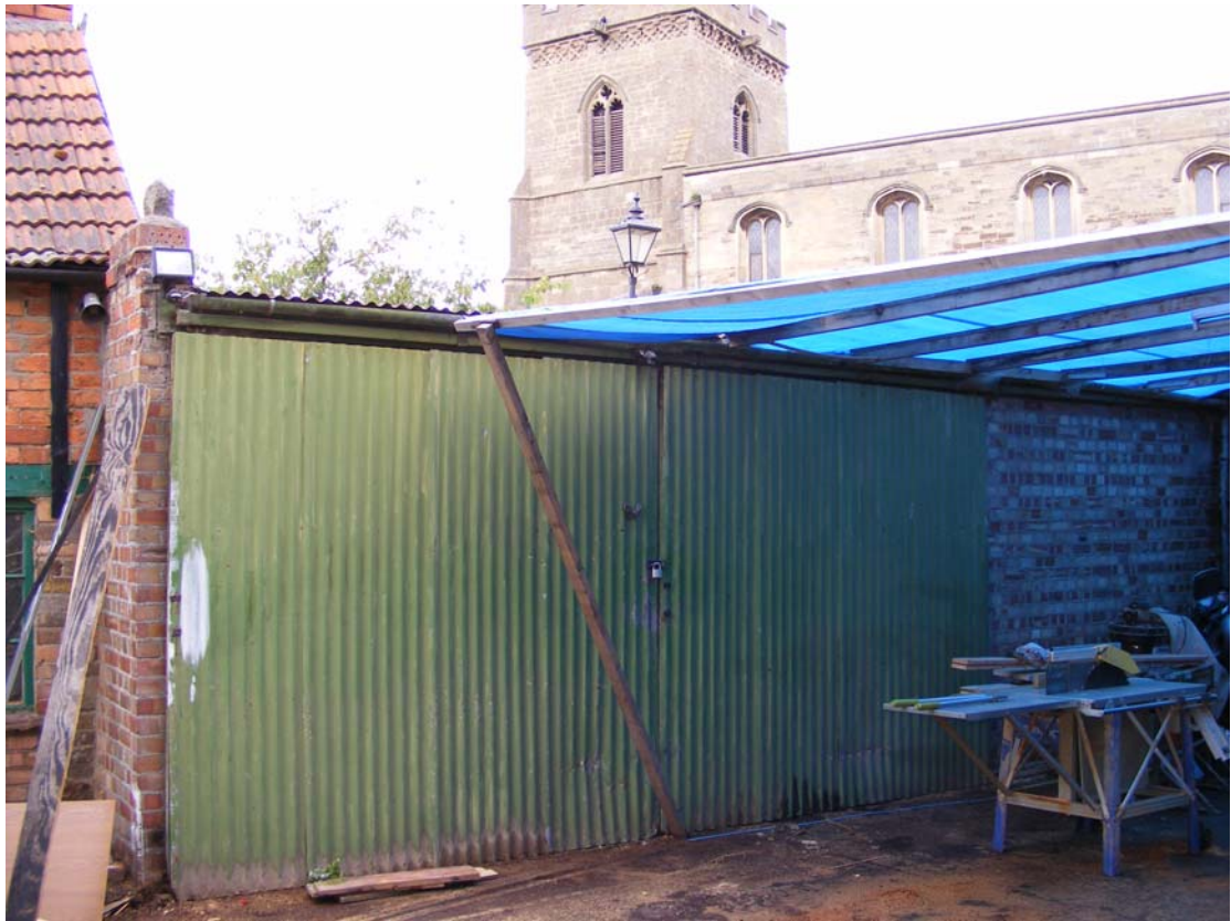
Fig 50: Shed added to cottage at north end
