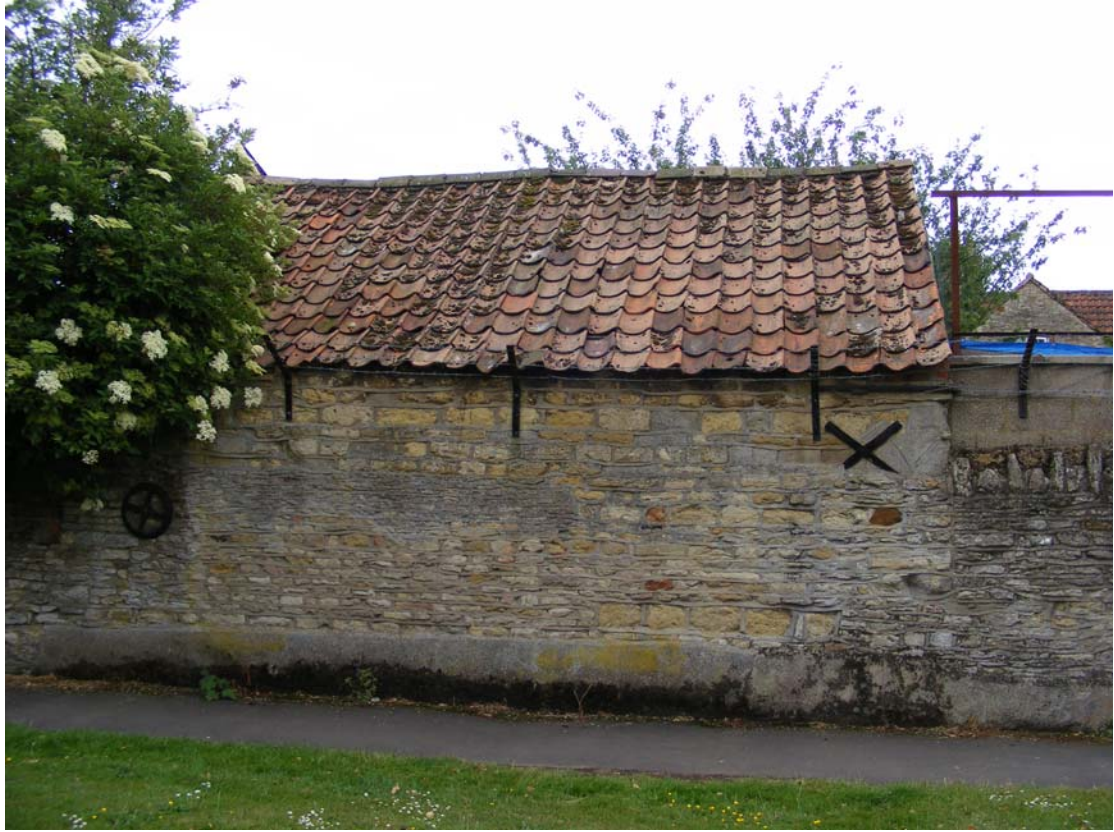
Fig 52: Carriage House rear, facing churchyard
