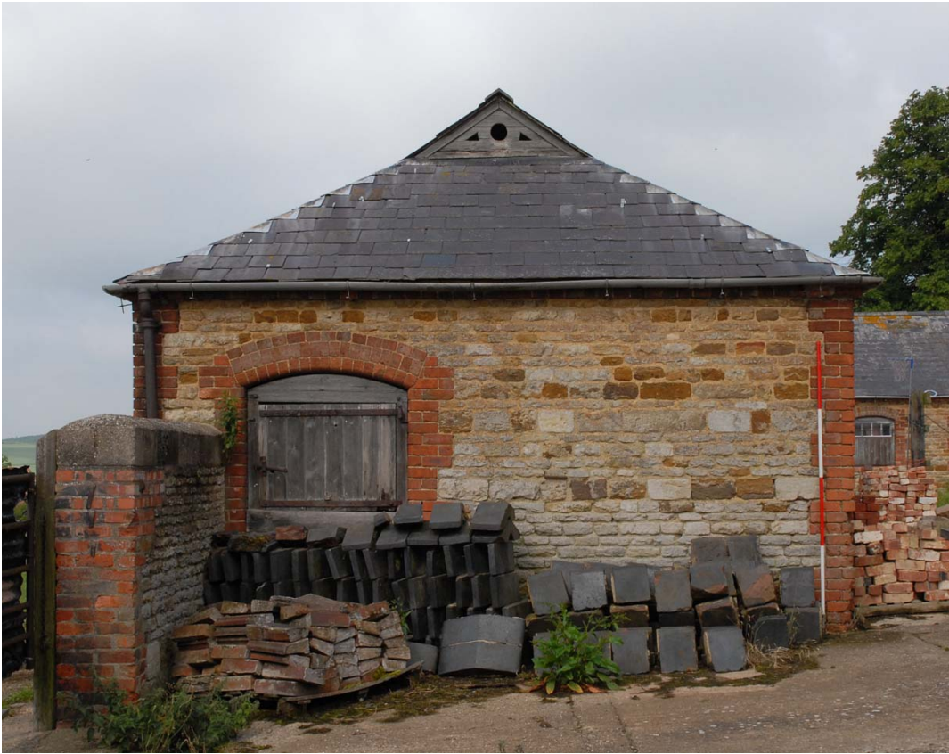
Plate 14: Building 2 east elevation
