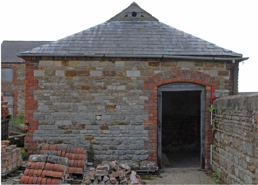
Plate 15: Building 2 west elevation
