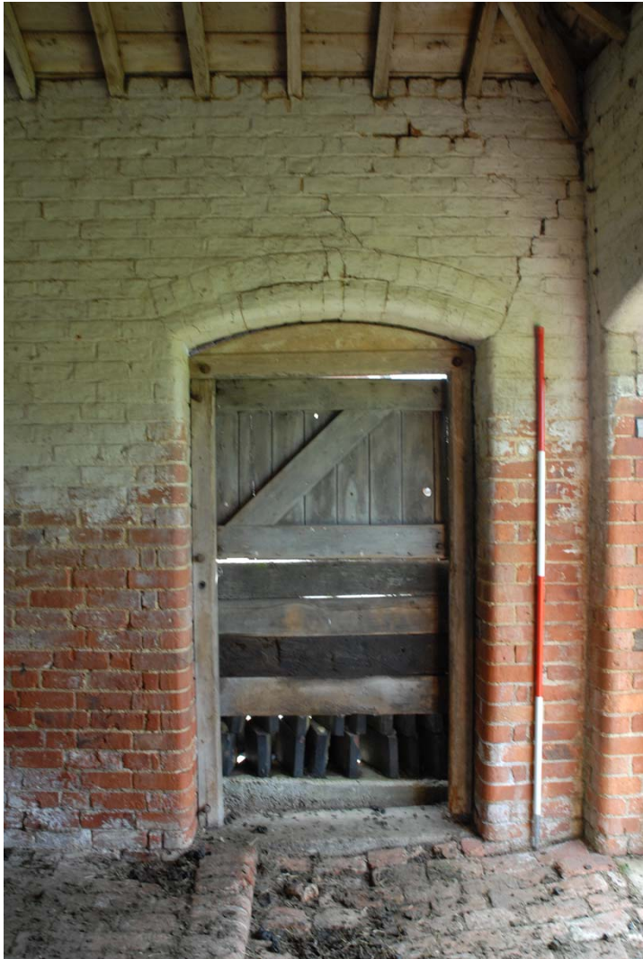
Plate 13: Building 2 door detail
