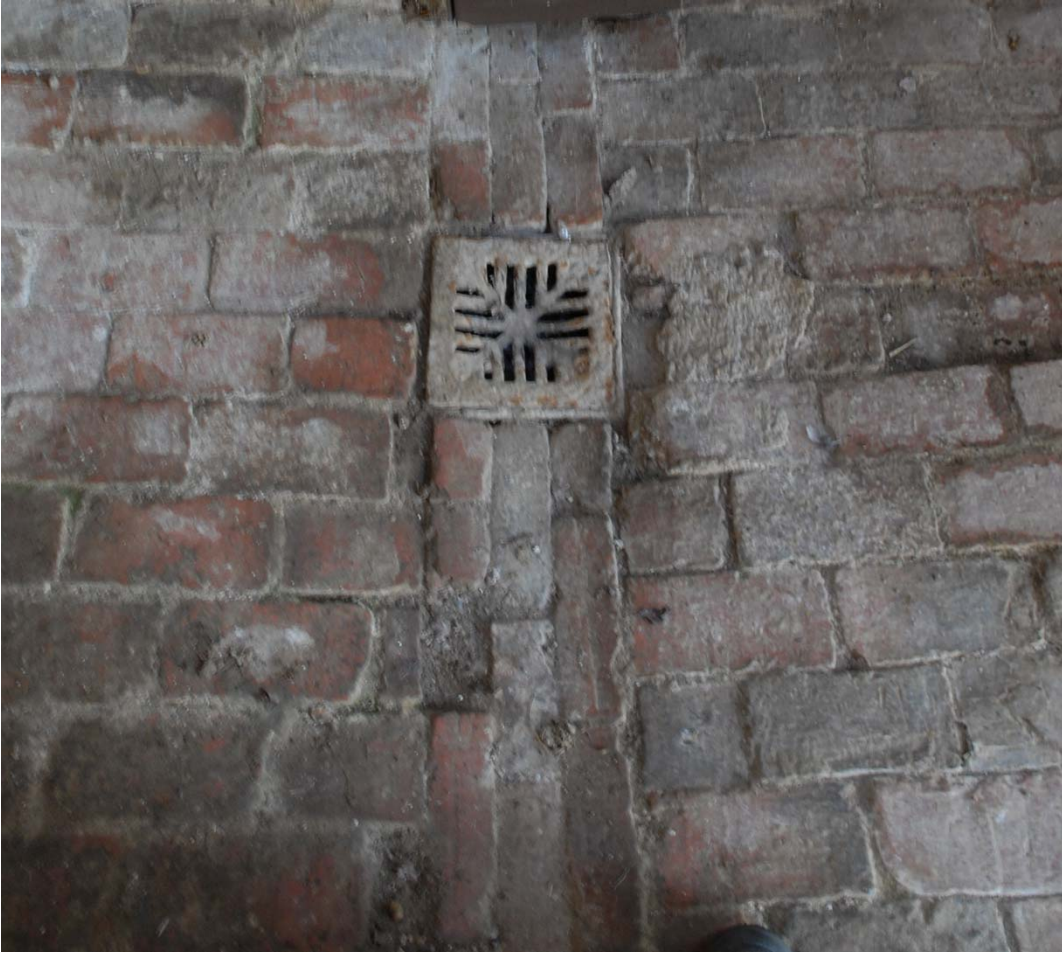
Plate 9: Building 1 floor detail
