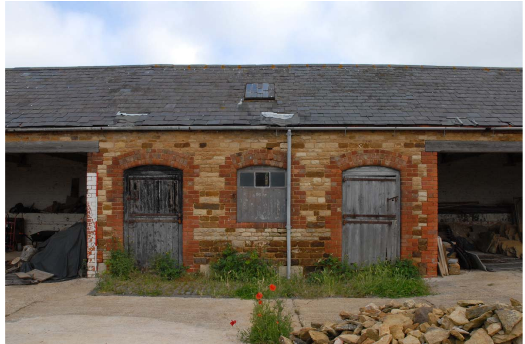
Plate 4: Manor Farm Building 1 south elevation
