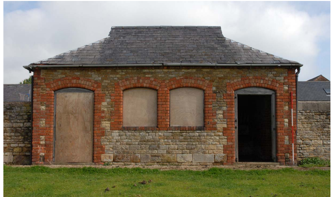
Plate 16: Building 2 south elevation
