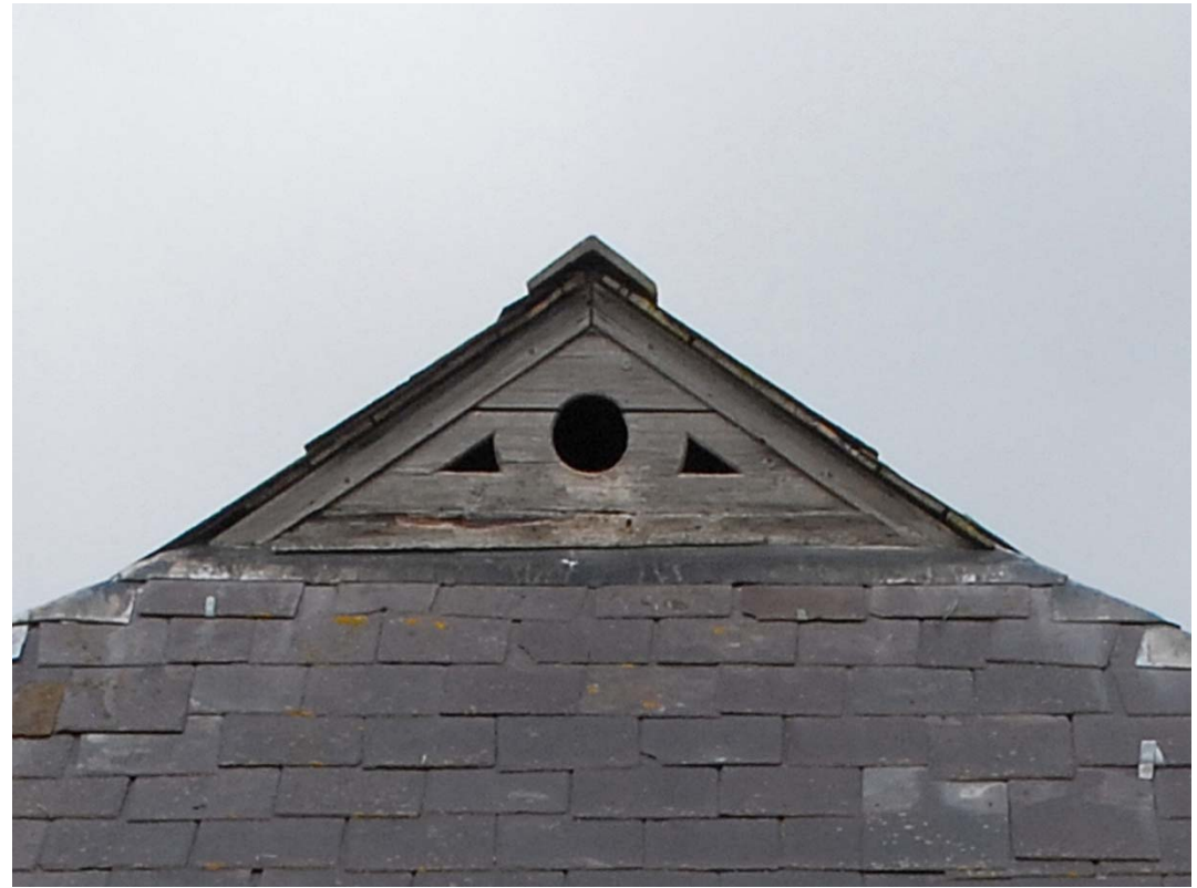
Plate 18: Building 2 pierced ventilation detail
