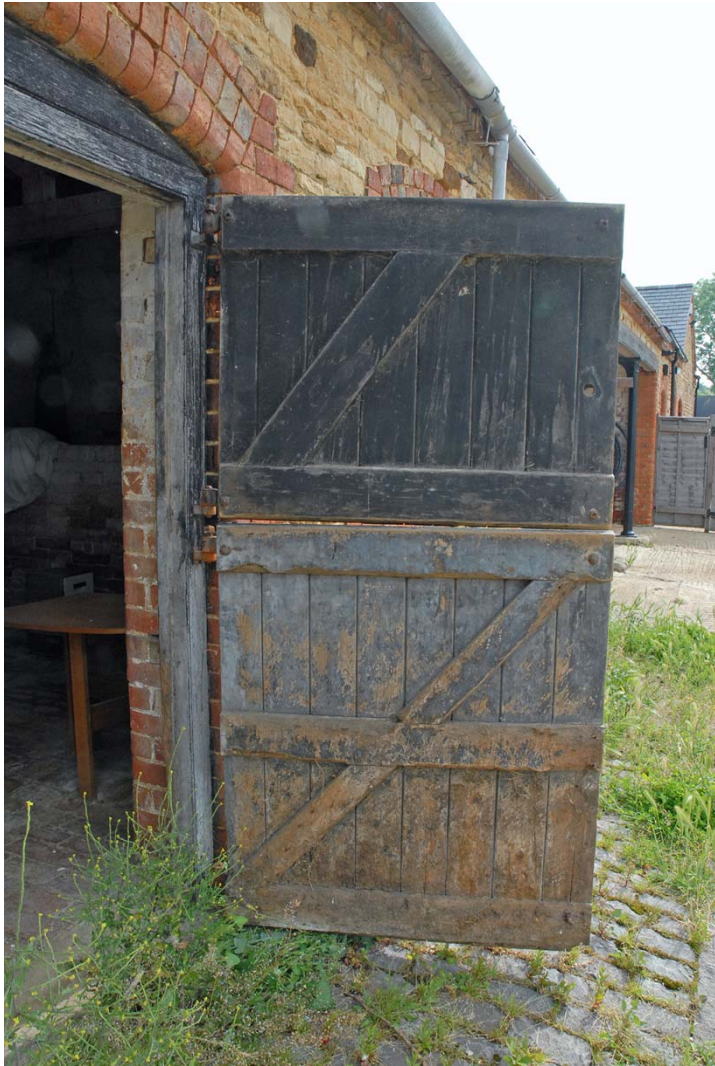
Plate 5: Building 1 stable door
