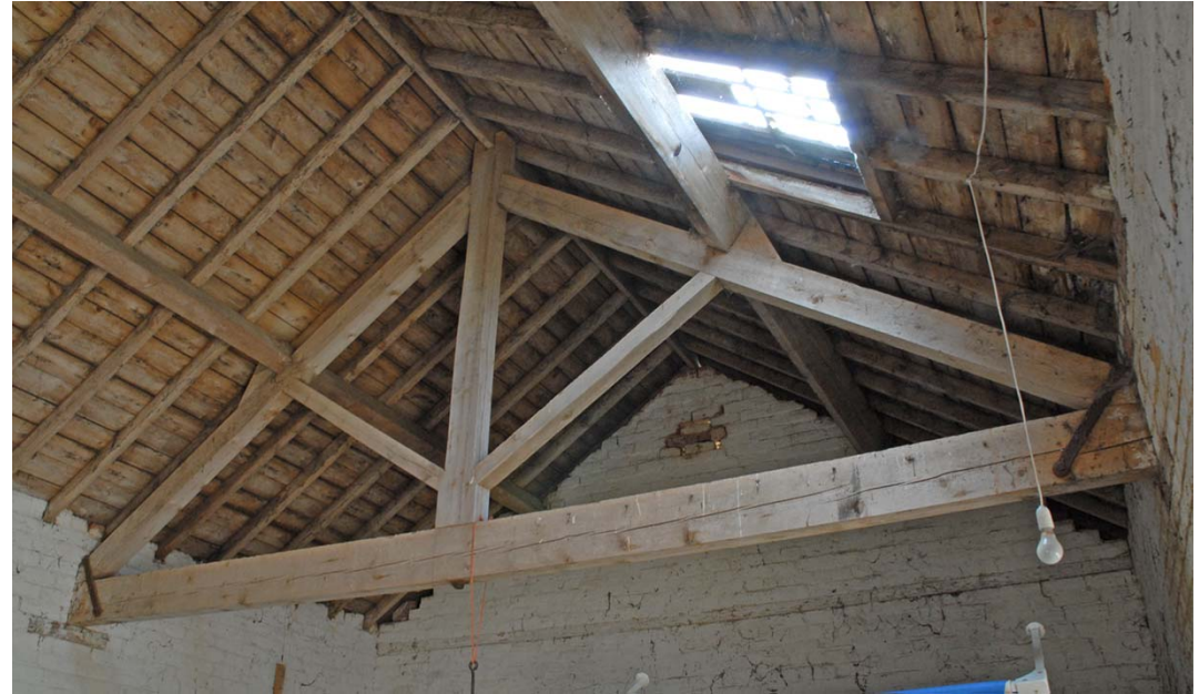
Plate 10: Building 1 kingpost truss detail
