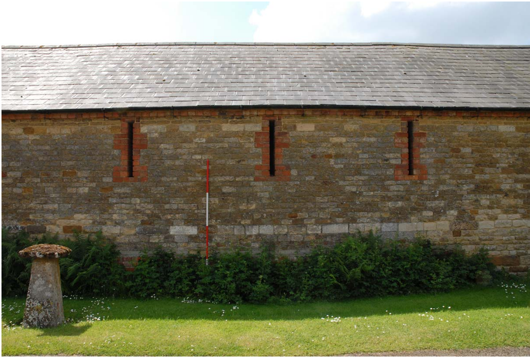
Plate 7: Building 1 north elevation
