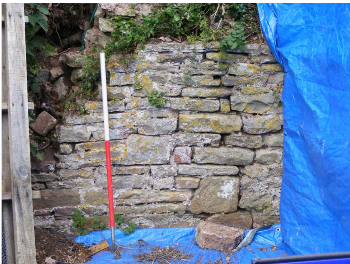
Plates 7 and 8: Showing possible joggle joints perhaps derived from the removed of quoins at the infilling of a gateway at the centre of the south-western wall
