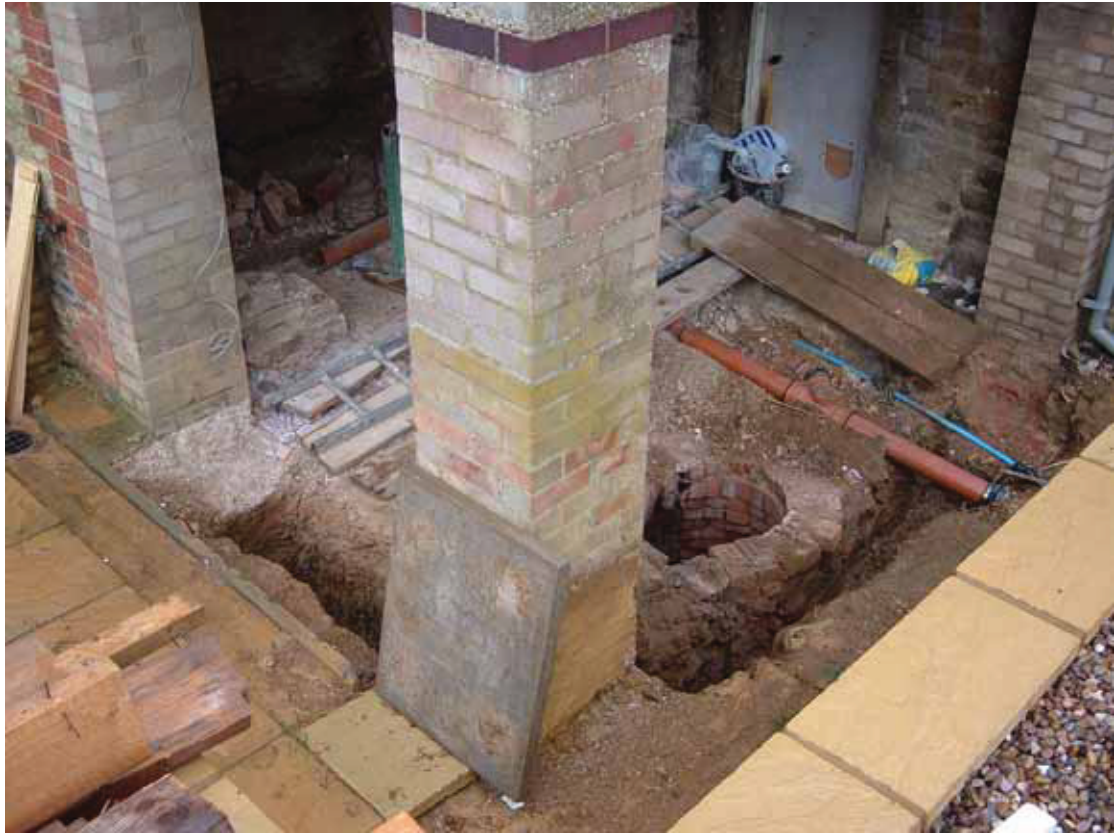
Kitchen foundation trenches, looking east-north-east Fig 5
