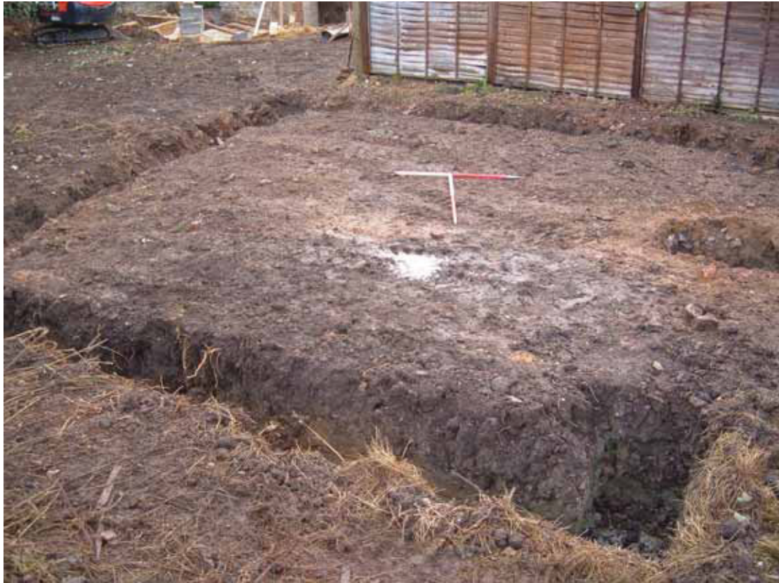
Garage foundation trenches, looking north-east Fig 3
