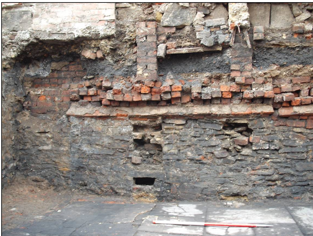
The stone cellar wall of No 8, Court 9, looking south, showing scars of the removed brick piers beneath the ground floor fireplace, and the springing of the brick vault, with the removed stairs to the left Fig 30
