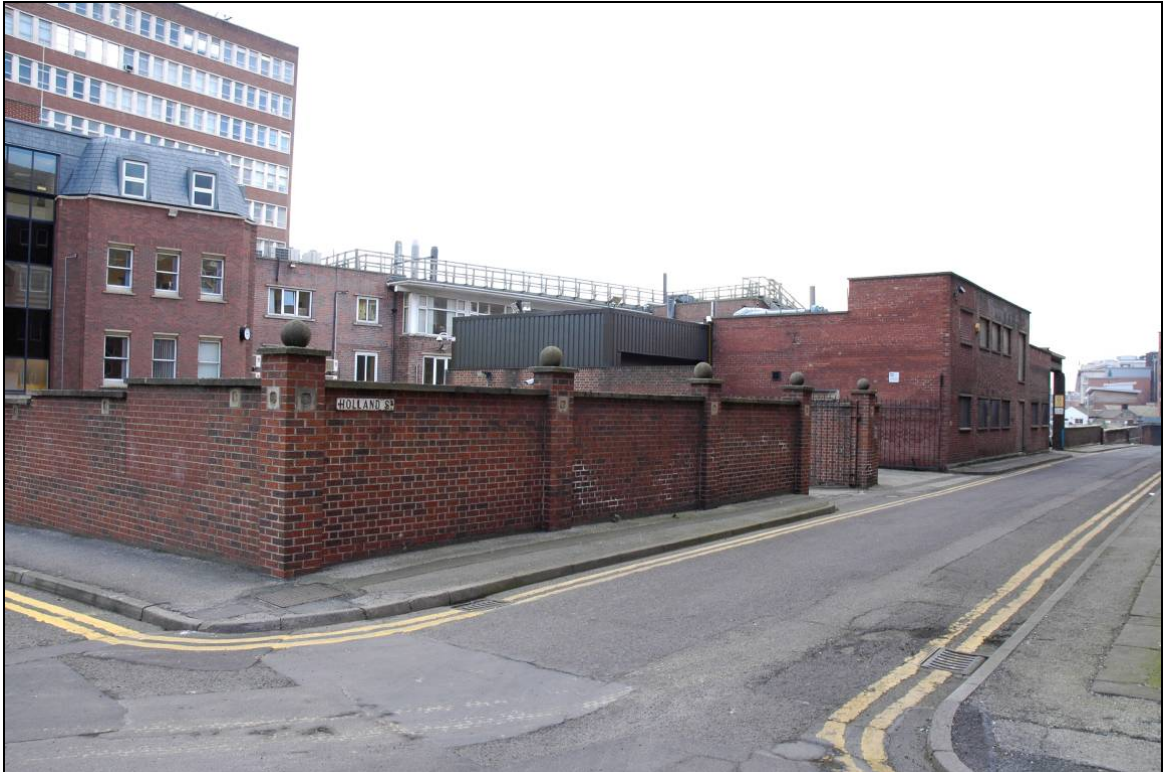
View of site prior to the demolition of the Assay Office, looking north-east along Holland Street Fig 8
