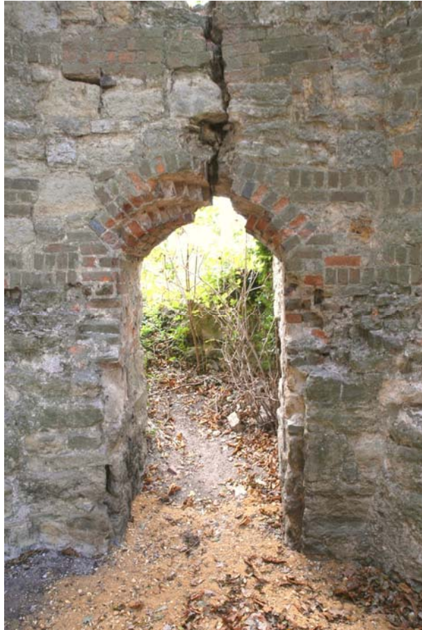
Segmental brick arch of door Fig 20
