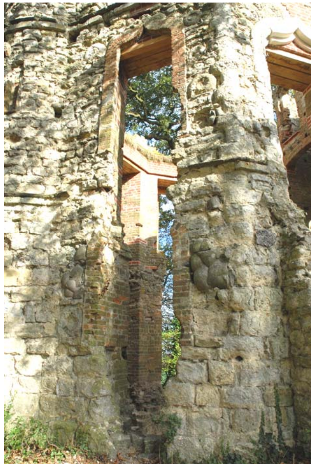
Brick detailing around window on south-west wall Fig 9
