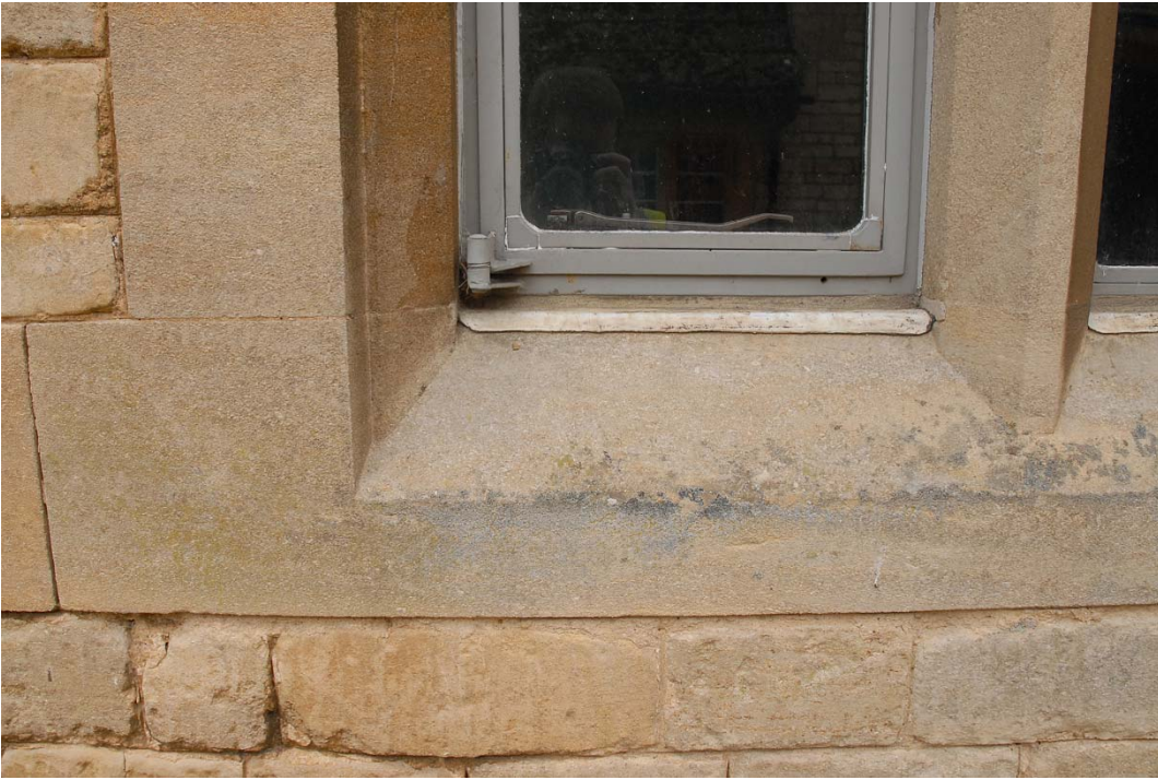
Fig 8: Lead flashing under window
