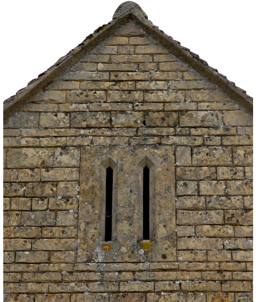
Fig 9: Vents on gable end
