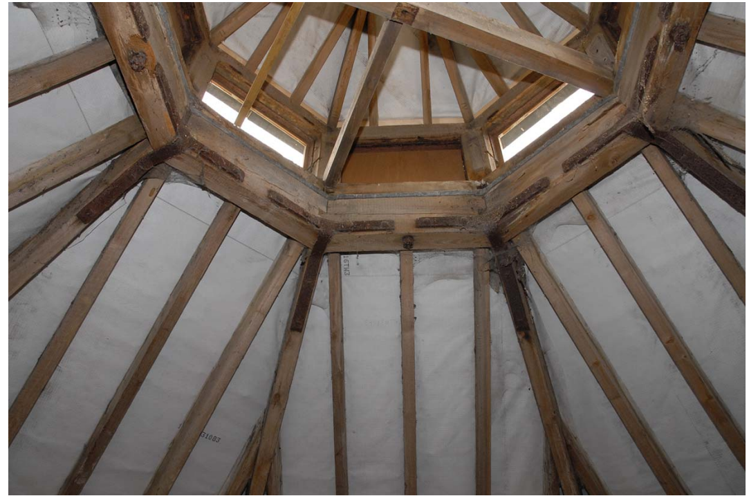
Fig 21: Lantern roof in dovecot
