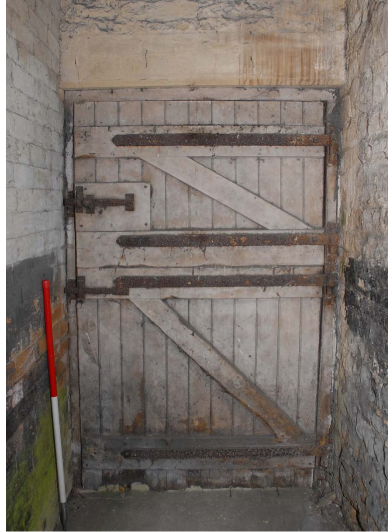
Fig 29: Ledged and braced door in Room 6
