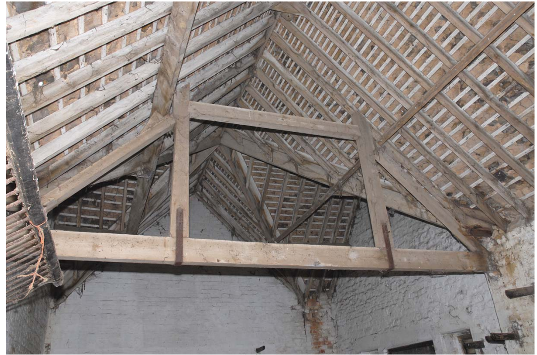
Fig 27: Queen strut truss in Room 7
