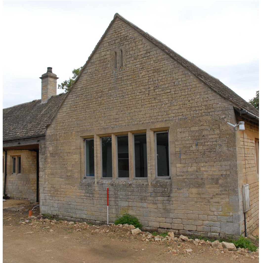
Fig 5: Gable west range
