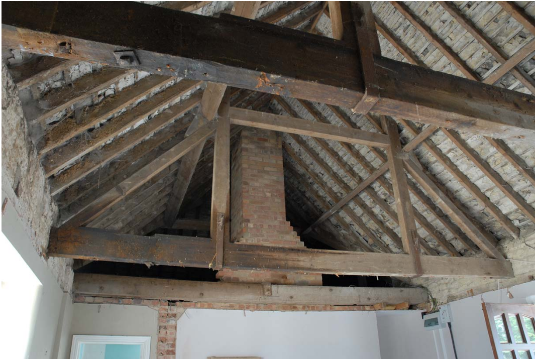
Fig 14: Room 2 queen strut truss
