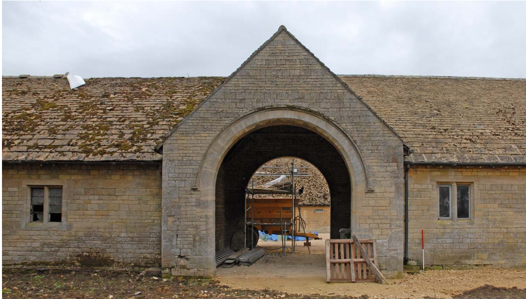
Fig 26: North range north facing elevation of arch
