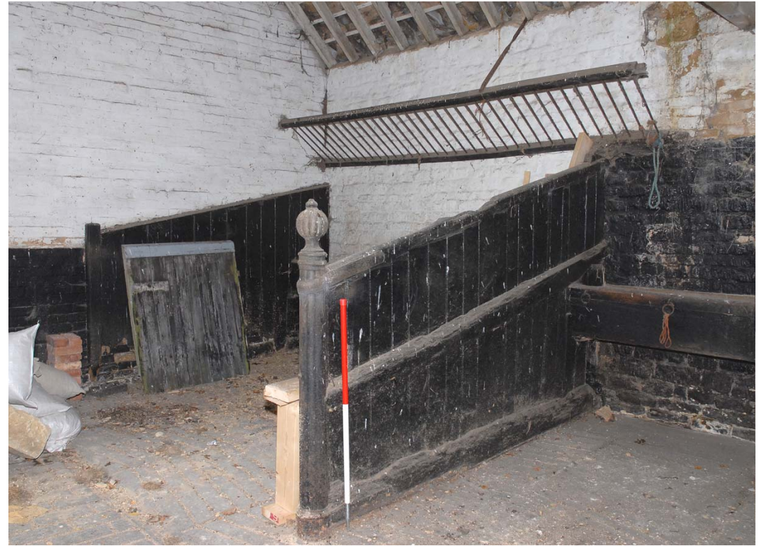
Fig 31: Stalls in Room 7
