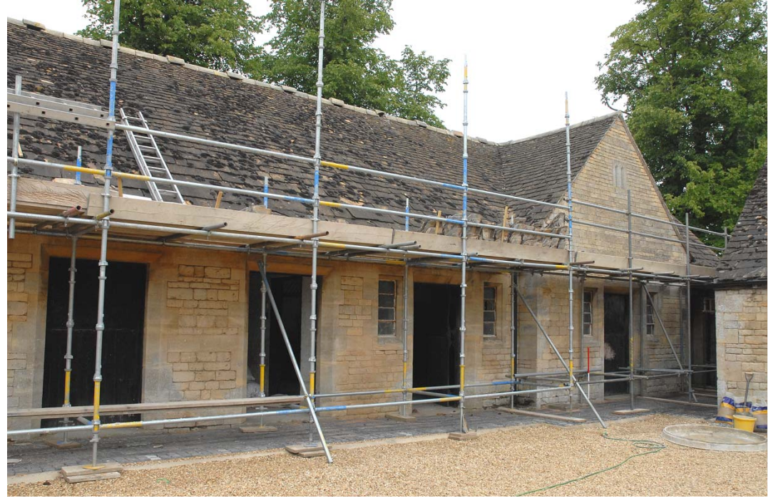
Fig 25: North range south facing elevation
