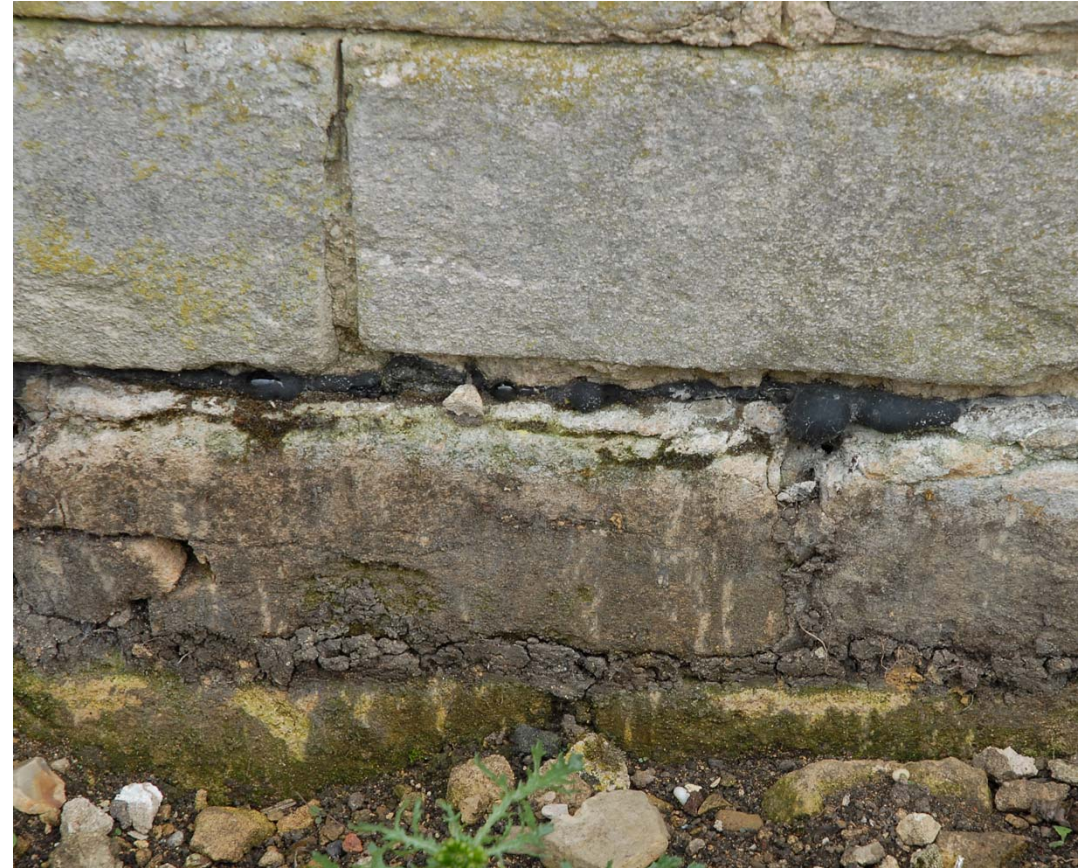
Fig 7: Bitumen damp course
