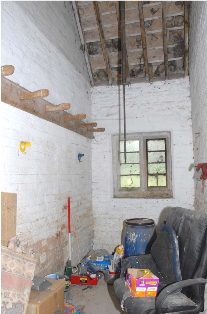
Fig 30: Room 7a general view of tack room
