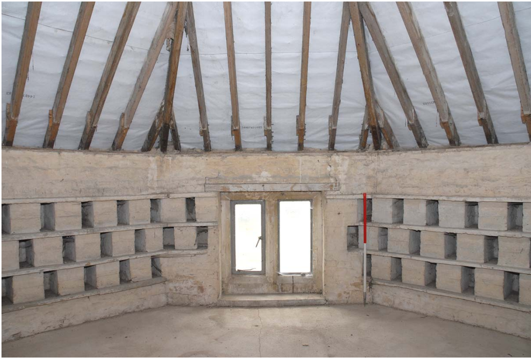
Fig 20: Room 4a dovecot interior
