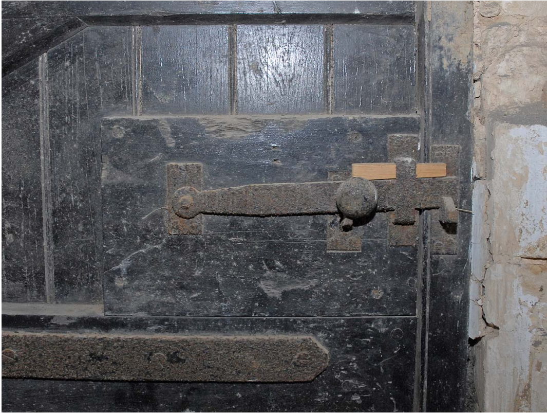
Fig 24: Room 5 door latch detail
