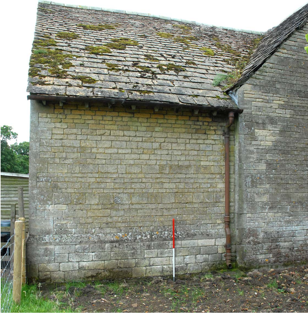
Fig 34: North facing elevation of north range showing the extension
