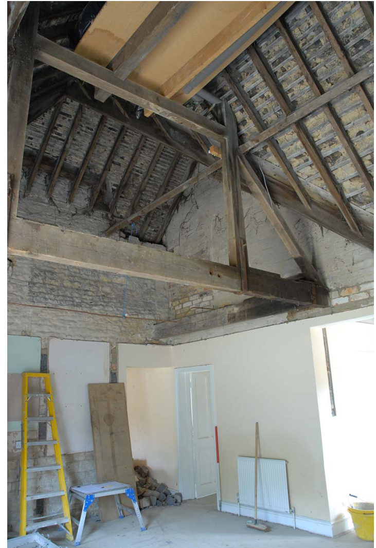
Fig 17: Room 3 roof detail
