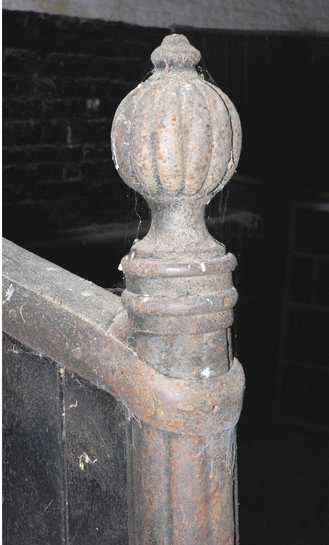
Fig 32: Detail of cast iron stall post
