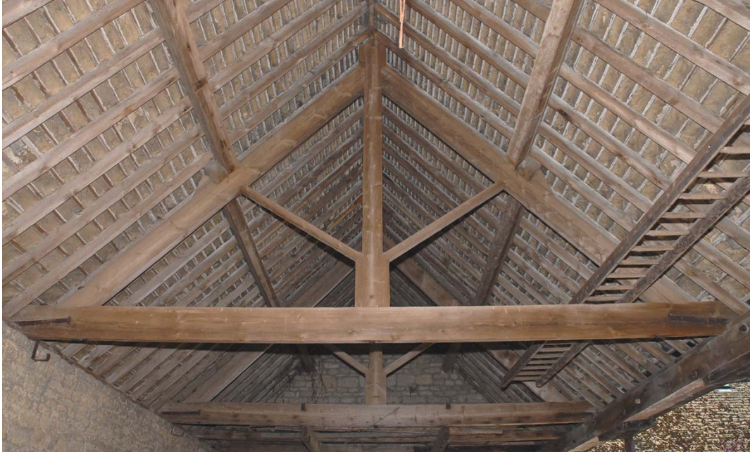
Fig 36: King post truss in the open stock/cart shed
