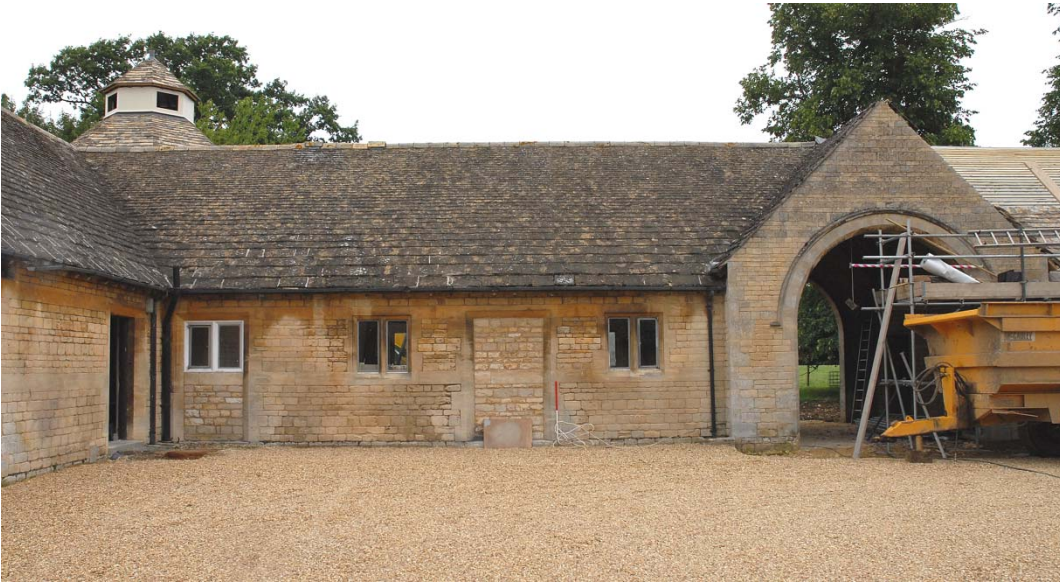
Fig 22: North range south facing elevation
