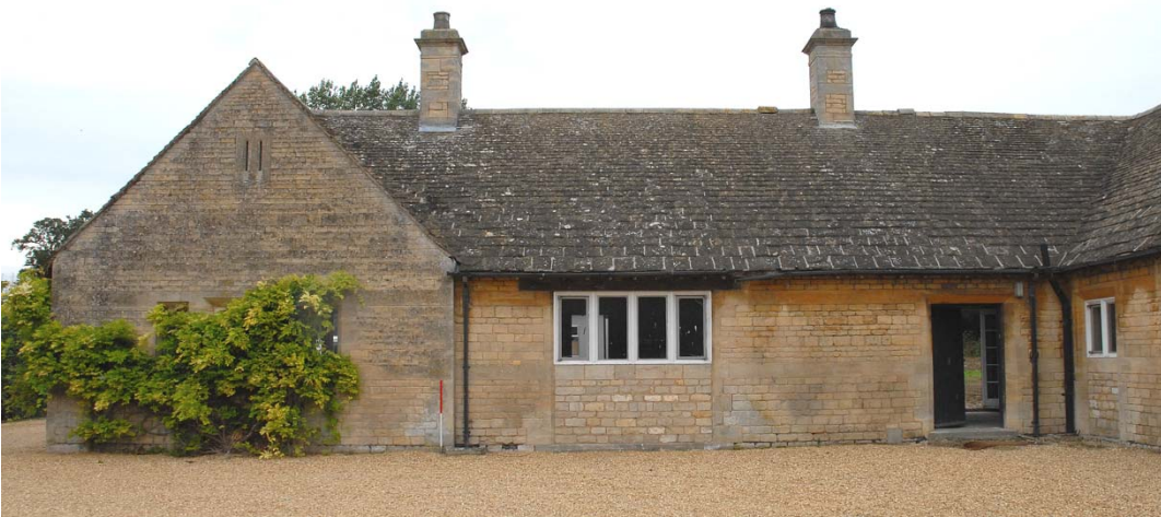
Fig 12: West range east facing elevation
