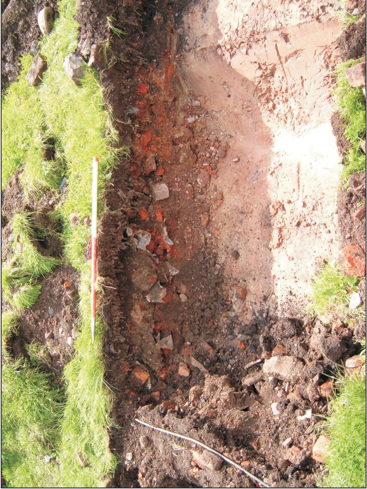
Trench1, made up ground and cable, looking south-east Fig 9
