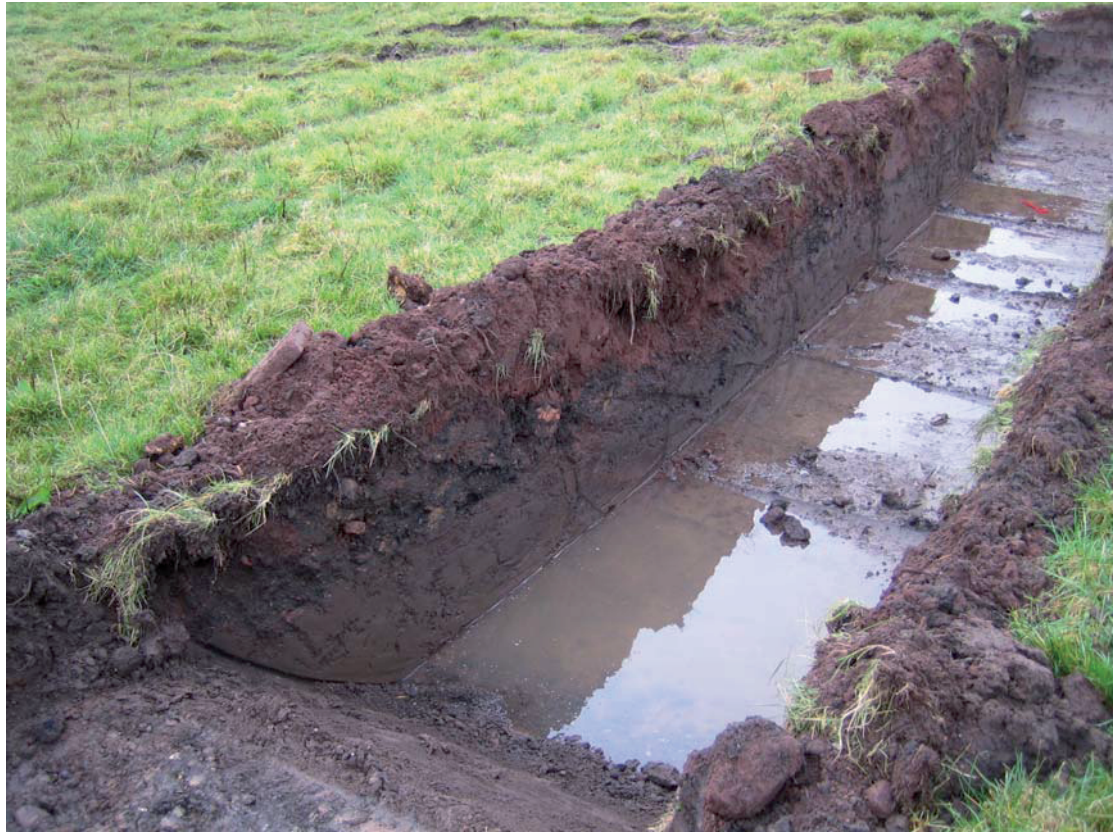
Fig 10: Trench 7 'pond', looking south-east
