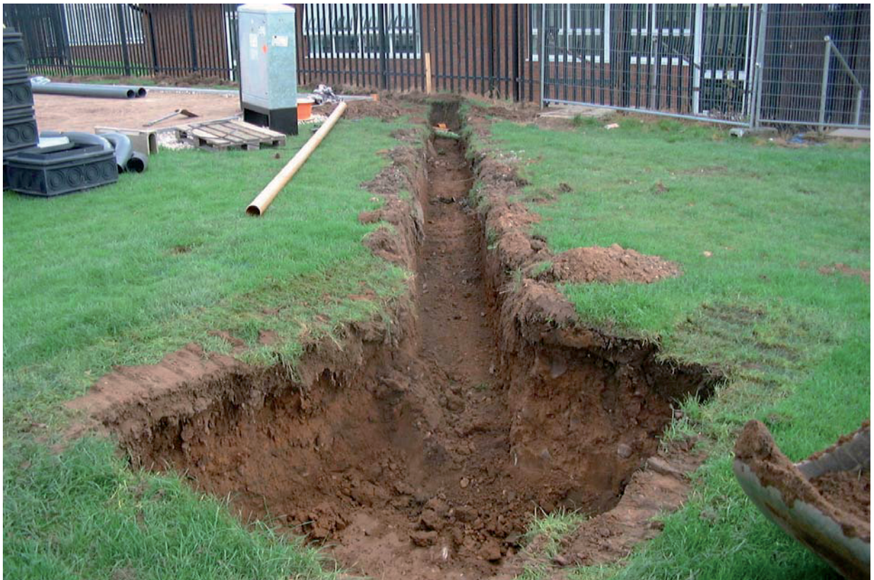
Fig 4: The soak-away during excavation
