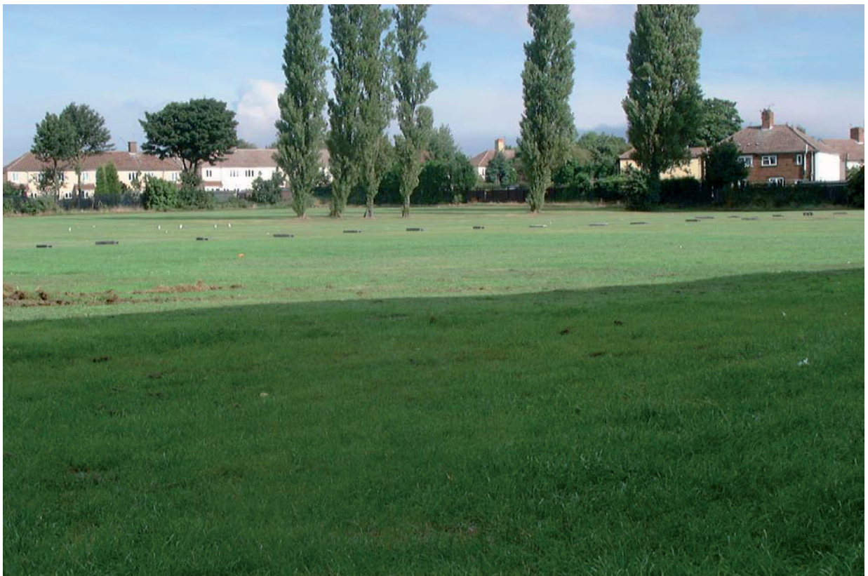
Fig 2: General view of development area at the start of groundworks
