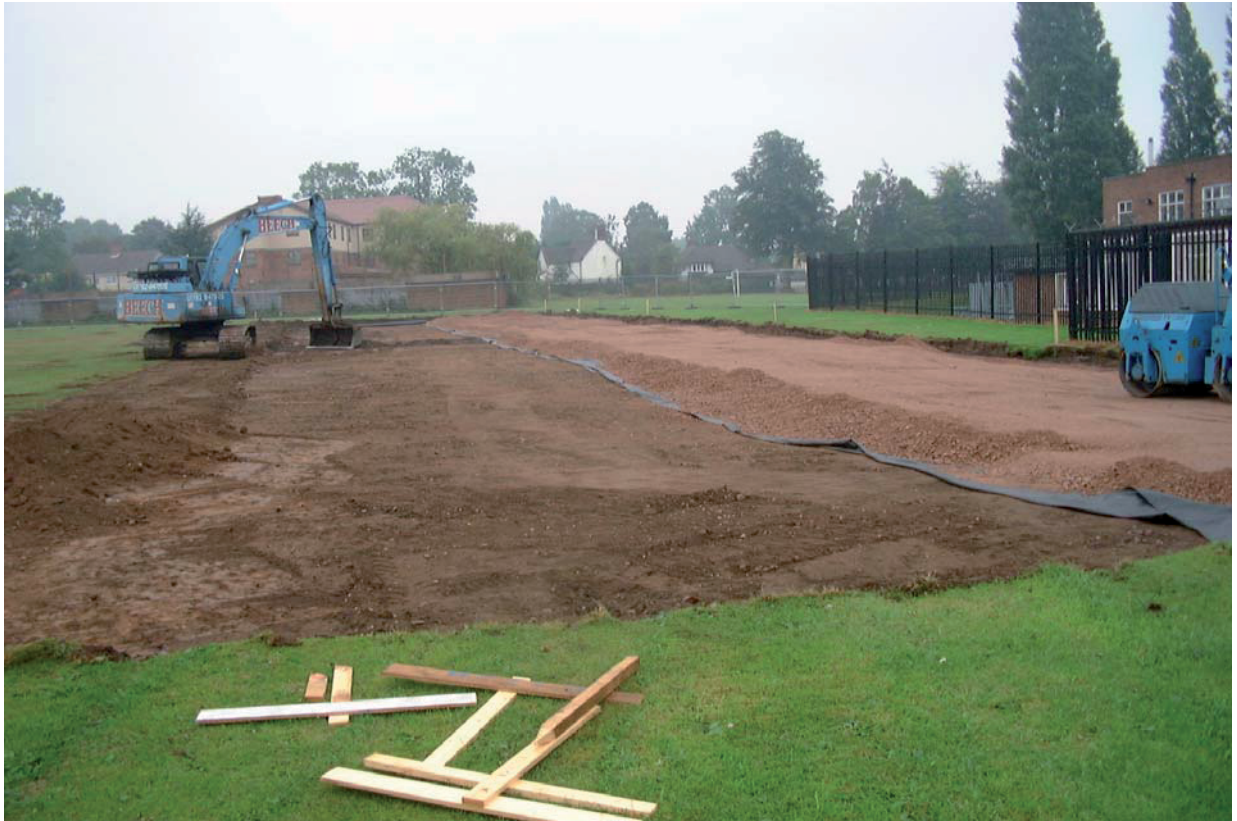
Fig 3: Groundworks in progress
