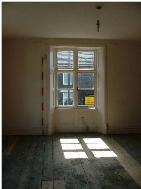
Plate 56: Detail of window in east wall, first floor (Scale = 2m)
