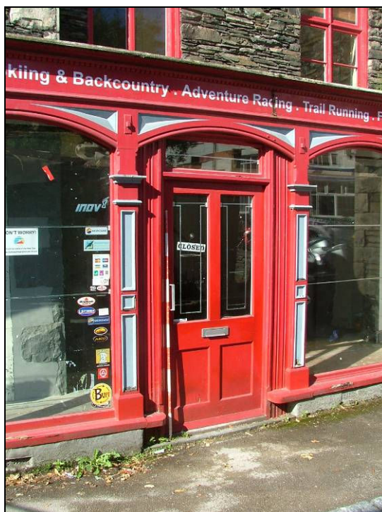
Plate 17: Detail of main entrance in the north elevation (Scale = 2m)
