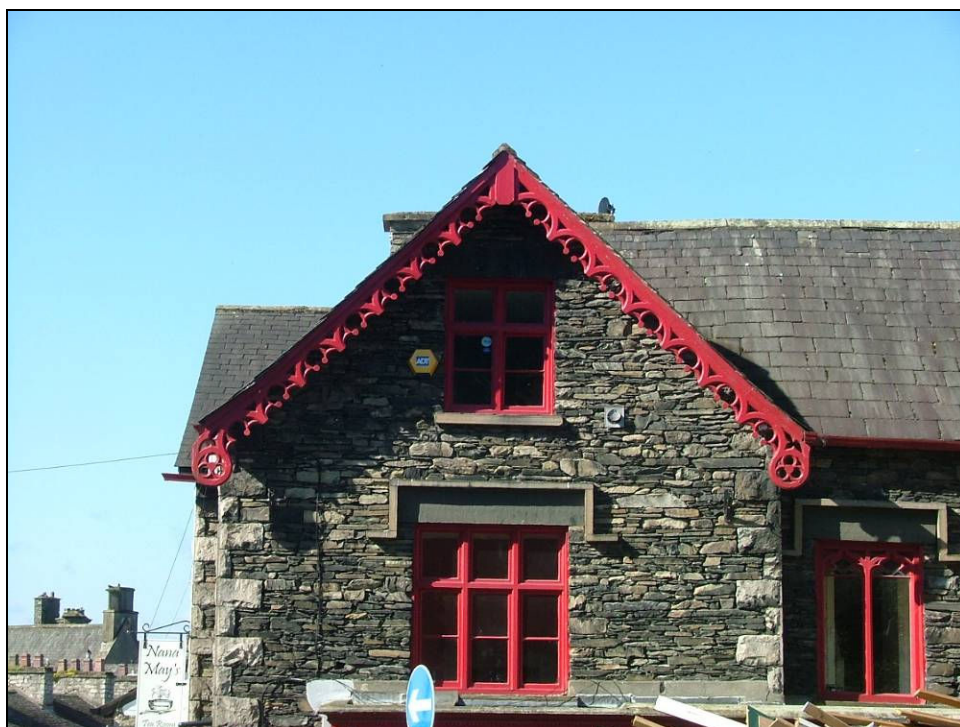
Plate 11: Detail of decorative bargeboards, north elevation of No. 2 Victoria Street
