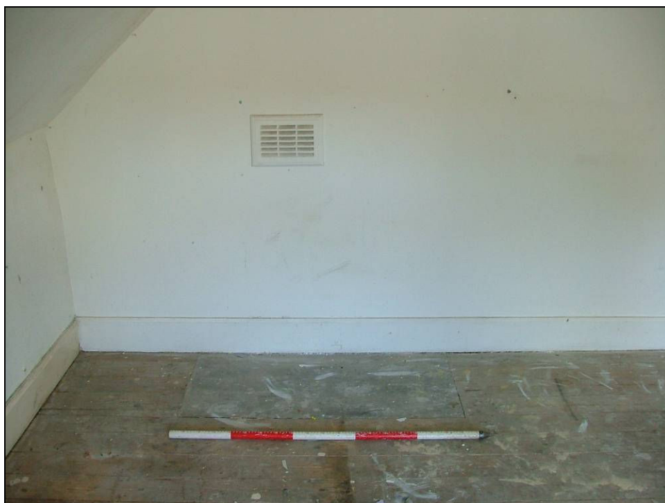
Plate 71: Location of former fireplace, east room, second floor (Scale = 1m)
