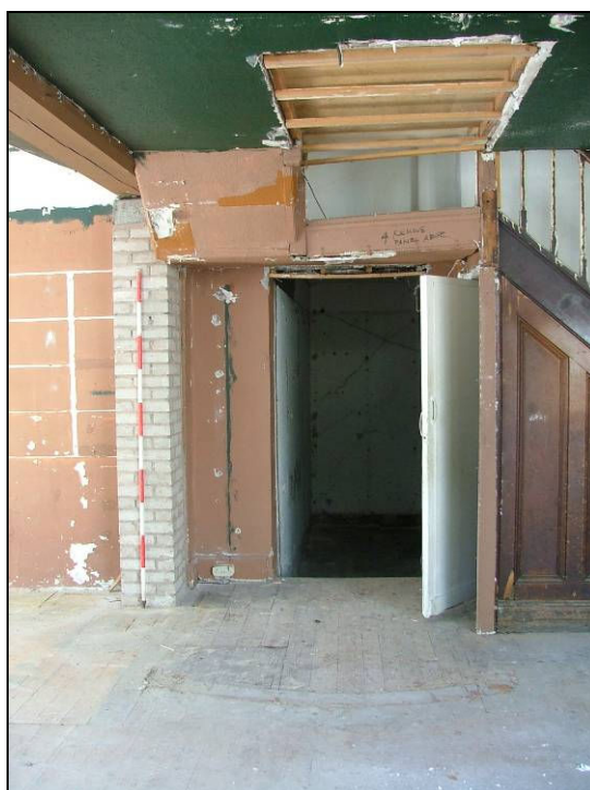
Plate 37: View looking south showing the door to the room to the south (Scale = 2m)
