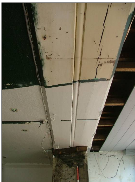
Plate 31: Detail of lintel over large opening in north elevation
