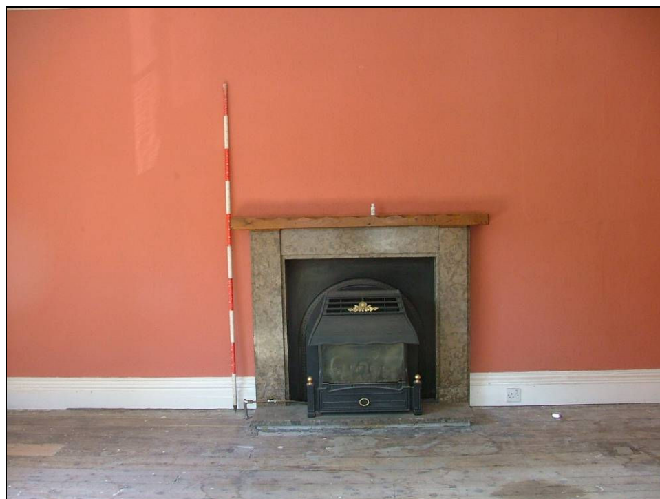
Plate 61: Detail of fireplace, east room on first floor
