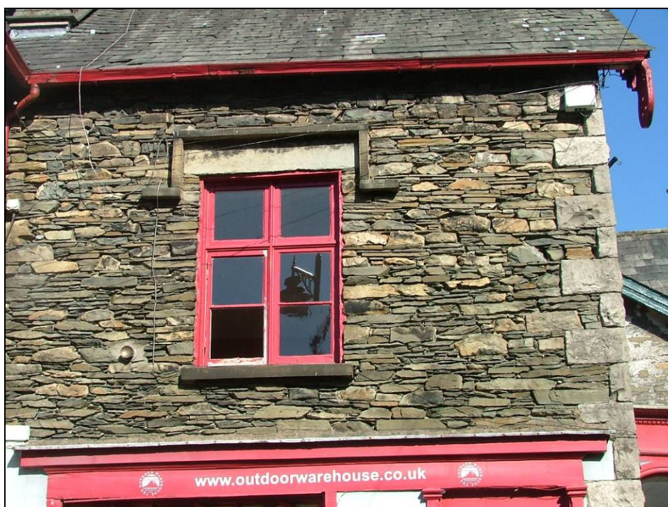
Plate 24: Detail of first floor window, east elevation
