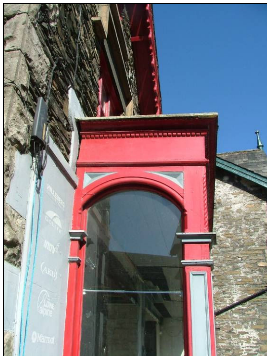
Plate 16: Detail of arched heads and ornamental decoration of the timberwork of the shop front
