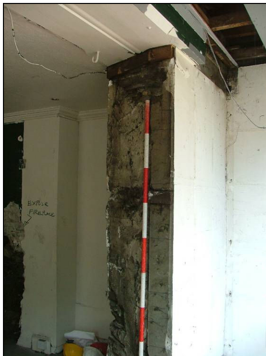
Plate 30: Detail of possible former shop window jamb, ground floor
