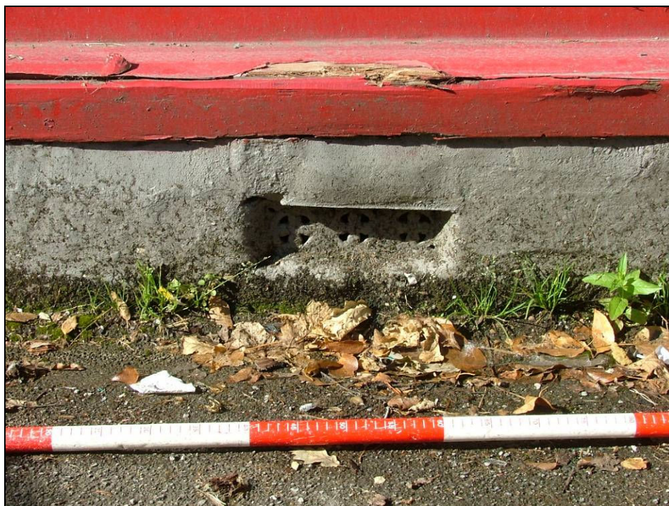
Plate 18: Detail of one of the metal ventilation grills in the stall riser of the shop front
