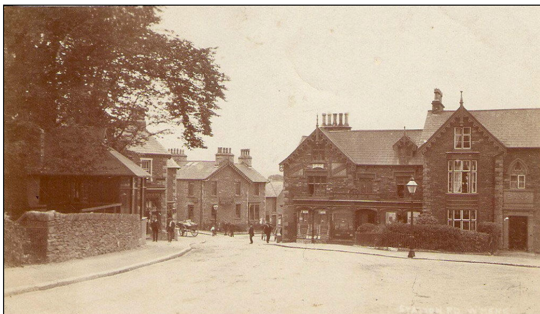
Plate 5: View looking south showing the north elevation of No. 2 Victoria Street, with No. 1 High Street to right of photograph
