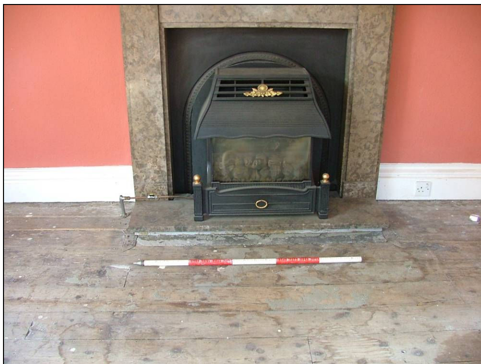
Plate 62: Evidence of earlier hearth below the modern fireplace, east room, first floor (Scale = 1m)
