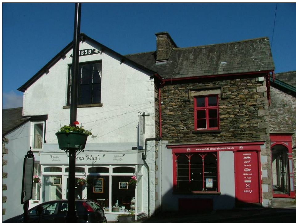
Plate 8: East elevations of No.2 (right) and No. 4 (left) Victoria Street showing a date stone of 1859
