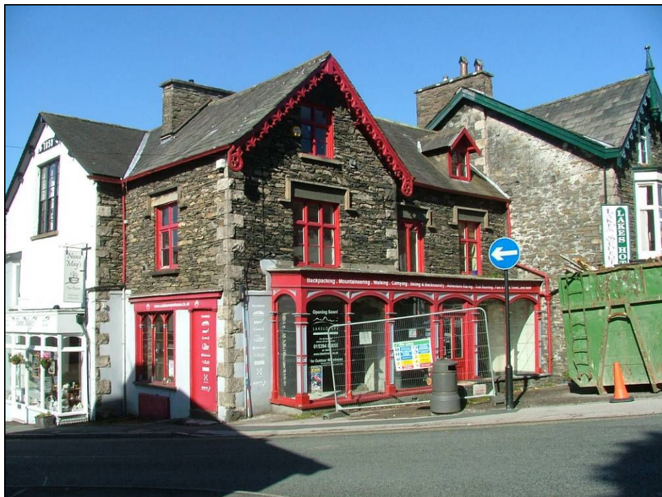
Plate 7: North elevation of No. 2 Victoria Street
