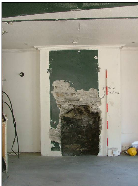
Plate 32: Detail of fireplace, ground floor (Scale = 2m)
