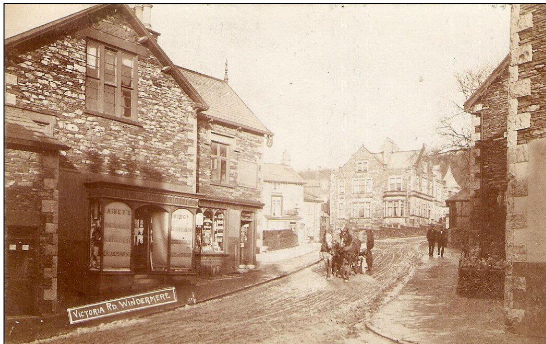
Plate 6: View looking north showing No's 2 and 4 Victoria Street to left of photograph
