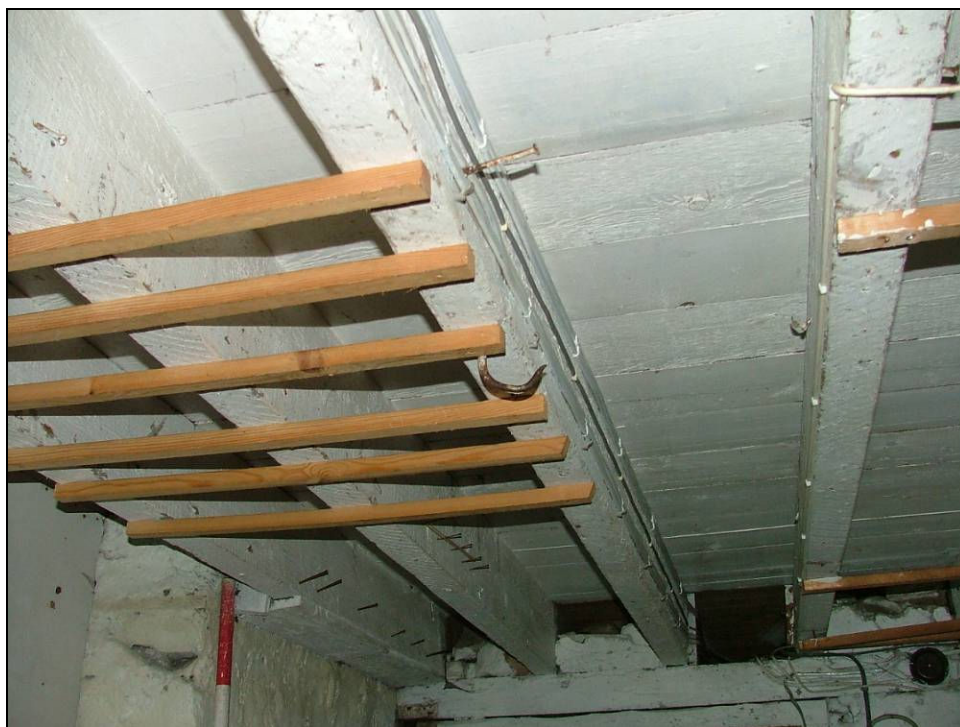
Plate 48: Possible meat hook, ceiling of cellar
