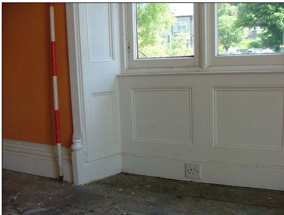
Plate 58: Detail of panelling and decorative detailing, first floor window, north elevation
