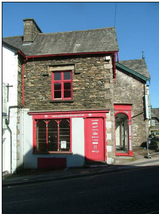
Plate 20: East elevation facing onto Victoria Street
