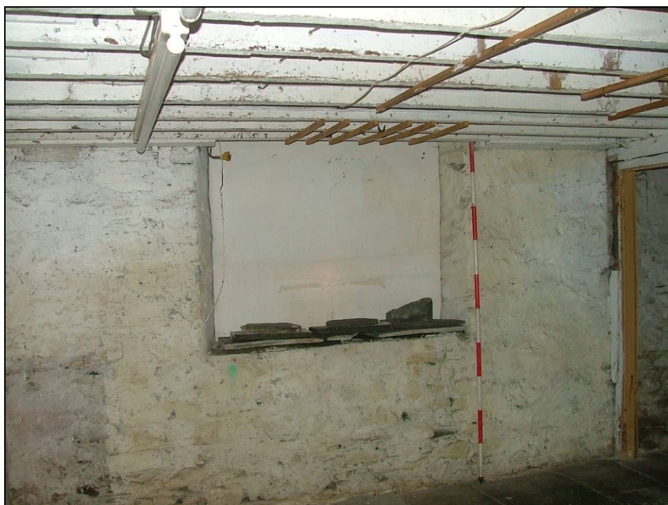
Plate 47: Detail of blocked window, north wall of cellar (Scale = 2m)
