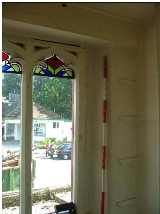
Plate 64: Detail of small room on the first floor
