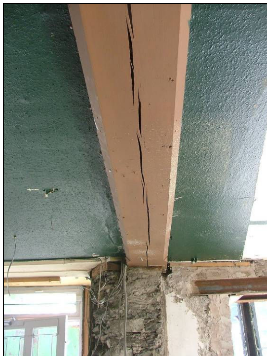
Plate 38: Detail of large beam with chamfered edges, ground floor of northern room
