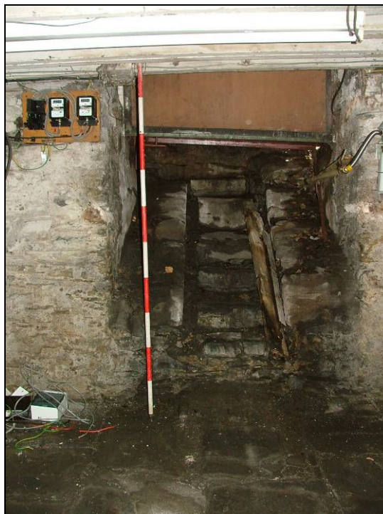
Plate 50: Detail of steps into cellar from the pavement on Victoria Street (Scale = 2m)
