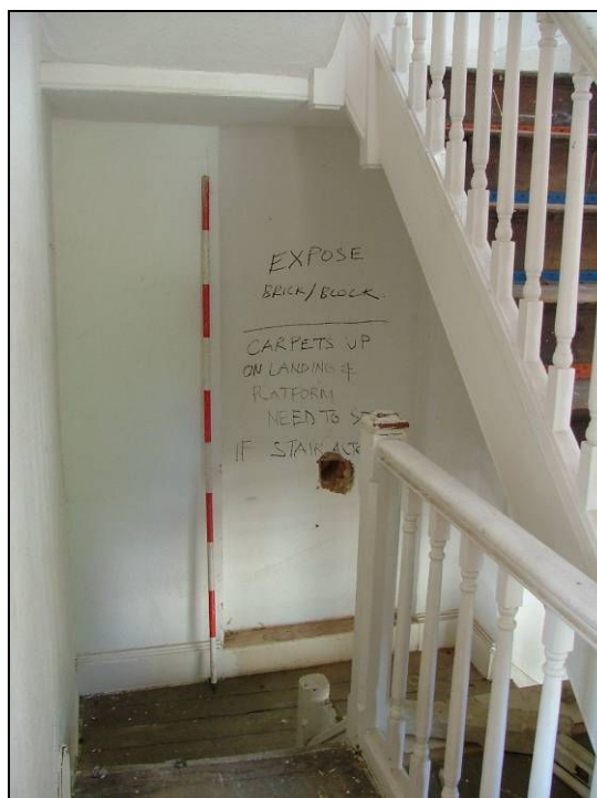
Plate 52: Blocked doorway at the first landing from the ground floor (Scale = 2m)
