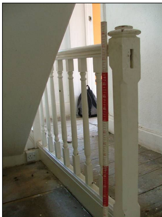
Plate 53: Detail of the balusters and newel post with redundant mortice hole for a handrail, first floor (Scale = 1m)
