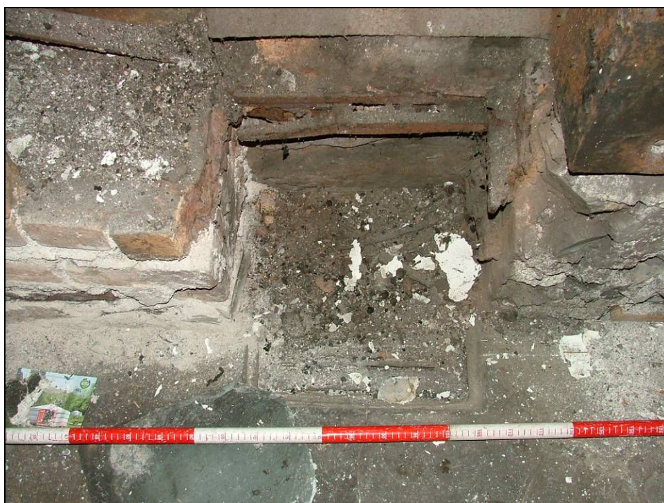
Plate 41: Detail of grate at base of range, ground floor
