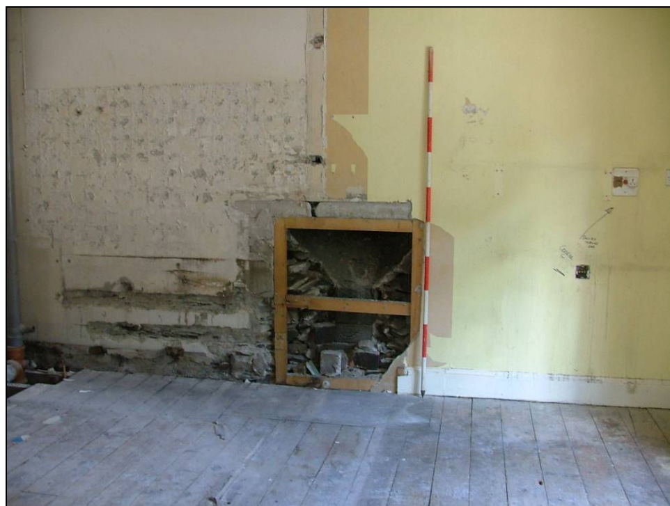
Plate 67: Former fireplace, west wall of first floor (Scale = 2m)
