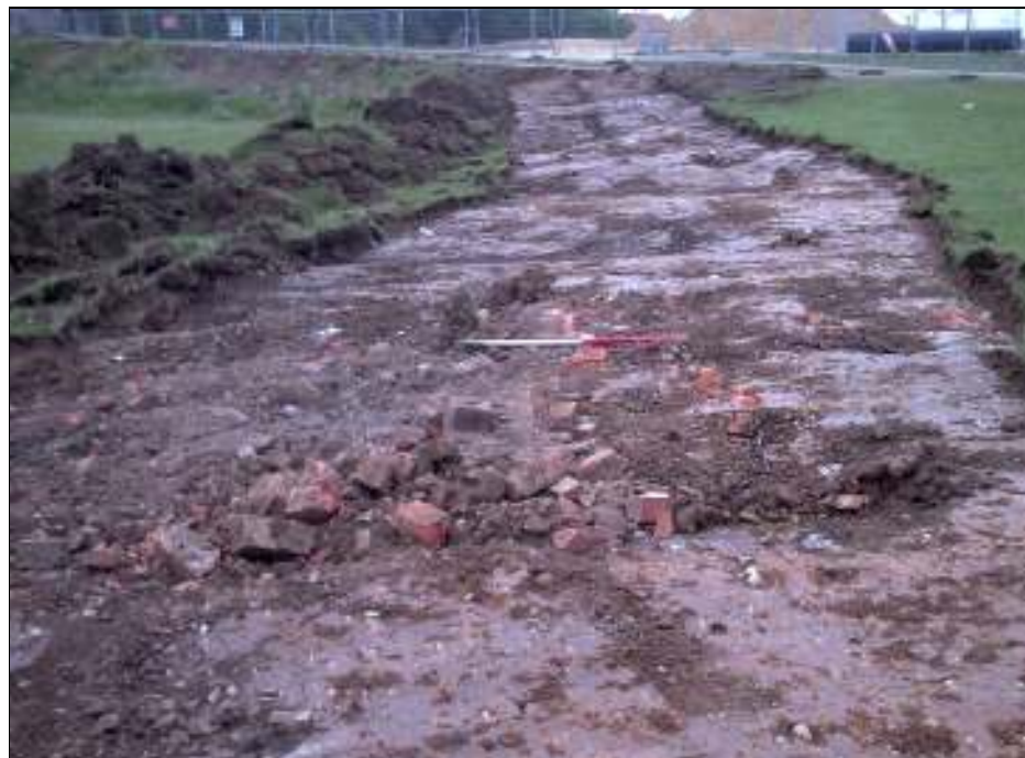
Plate 8: Area of building debris, looking north
