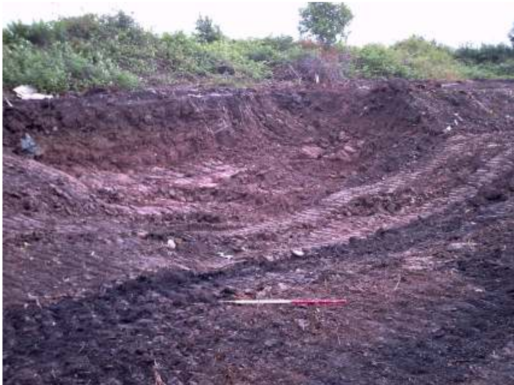
Plate 10: Contaminated soil strip to the east of the rail line, northern end
