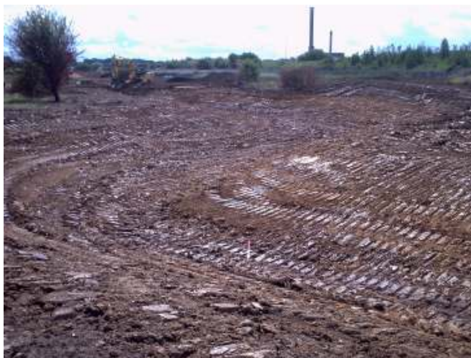
Plate 12: The new channel, west of the Brigham Road
