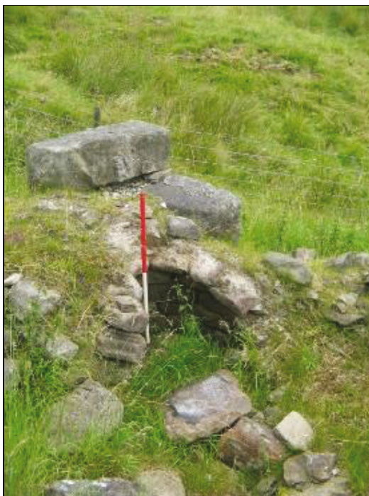
Plate 9: Fireplace / flue along northwestern internal elevation
