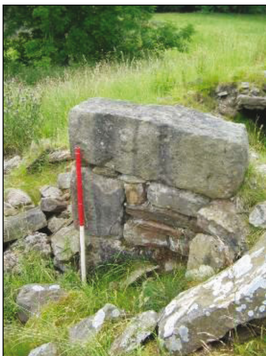
Plate 8: Large masonry appear to have been former corner quoins, looking south
