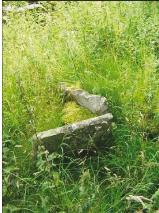
Plate 11: Possible trough to rear of building (north elevation), looking west, southwest
