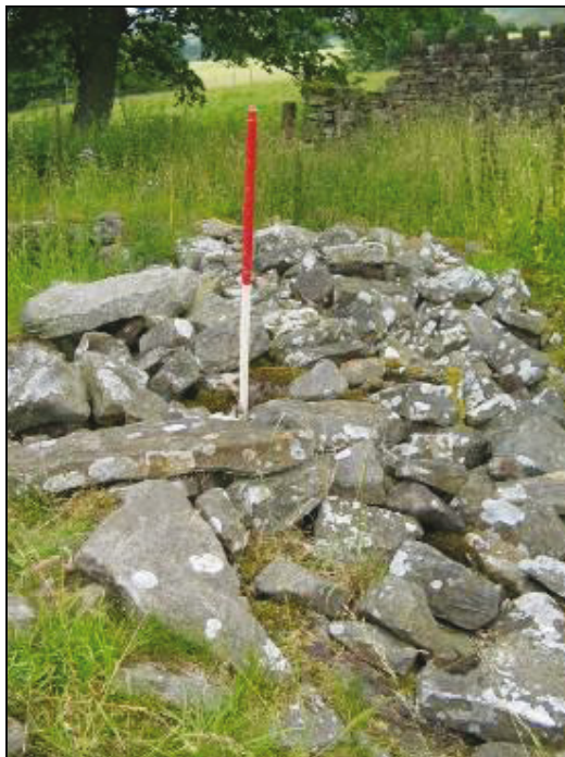
Plate 2: Area of piled building debris to the north of the former building, looking west
