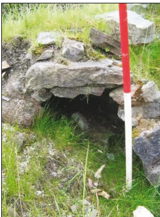
Plate 10: Close up of fireplace / flue on southwestern internal elevation
