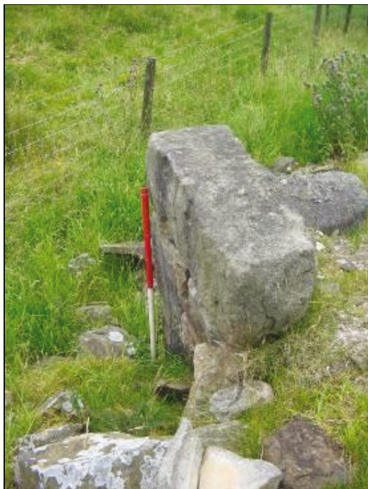
Plate 7: Remains of standing wall on north elevation, looking west
