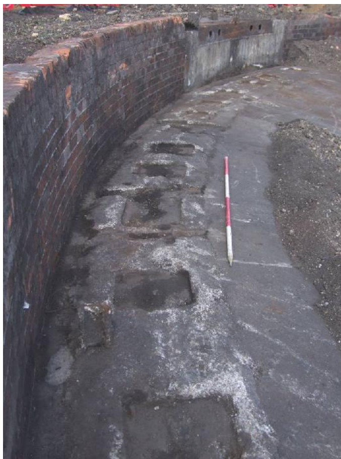
Plate 47: Concrete Fittings 4205 and (left foreground) rail <4207>. Facing South.
