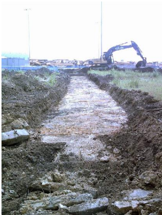
Plate 30: Trench 55. Facing South-west.
