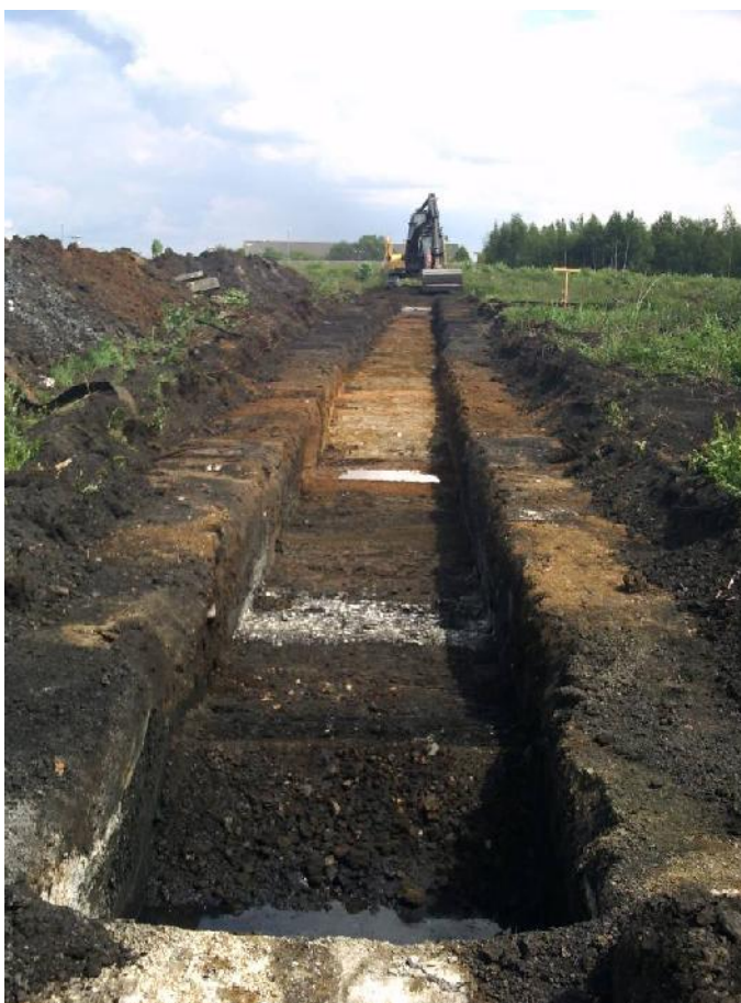
Plate 16: Working Shot Showing Backfilled Modern Excavation 1904. Facing East.
