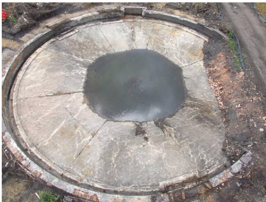
Plate 43: Turntable 1. Aerial View. Facing South.
