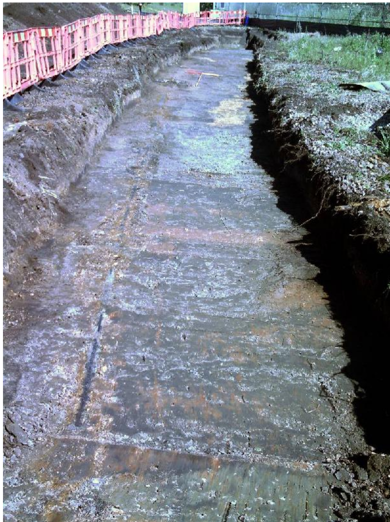
Plate 6: Trench 4. Facing south-west.
