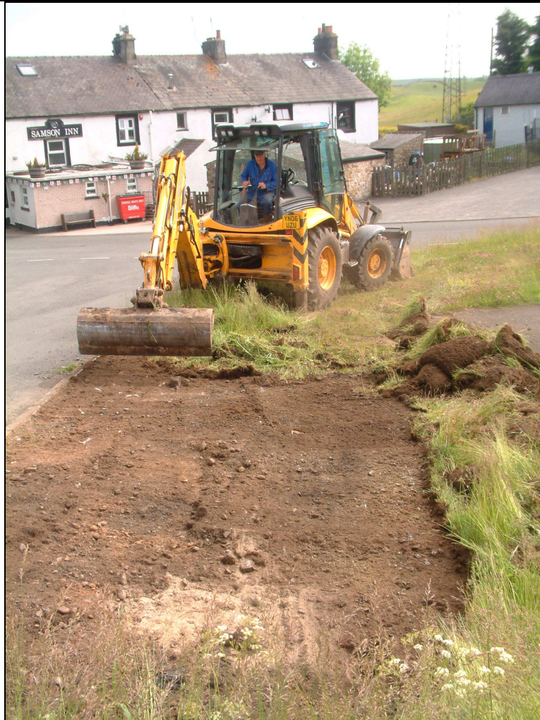
Plate 1: Topsoil stripping on day one, looking east
