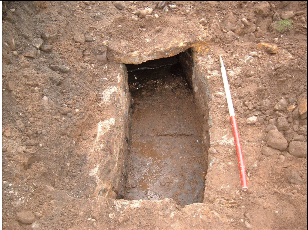
Plate 9: Stone lined culvert encountered on day five during the excavation of Trench Four
