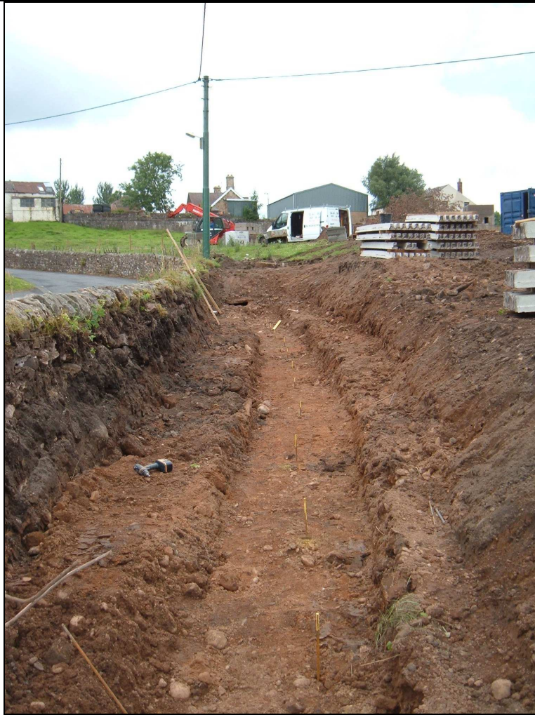
Plate 8: Trench Four looking south on day five
