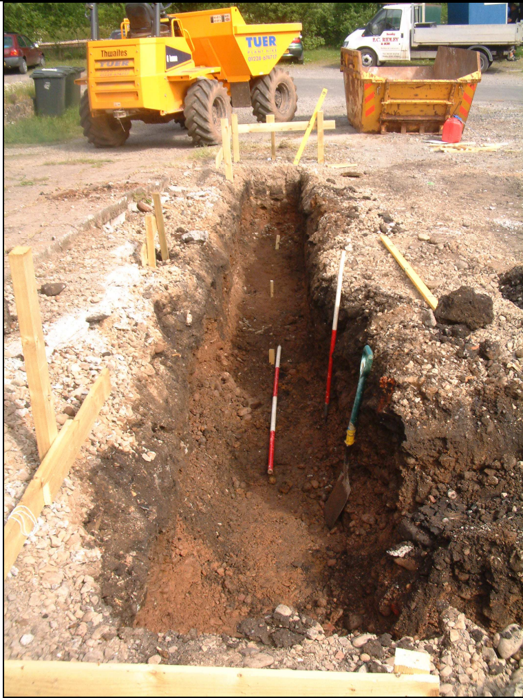
Plate 4: Western edge of Trench Two looking north on day three
