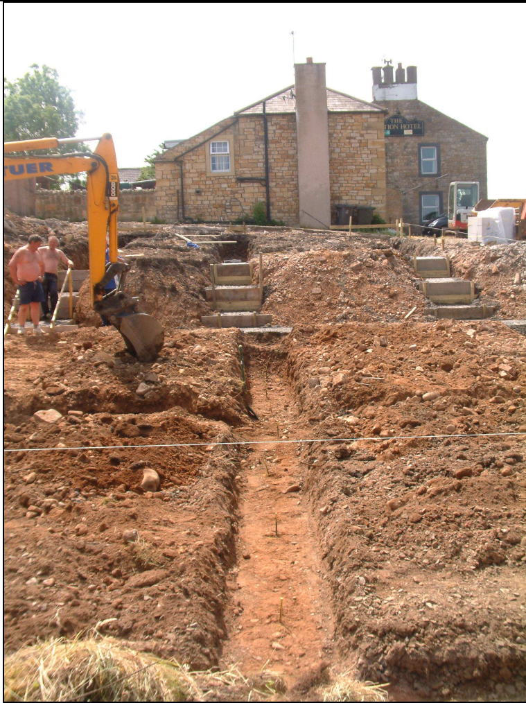
Plate 6: Trench Three looking west on day four
