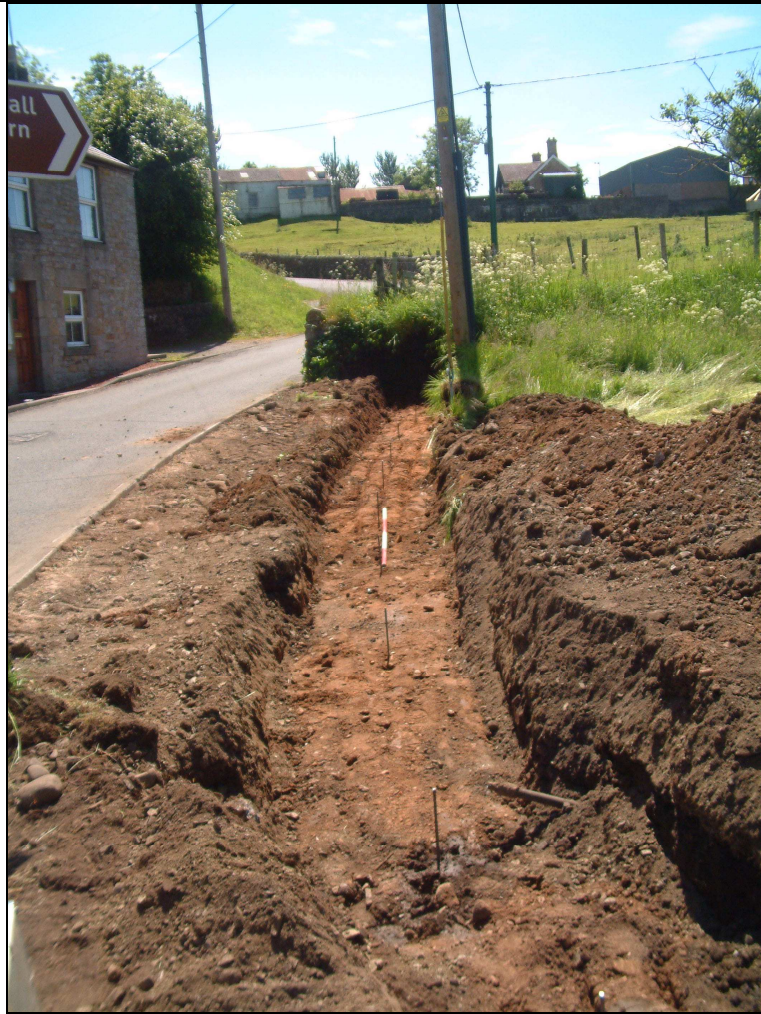
Plate 3: Trench One looking south on day one
