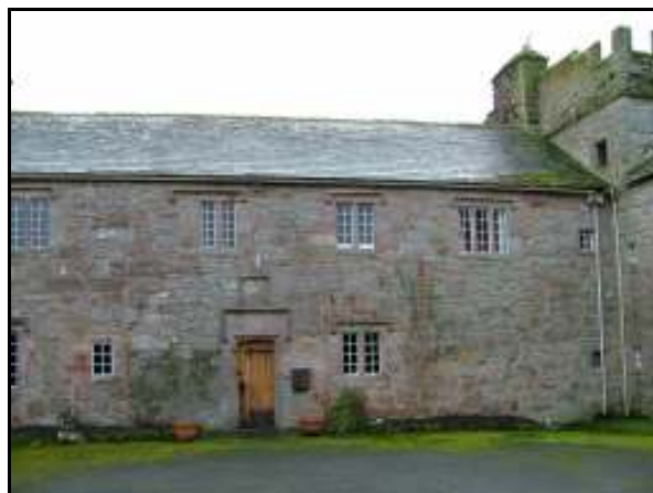
Plate 1: The Hall Block from the northwest
