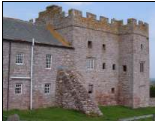
Plate 3: The South Tower and West Range, looking east
