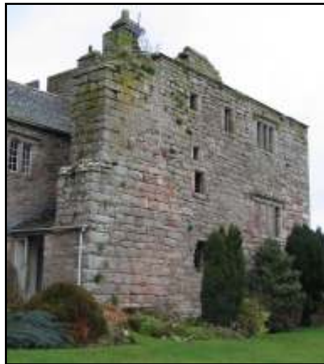
Plate 2: The North Tower and chimneystack, looking north
