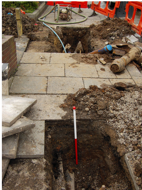
Plate 5. Area B. Trenches 1 and 2 looking west.
