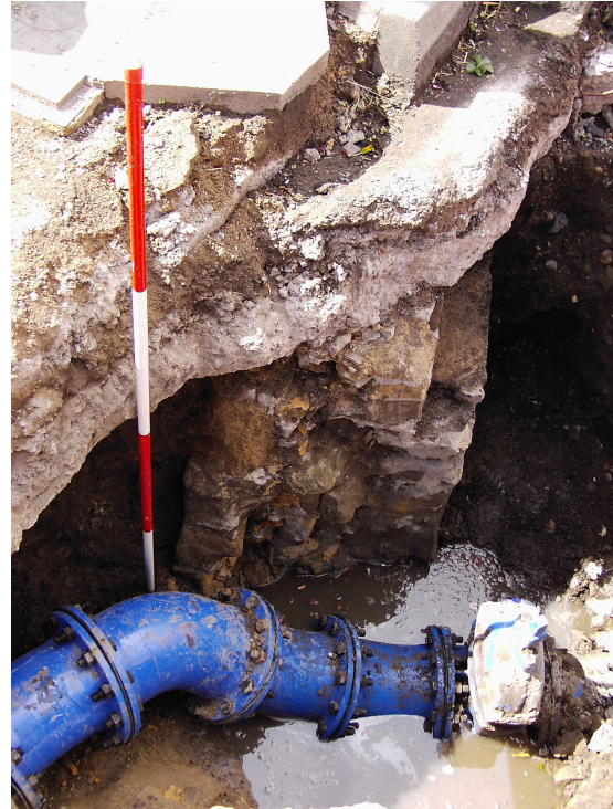
Plate 3. Wall section by new water pipe, looking north-west.
