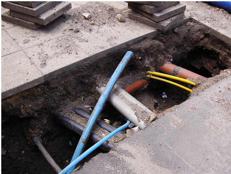
Plate 11. One of the cuts in Area C, showing modern services.
