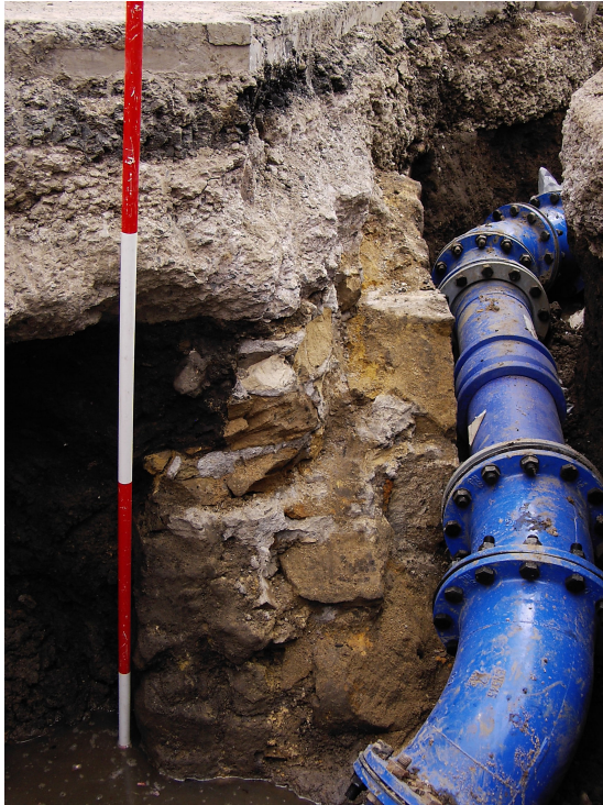
Plate 2. Wall section by new water pipe, looking south-east.
