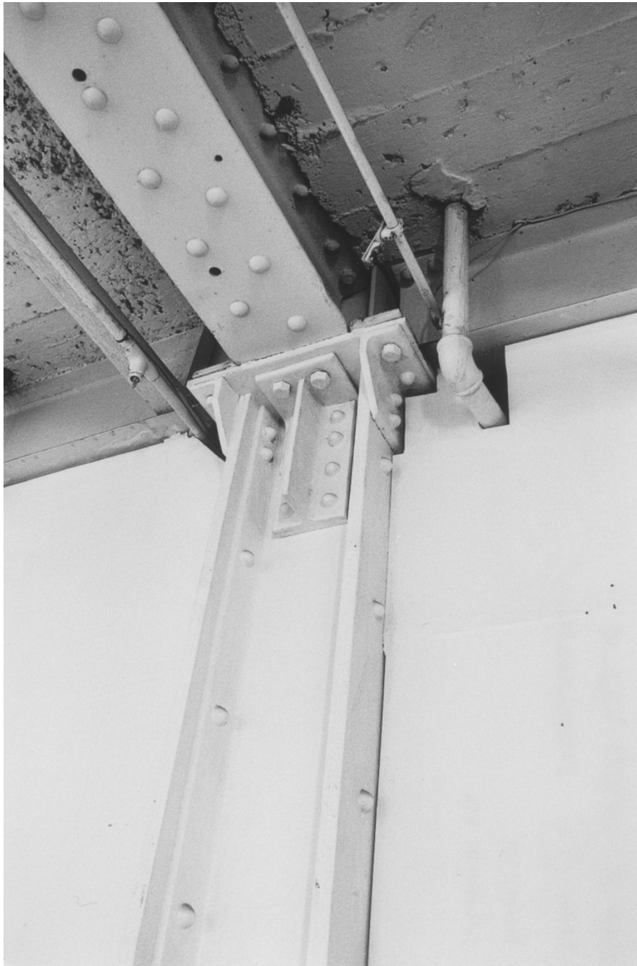
Plate 24 (above) detail of 1905 steelwork in room 53.
