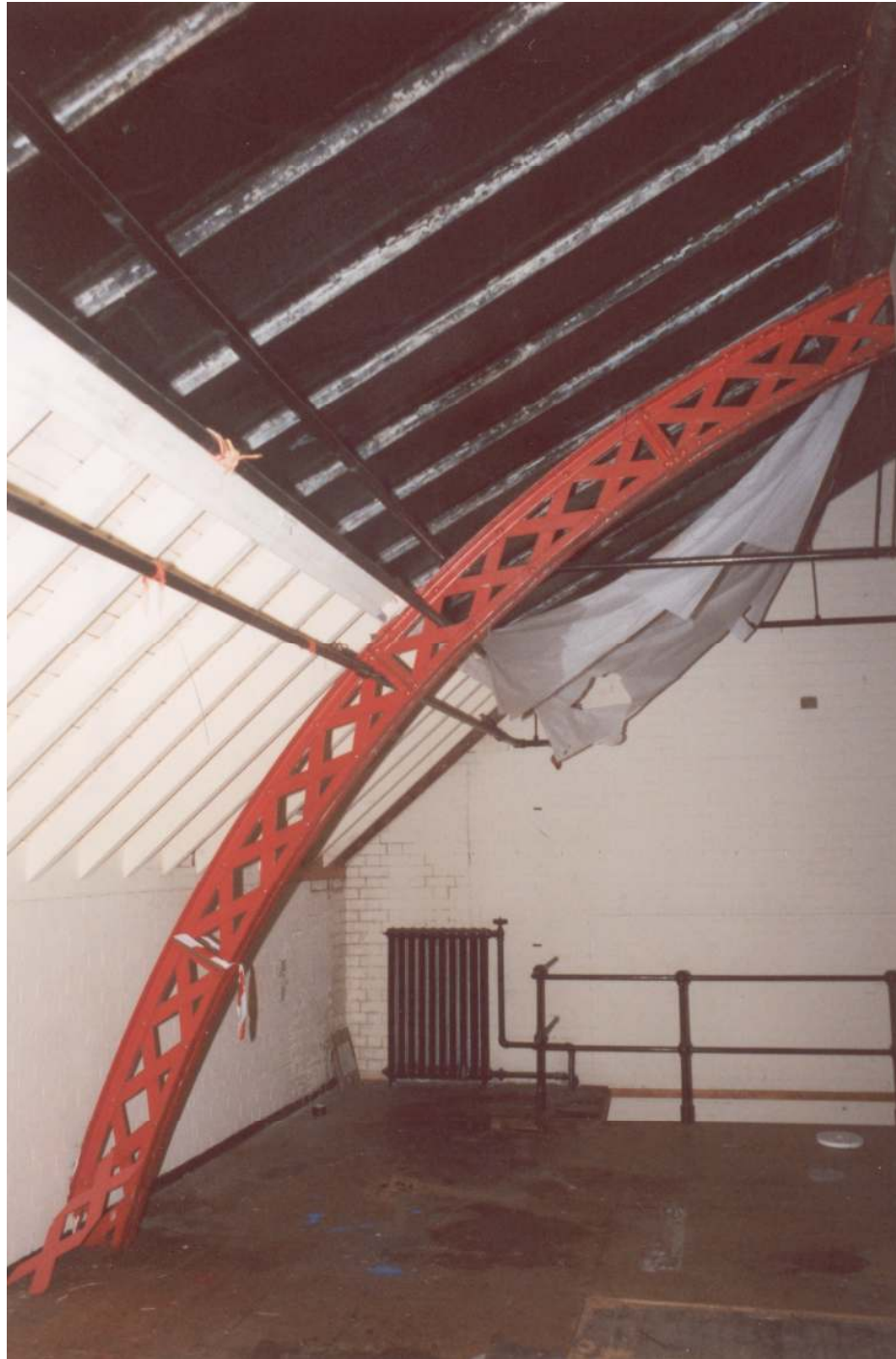
Plate 20: Fourth Floor. Lattice Girder Truss, Room 15, looking east.
