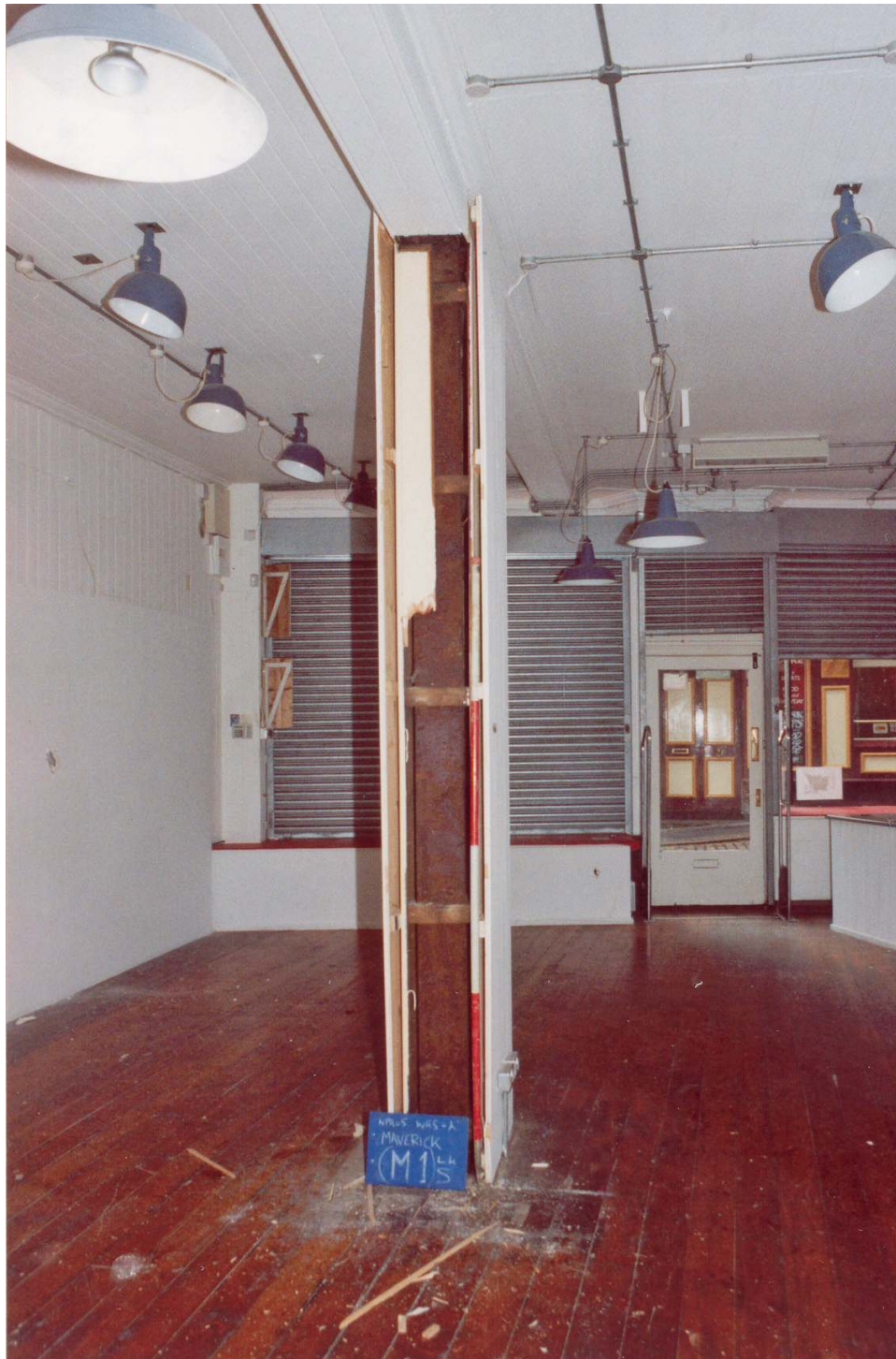
Plate 30: 31 High Bridge. Room M1, looking south, showing steel girder.
