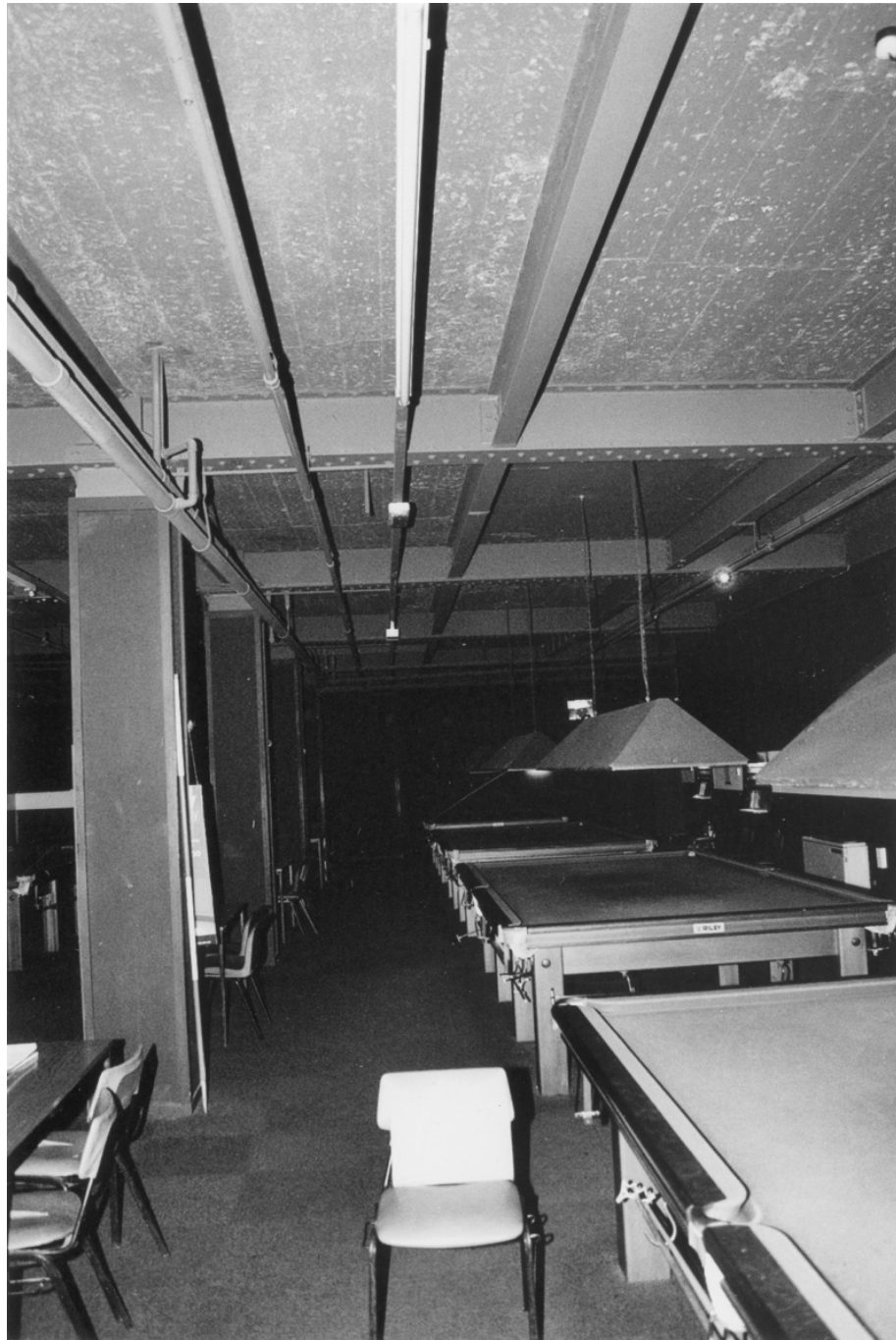
Plate 8: First Floor. Room 86 (Riley's) looking west
