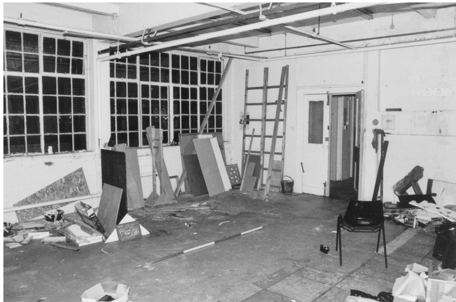
Plate 17 (above): Third floor. Room 30, looking south-west.
