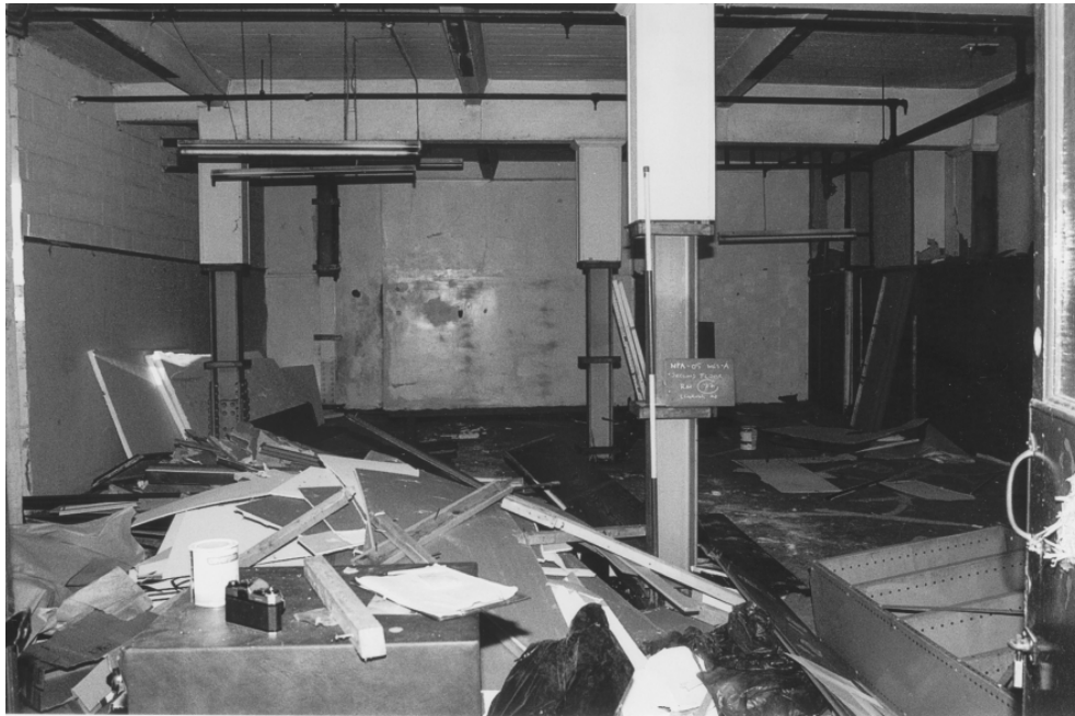
Plate 9: First Floor. Room 77 (Store) looking west
