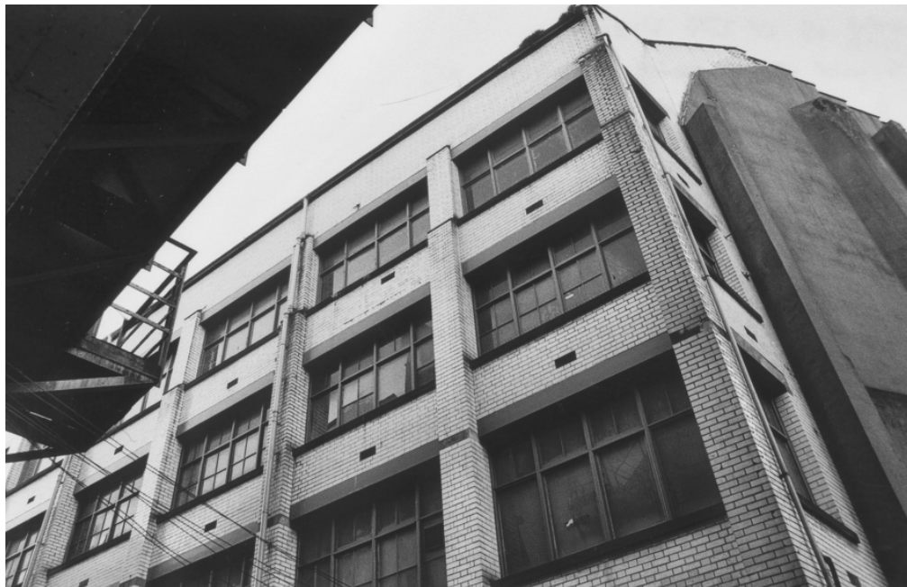
Plate 38: South elevation of 1905 warehouse.
