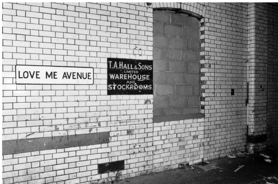
Plate 35: Love Me Avenue: Blocked original entrance to 1905 warehouse.
