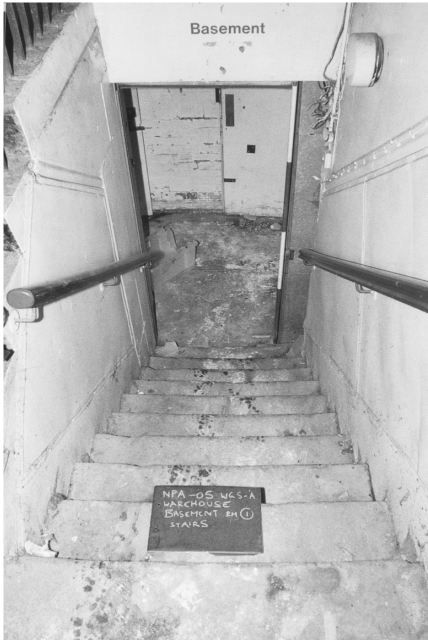
Plate 1: Basement. Room 1 (stairwell) looking north
