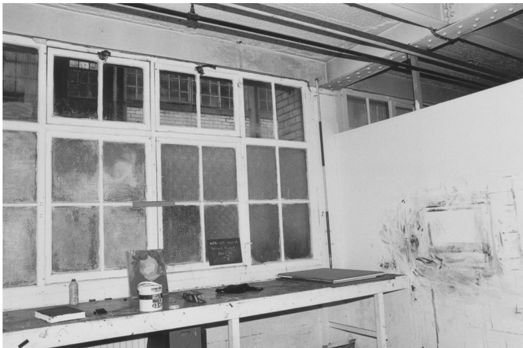
Plate 15 (above): Second Floor. Room 56, looking north-east.
