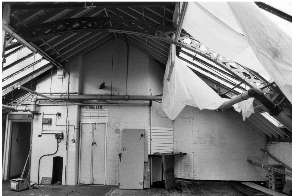
Plate 19: Fourth Floor. Room 15, looking east.
