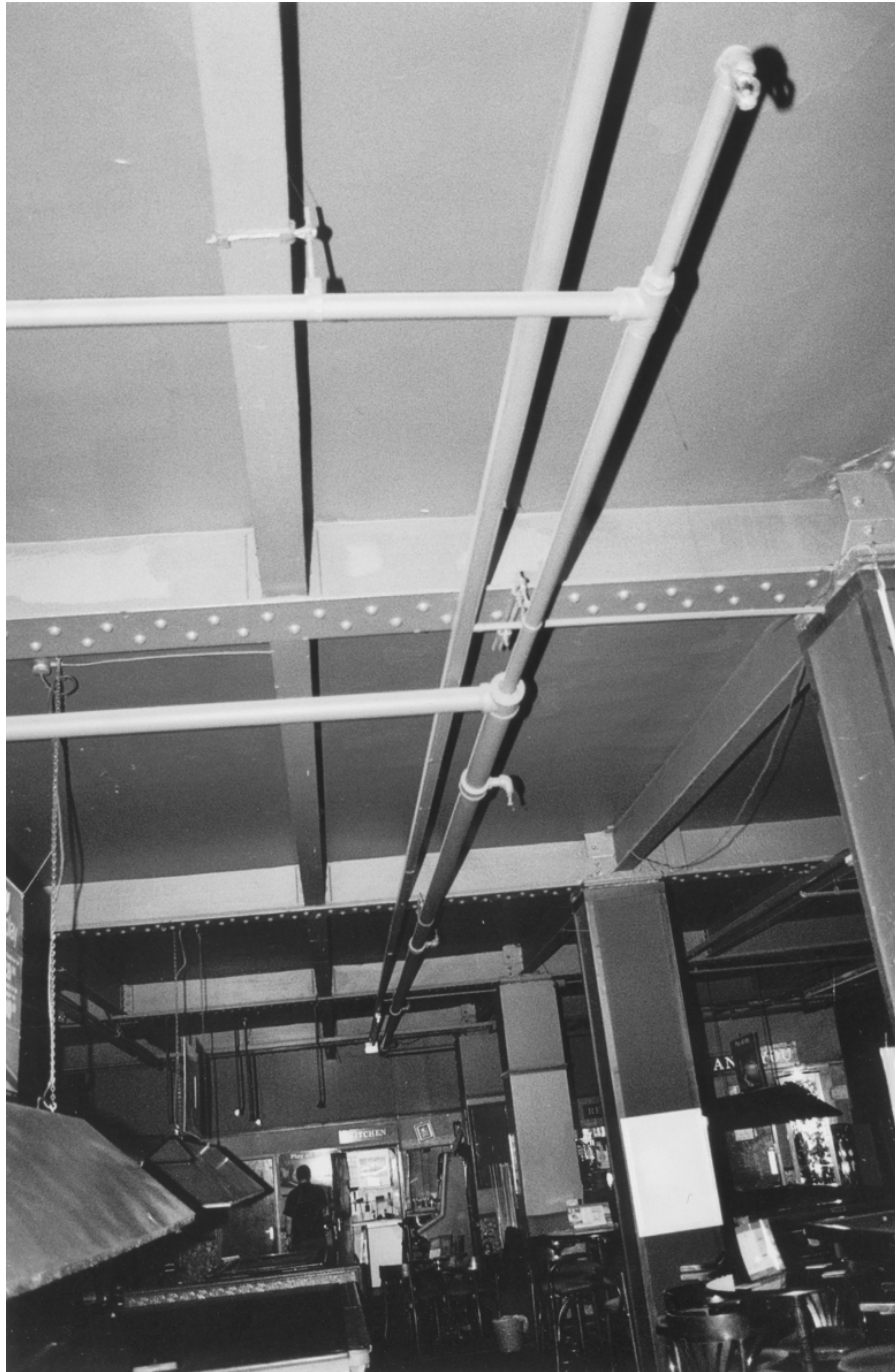
Plate 7: Ground Floor. Room 83 (Riley's) looking east
