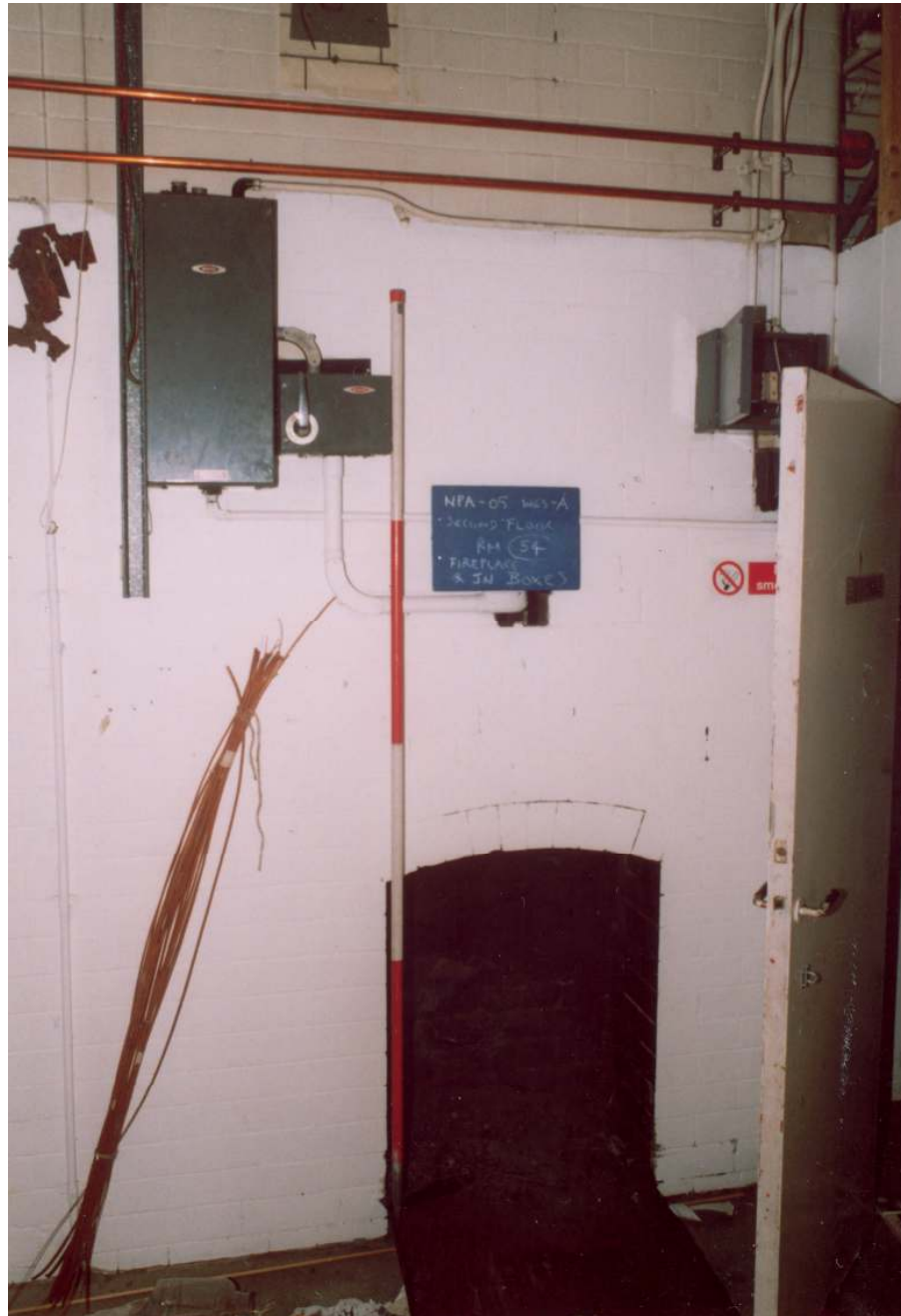
Plate 12: Second Floor. Room 54, fireplace, looking east.
