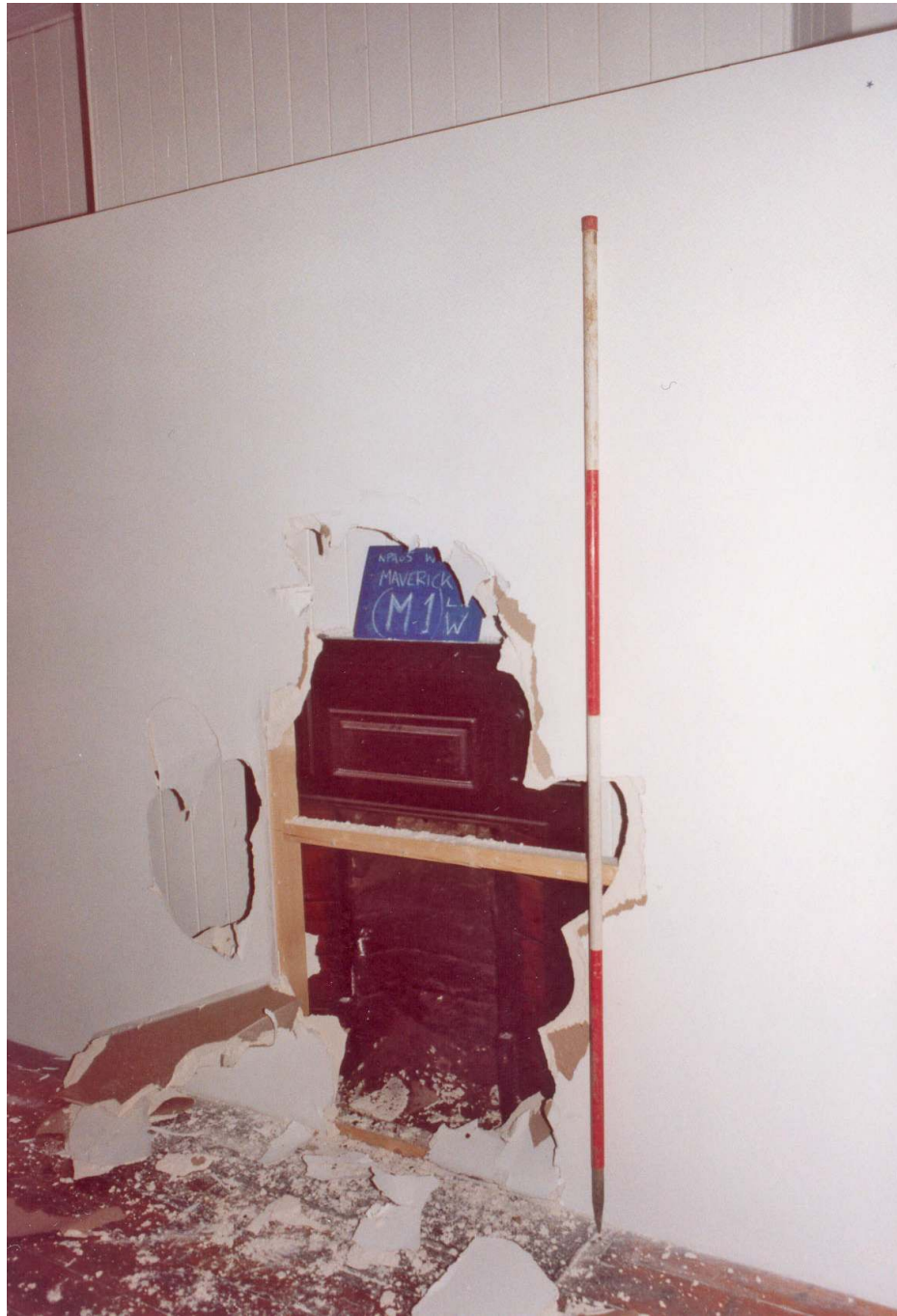
Plate 29: 31 High Bridge. Room M1, west wall. Original fireplace.
