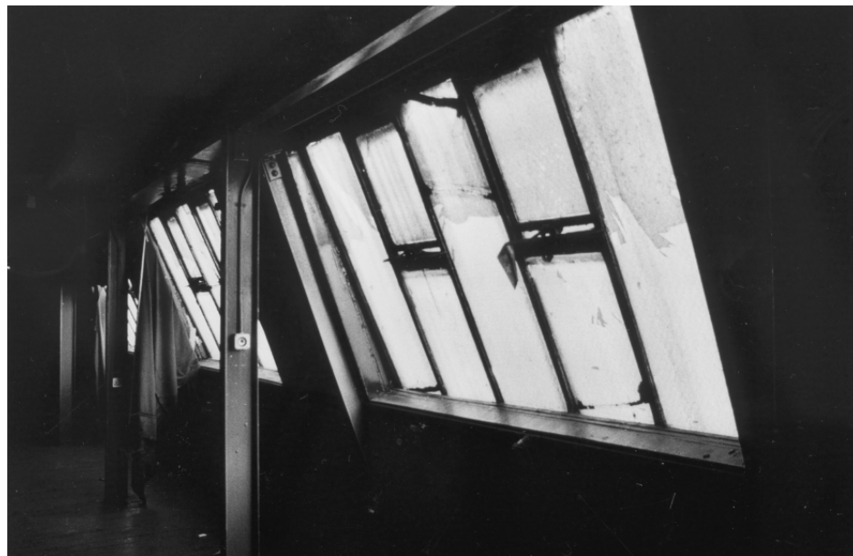
Plate 26: Fourth Floor, warehouse, room 24, detail of windows.
