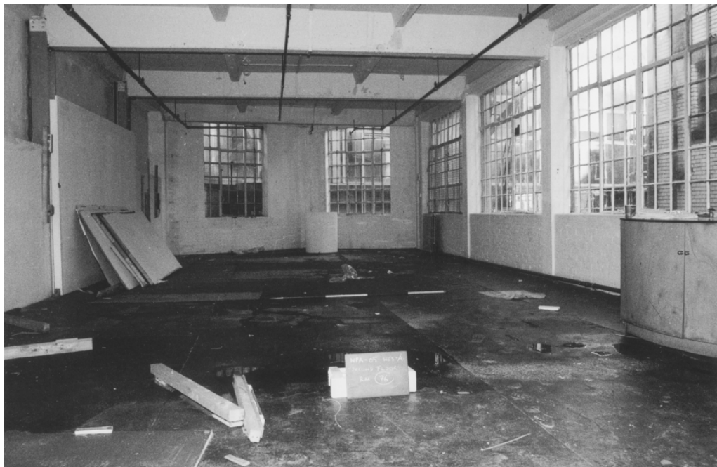
Plate 10: First Floor. Room 76, looking east
