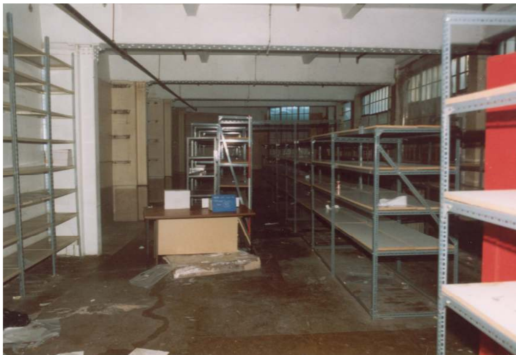
Plate 6: Ground Floor. Room 79 (Store) looking east
