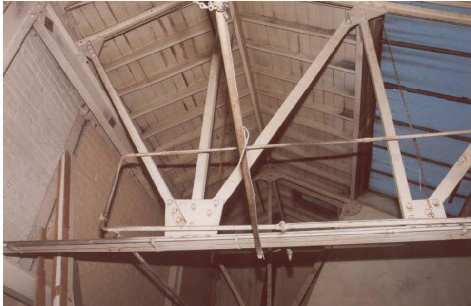
Plate 21: Fourth Floor. Room 13 (1932 building), steel frame roof, looking south.
