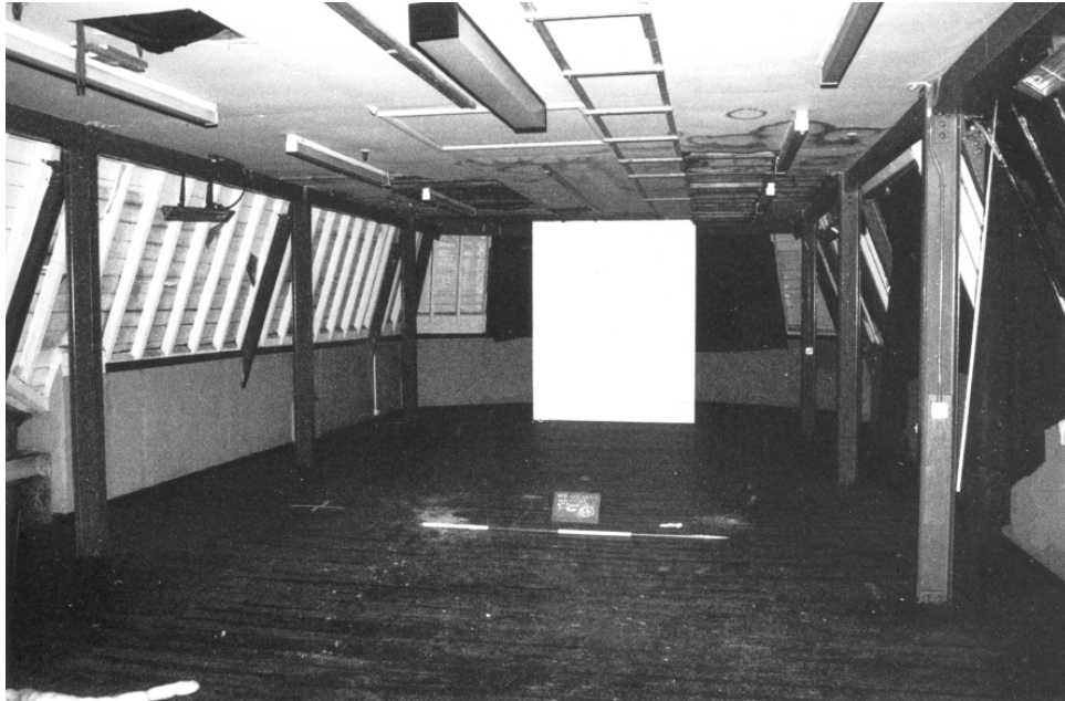
Plate 18: Fourth Floor. Room 24, looking east.
