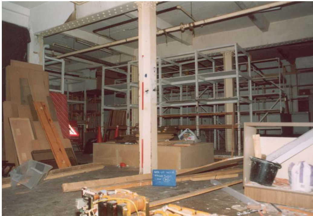
Plate 5: Ground Floor. Room 80 (Store) looking west
