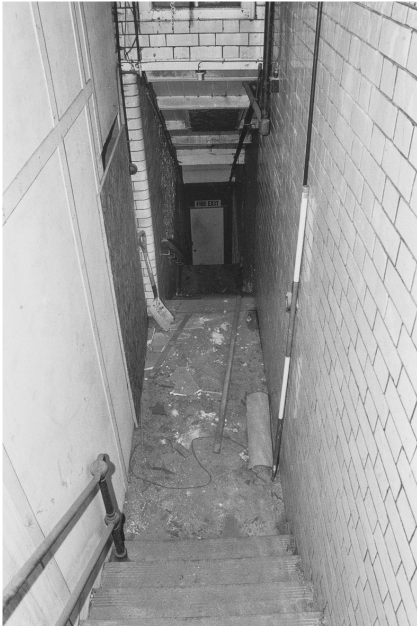
Plate 11: Second Floor. Room 49 (Back Stairs), looking south.
