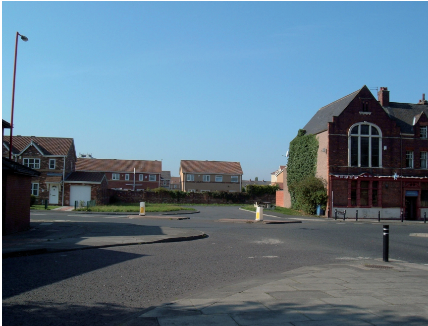
Plate 5: Photograph of the Development site as existing, facing west
