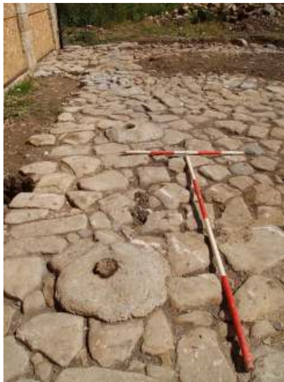
Plate 6: Bases of a modern barn [F213] overlying the post-medieval yard surface, looking east
