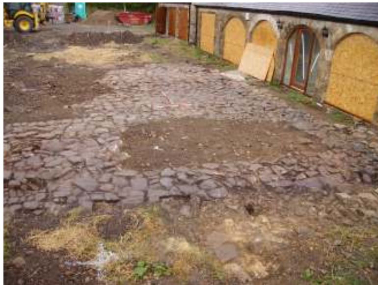
Plate 5: Stone yard surface [201] in Area F from the east
