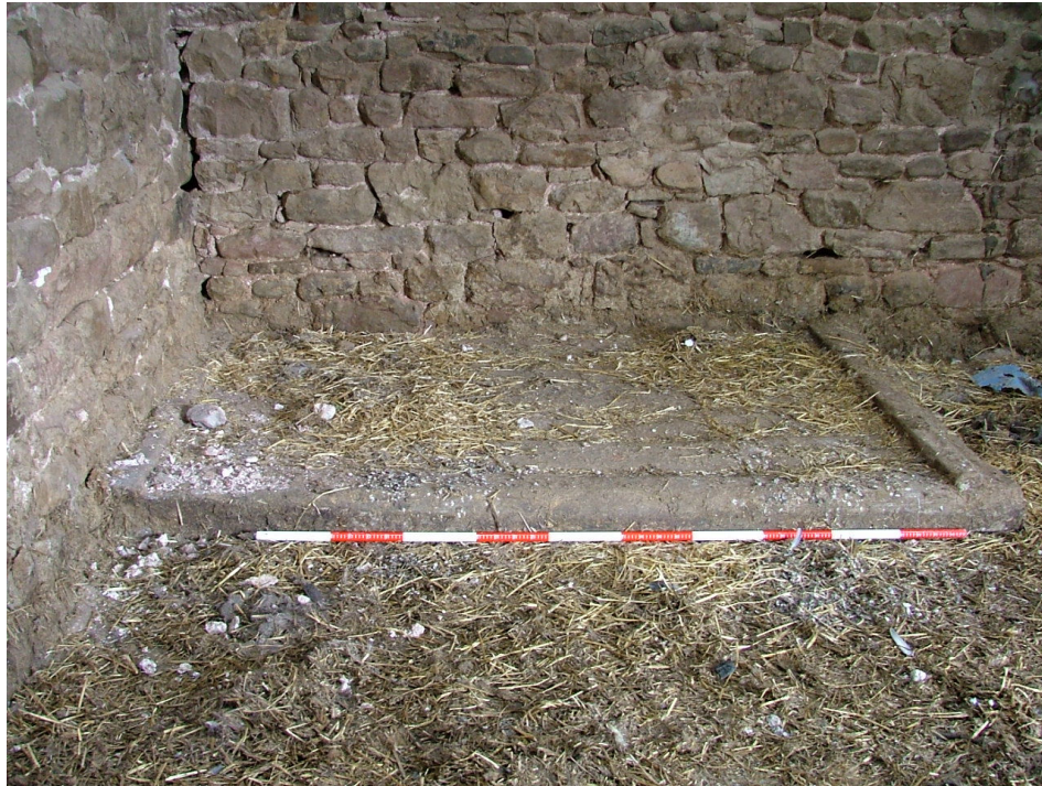
Plate 15 – One of the two timber platforms in the barn
