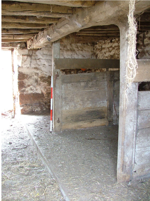
Plate 10 – Interior of western byre
