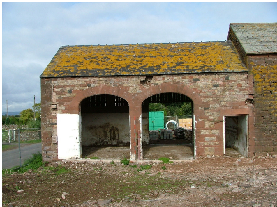
Plate 9 – Southern elevation of the cart shed
