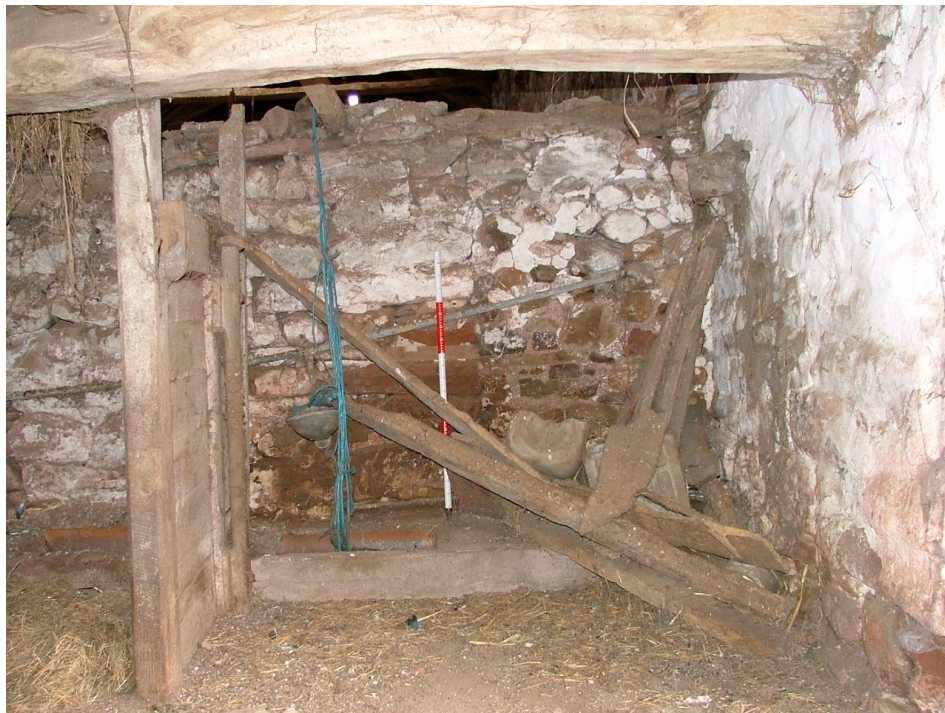
Plate 11 – Possible blocked doorway between western byre and barn
