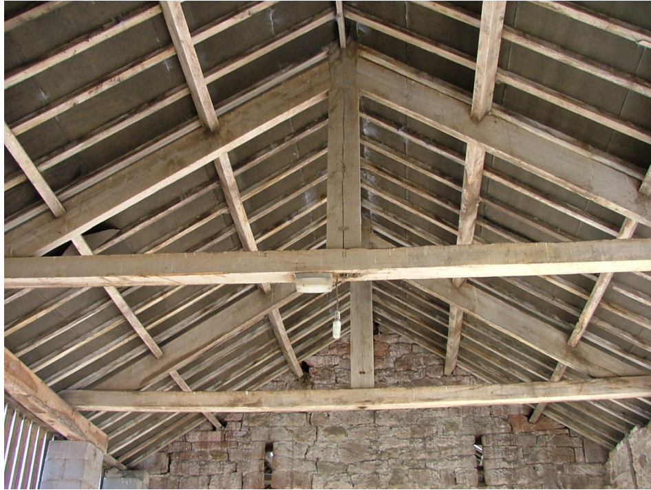
Plate 16 – King post roof trusses, cart shed
