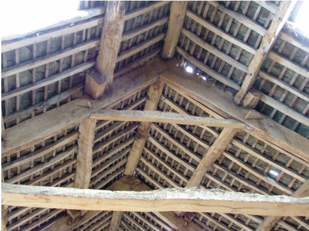
Plate 13 – Roof detail of barn
