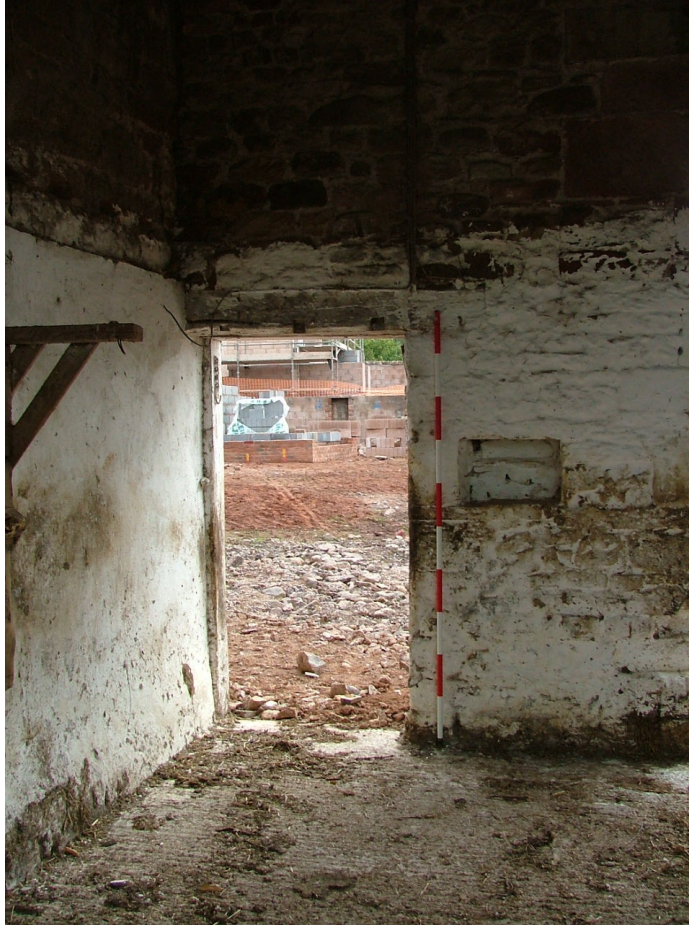
Plate 18 – Doorway and niche, southern wall of cart shed
