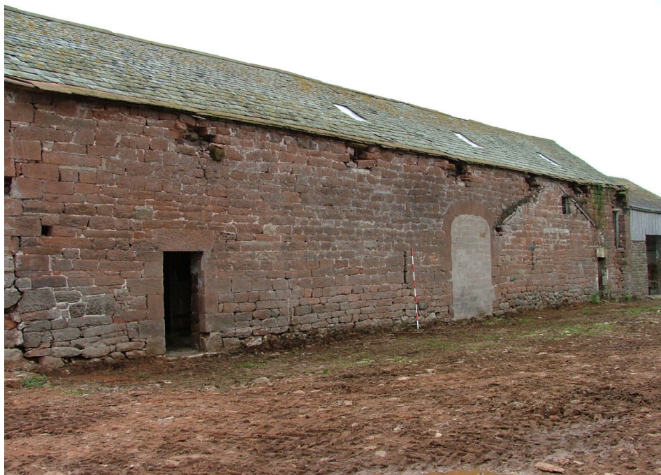
Plate 2 - North elevation of threshing barn
