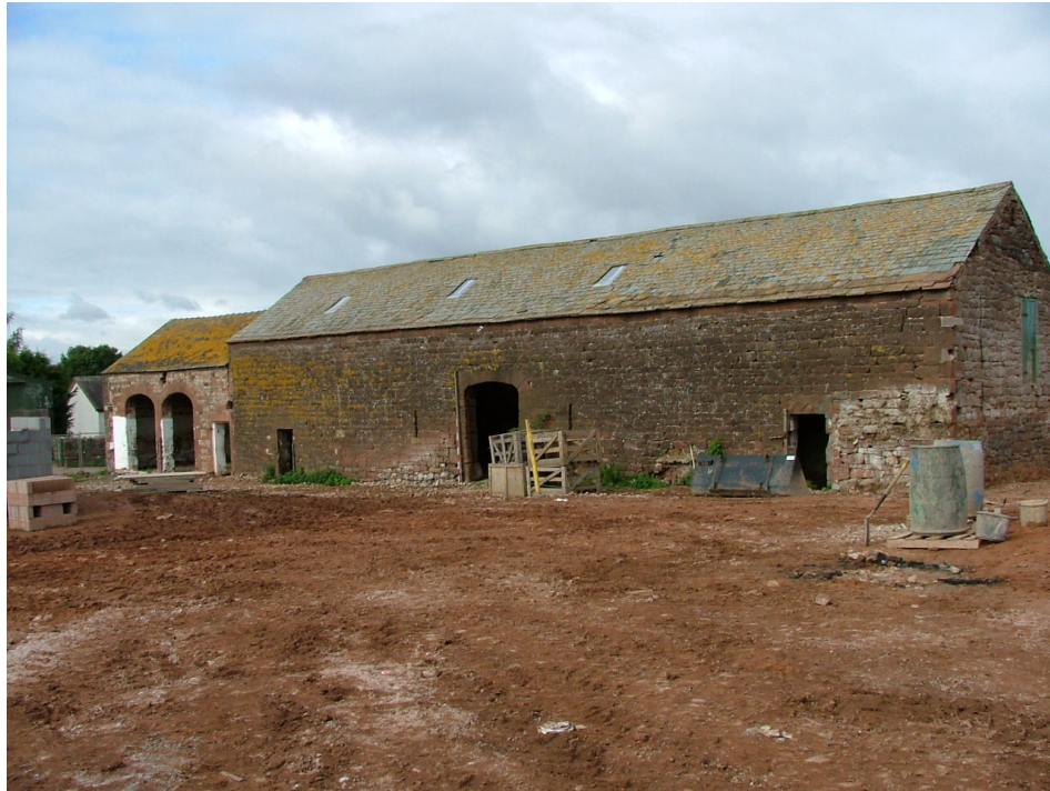
Plate 1 - South facing elevation of barn and cart shed
