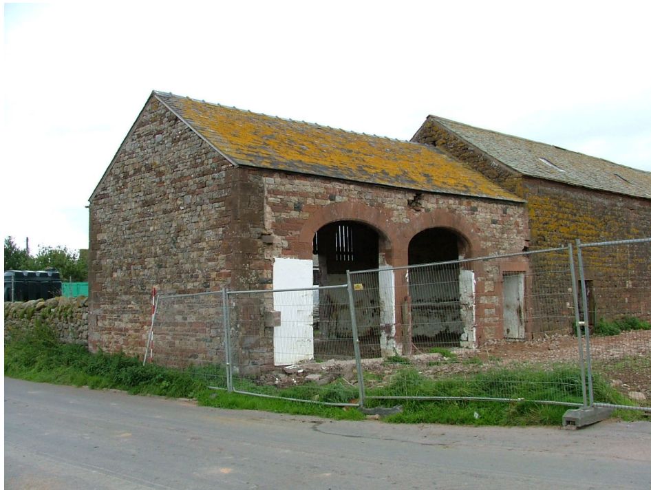
Plate 4 – Western end of barn and gable end of the cart shed
