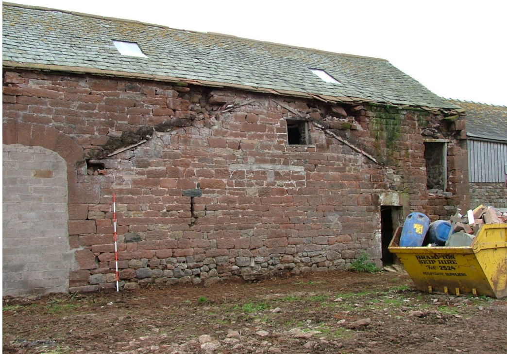
Plate 7 – Scar of the roof line of a gin-case
