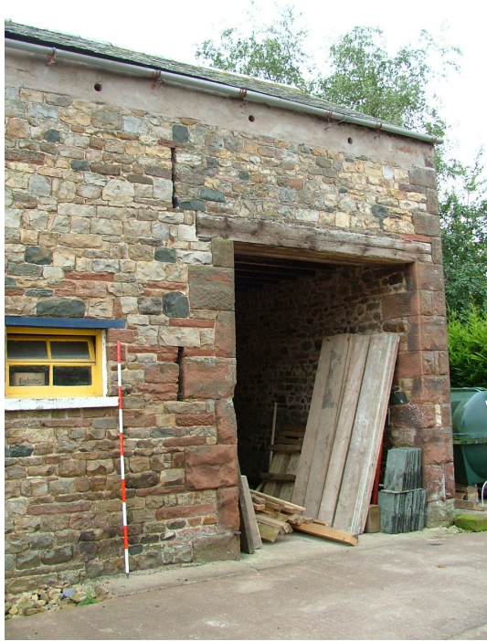
Plate 20 – Large doorway, southern end of Building D
