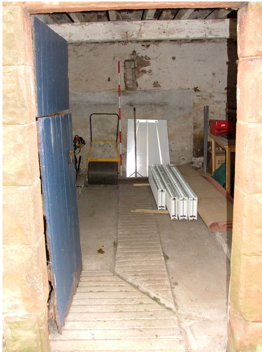
Plate 19 – Interior of byre, Building D
