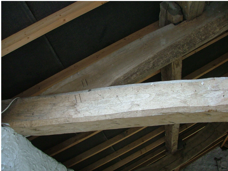
Plate 17 – Assembly mark 'II', roof truss first floor of Building C
