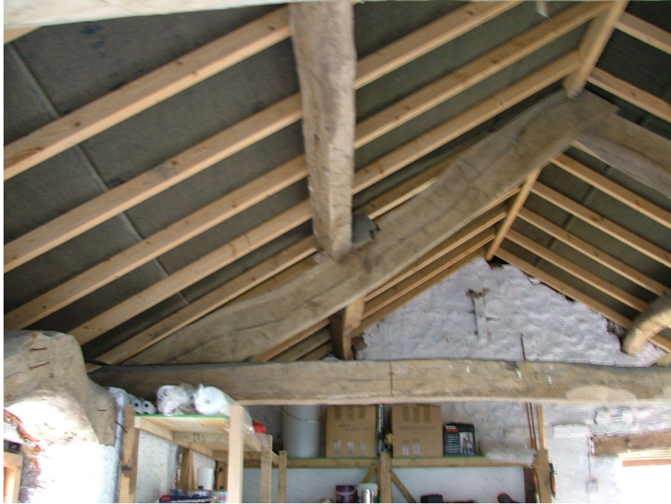
Plate 16 – Roof detail, first floor of Building C
