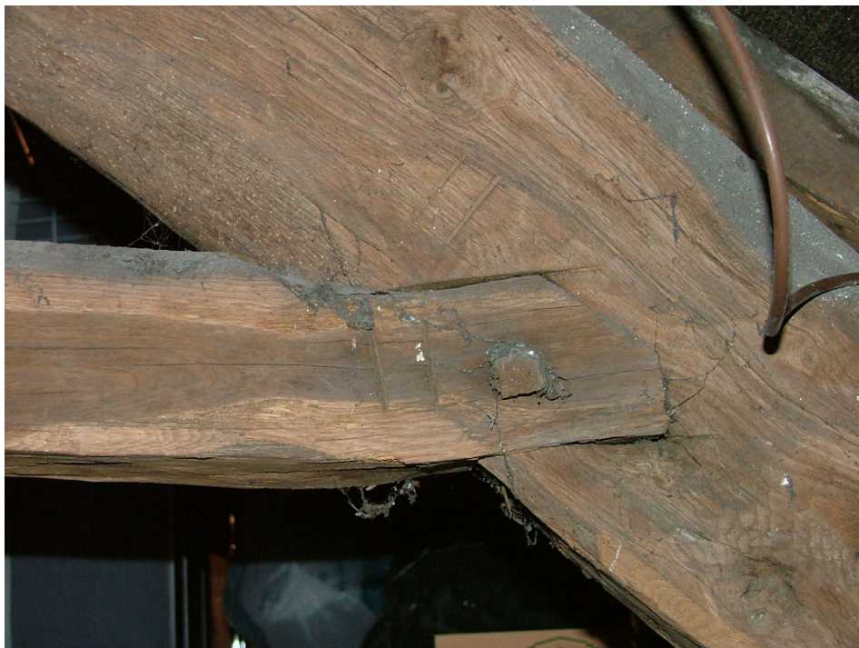
Plate 39 – Detail of joint, peg and assembly mark on roof truss
