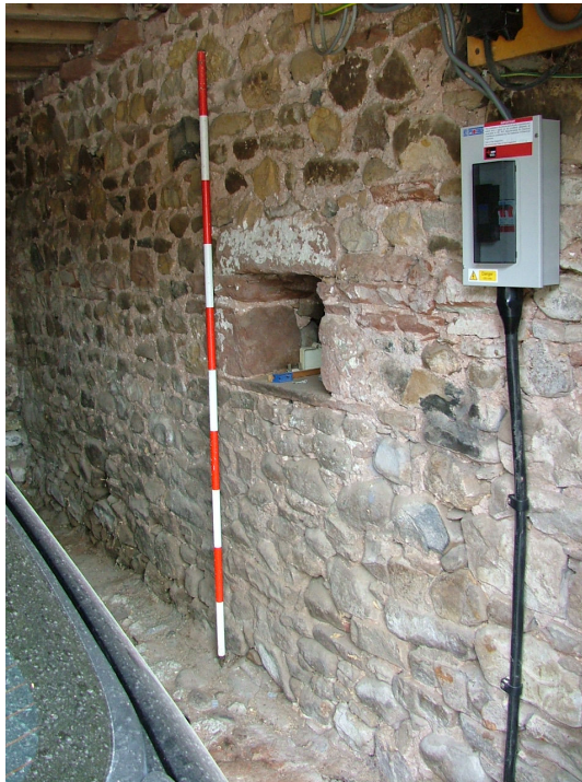
Plate 15 - Niche, interior of cart shed, Building C
