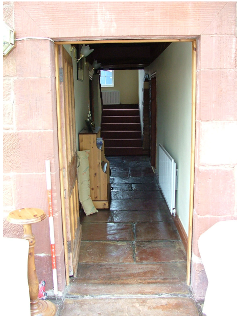
Plate 28 – Hallway of house looking north
