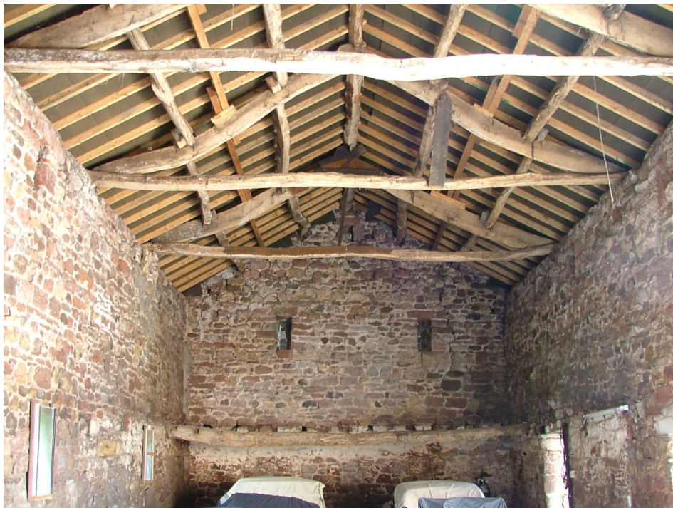
Plate 4 – Eastern gable end of Building A. Remains of limewash and rafter holes can be seen providing evidence for a former first floor
