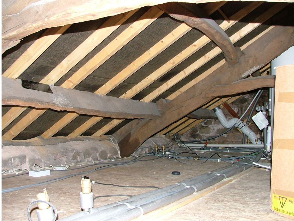
Plate 38 – Roof structure, main section of house
