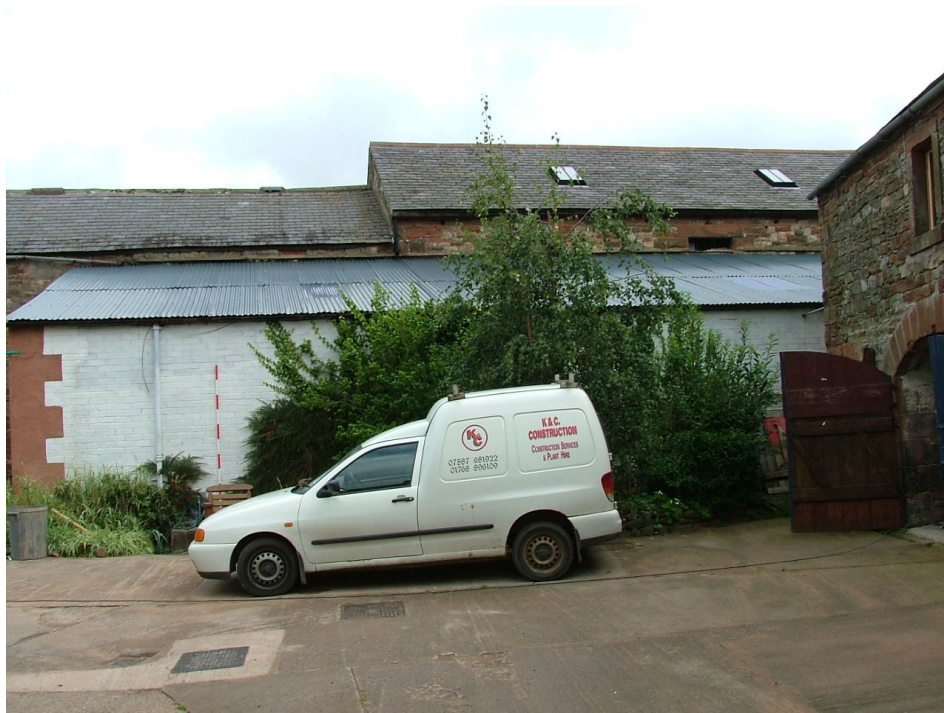
Plate 8 – Southern elevations of Building A, B and E with Building C to right of photograph
