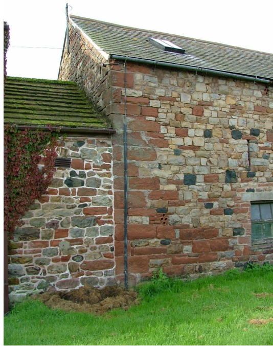
Plate 7 – Eastern end of the north elevation of Building B
