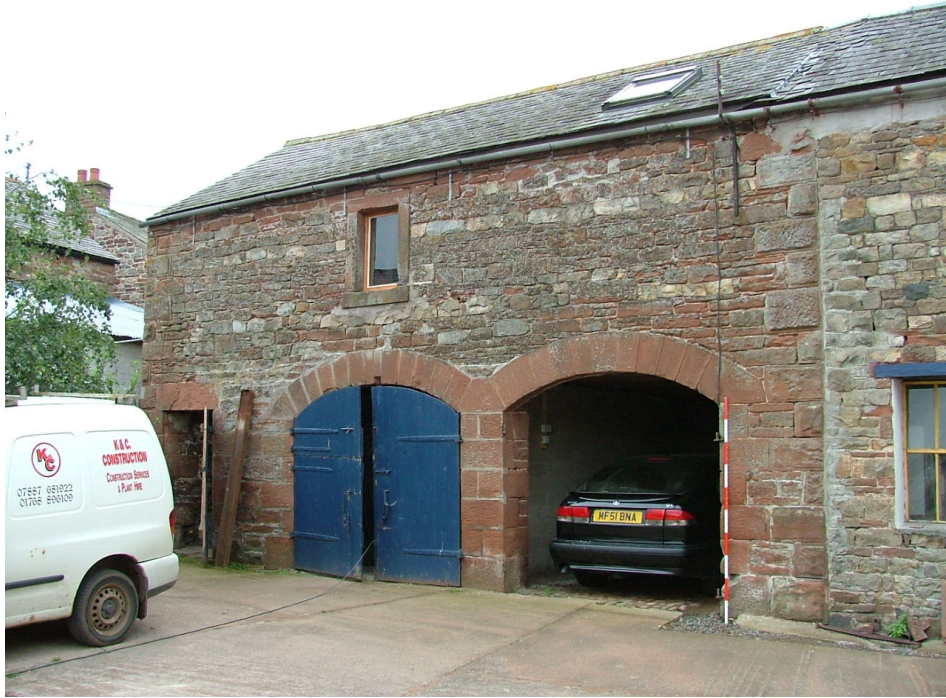
Plate 13 – West facing elevation of Building C
