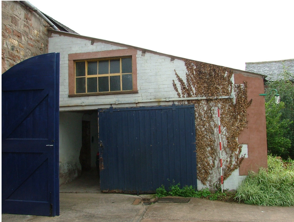
Plate 22 – Western elevation of Building E
