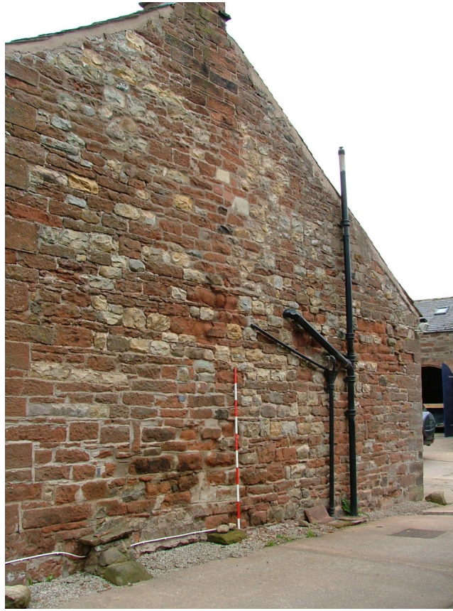
Plate 27 – Eastern elevation of house
