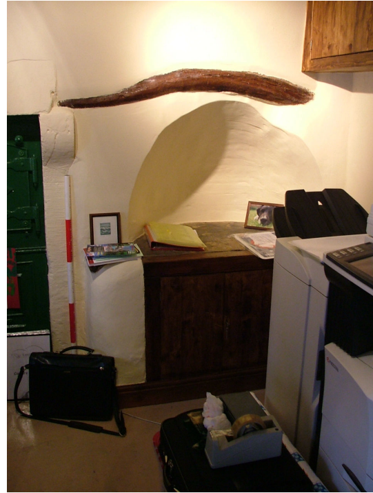
Plate 31 – Set-pot (or wash tub), outshut
