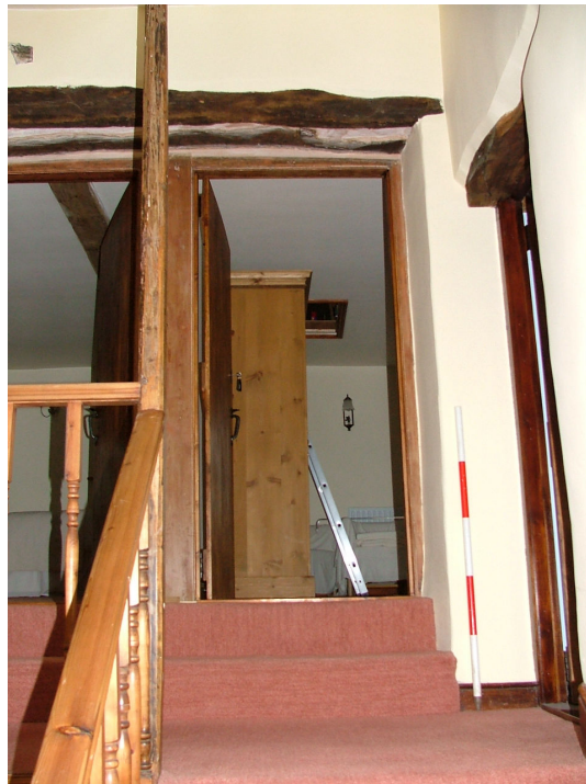
Plate 33 – First floor landing showing steps up to two front bedrooms
