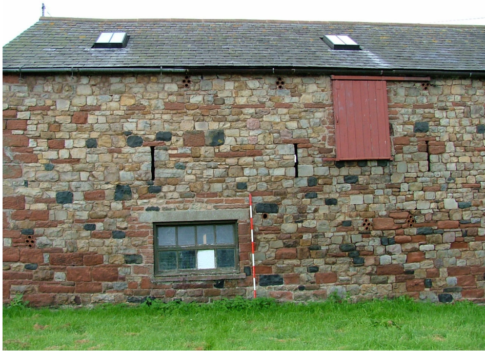
Plate 6 – Northern elevation of Building B
