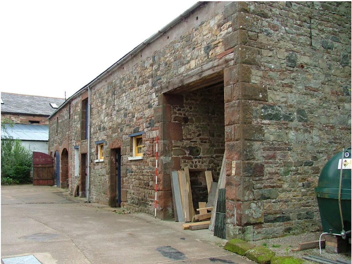
Plate 18 – Building D, western elevation
