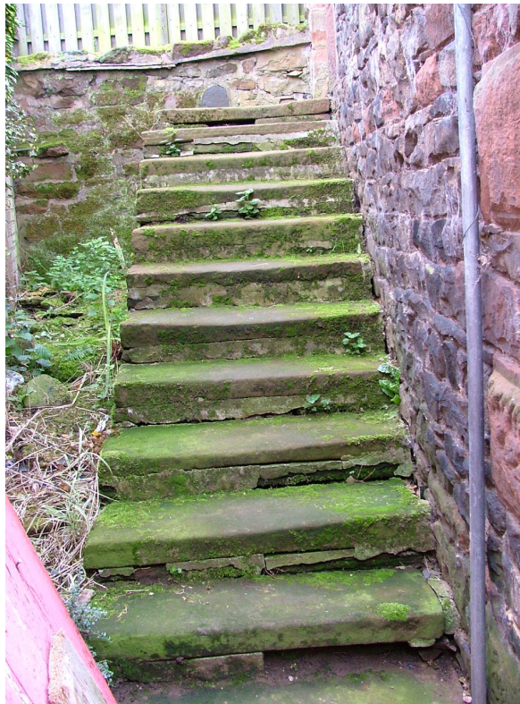
Plate 14 –Stairs, northern gable end of Building C
