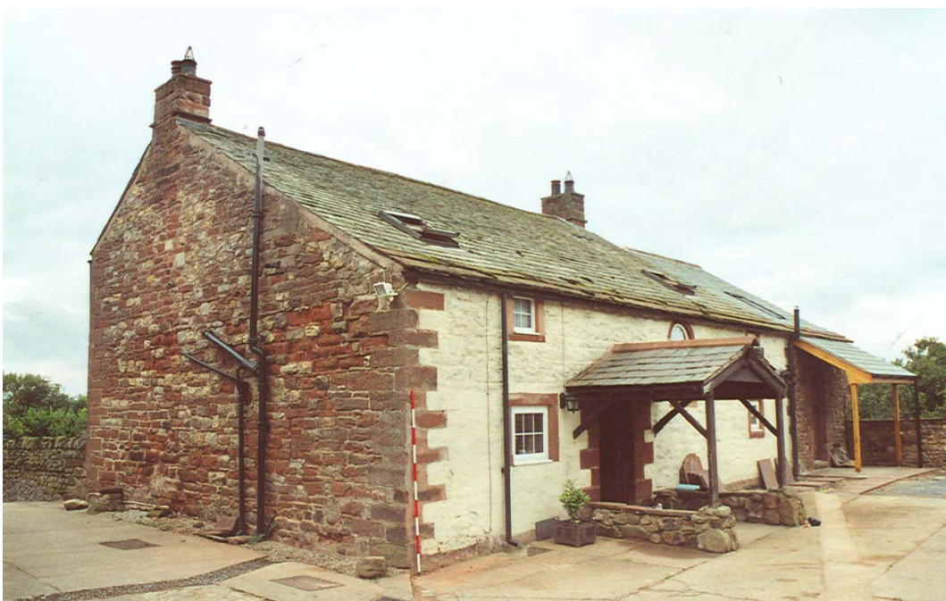
Plate 26 – North and eastern elevations of house
