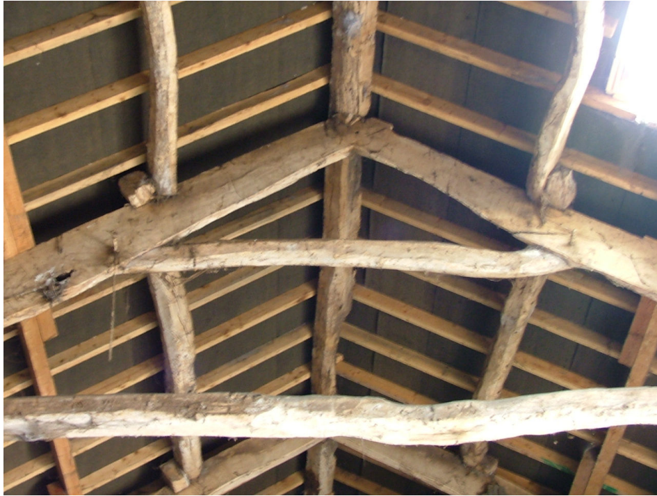
Plate 5 – Detail of roof truss with collar showing wooden pegs
