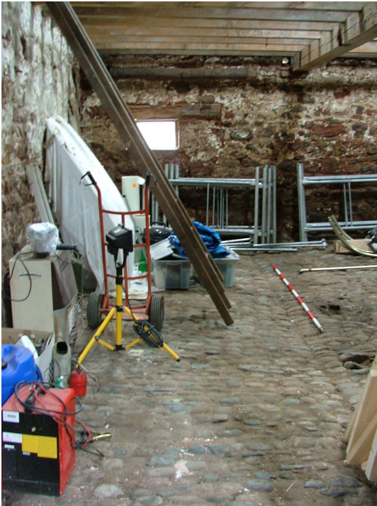
Plate 9 – Interior of store in Building B
