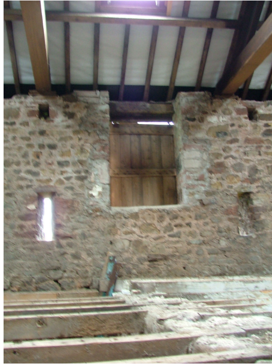
Plate 12 – Northern elevation of Building B, ventilation slits and pitching door
