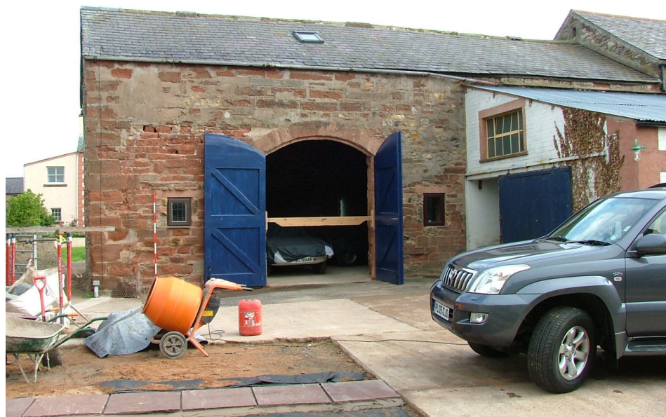
Plate 3 – Southern elevation of Building A
