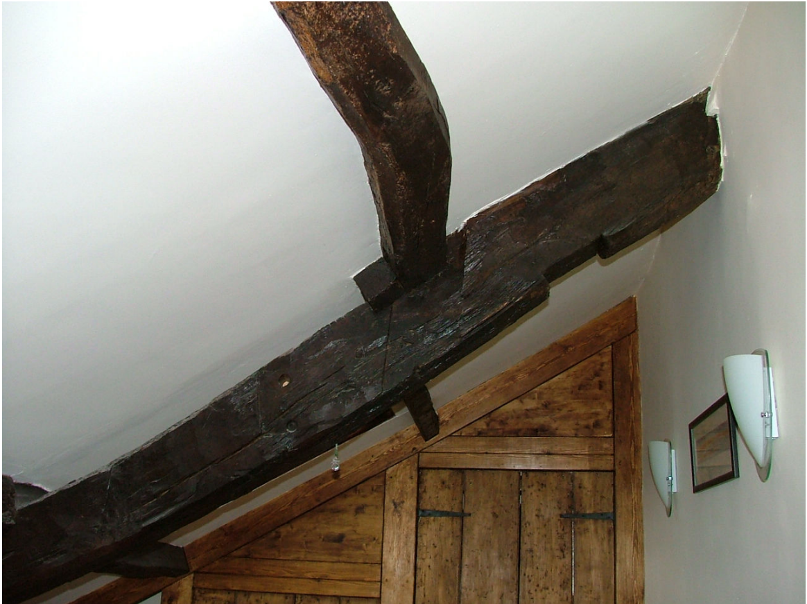
Plate 34 – Roof timbers, back bedroom over former scullery
