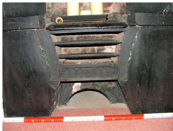
Plate 36 – Detail of grate, first floor bedroom
