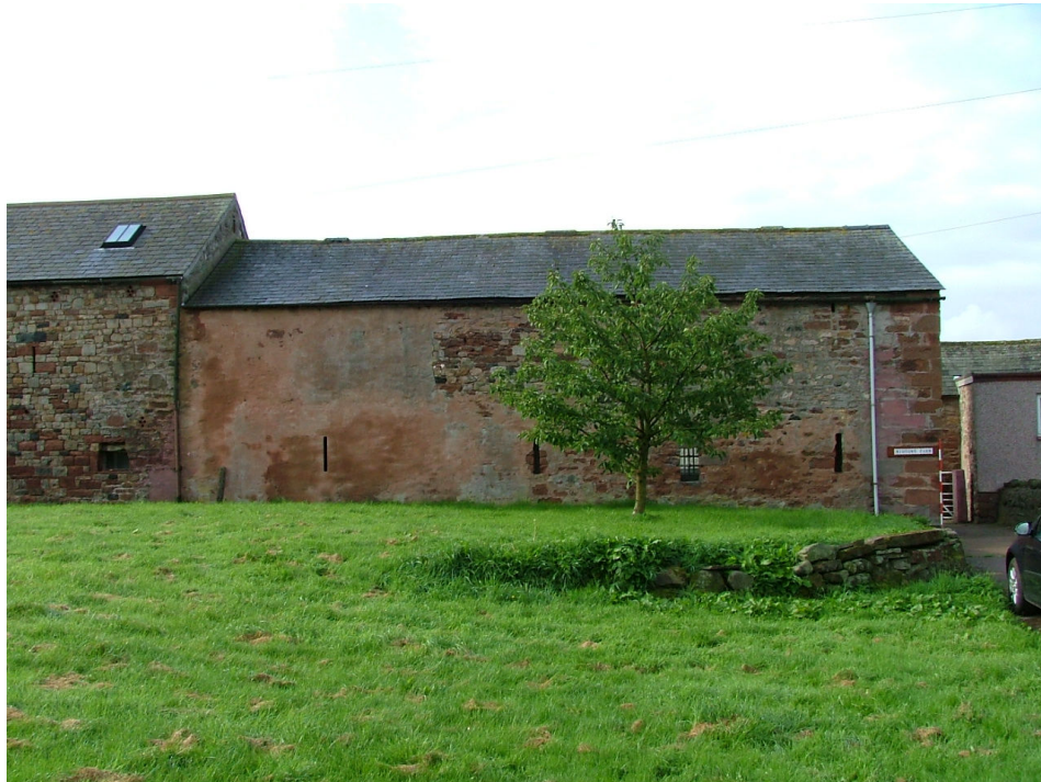
Plate 2 – Northern elevation of Building A
