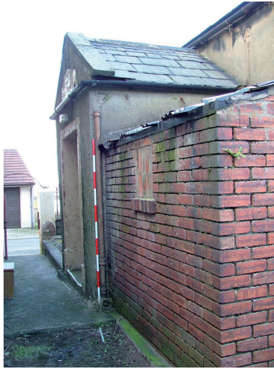
Plate 5 – Brick-built lean-to against eastern side of chapel porch
