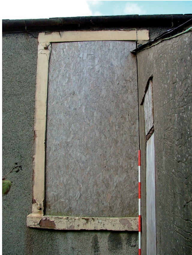
Plate 10 – Eastern elevation, showing wall of extension concealing part of the window jamb
