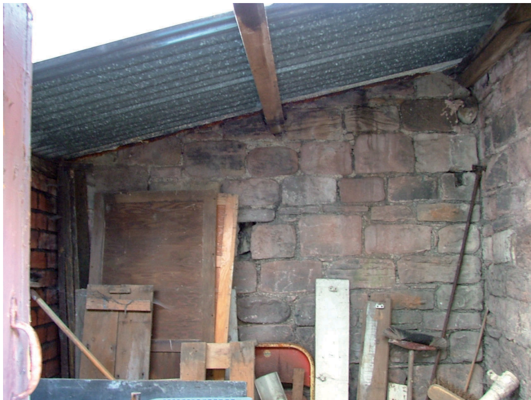
Plate 6 – Interior of brick-built lean-to showing construction material of chapel
