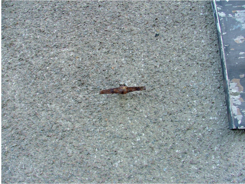
Plate 9 – Western elevation, one of four iron fittings set into the wall
