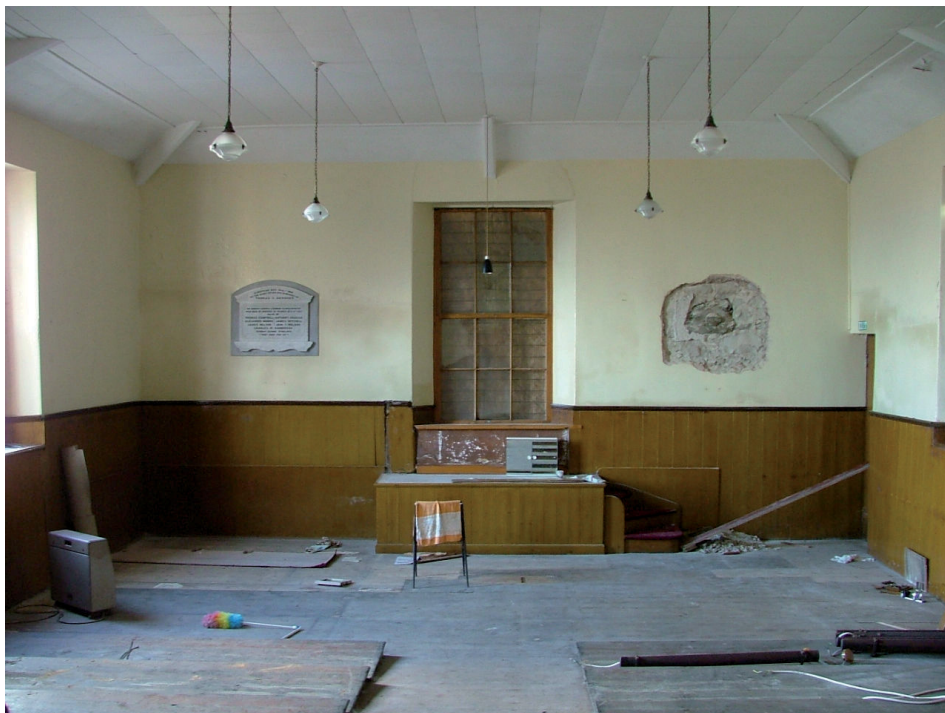
Plate 12 – Interior of chapel showing timber flooring and pulpit at northern end
