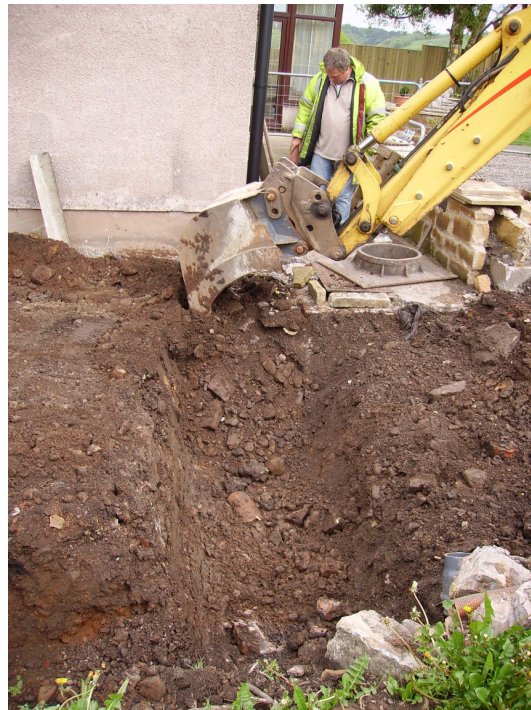
Plate 4: View of eastern section of trench under excavation, facing north
